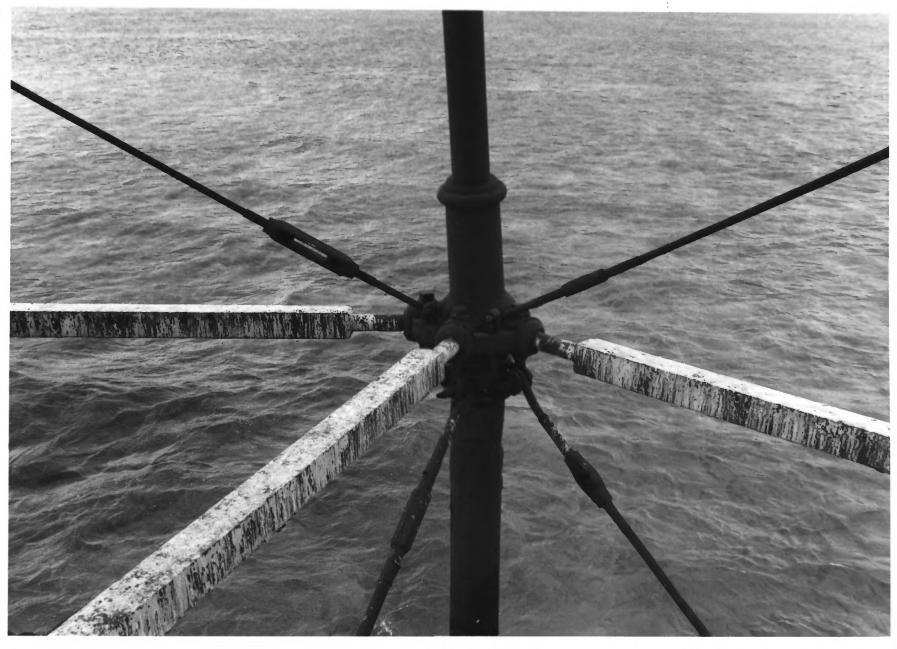
Carysfort Reef Lighthouse 2. Key Largo National Marine Sanctuary 3. Russell Wright 4. 4/82 5. NOAA 6. Peripheral cast iron pile-column with iron box-beams and tie rods 7. Photo # 9
