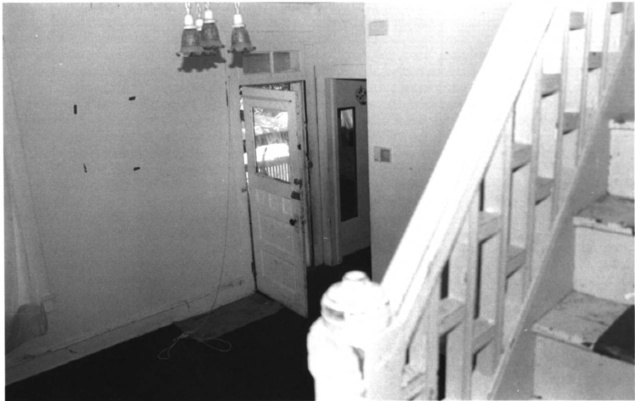
BARNES RENTAL HOUSES HISTORIC DISTRICT ATCHISON CO., KANSAS
