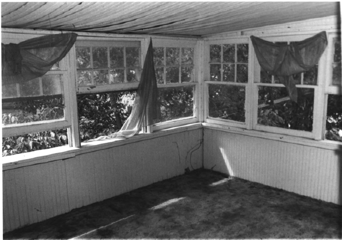
BARNES RENTAL HOUSES HISTORIC DISTRICT ATCHISON CO., KANSAS
