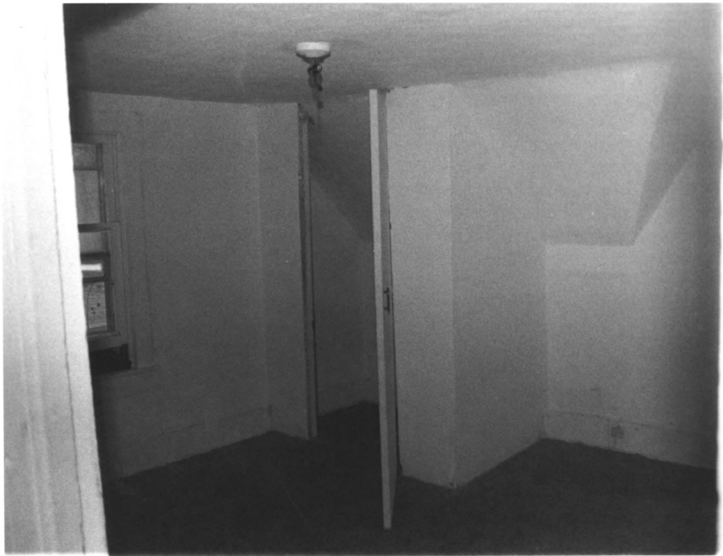
BARNES RENTAL HOUSES HISTORIC DISTRICT ATCHISON Co., KANSAS
