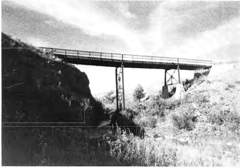
Photo 0005. Shonkin Creek Bridge. South elevation. View to the northeast
