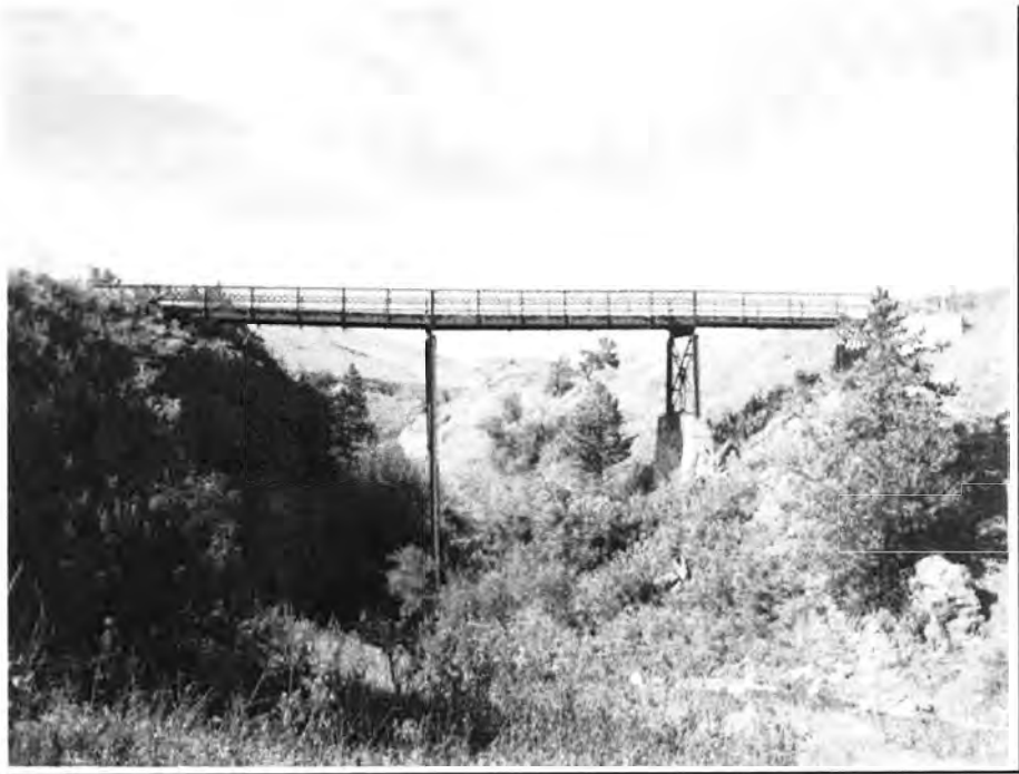
Photo 0004. Shonkin Creek Bridge. South elevation. View to the north.
