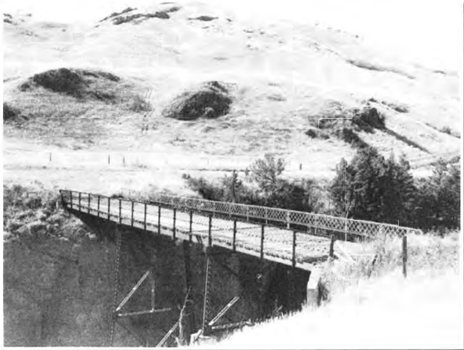
Photo 0003. Shonkin Creek Bridge. North elevation. View to the southeast
