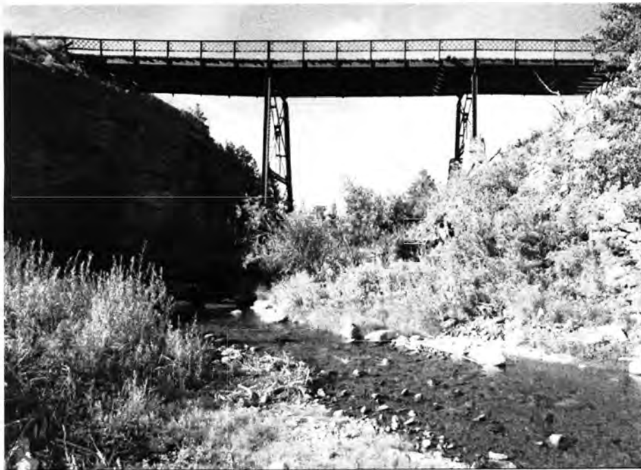
Photo 0002. Shonkin Creek Bridge. South elevation. View to the north
