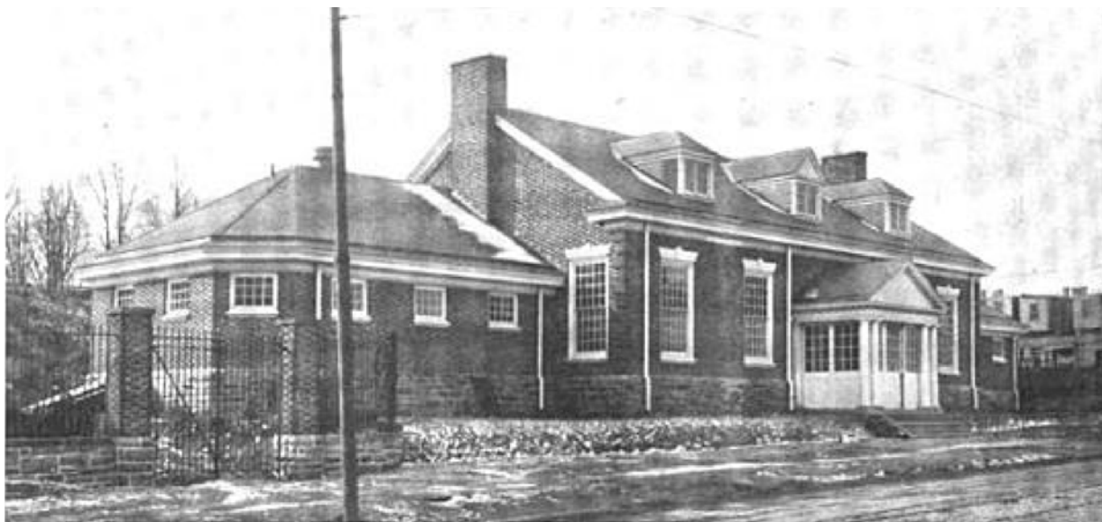
Figure 1. Happy Hollow Recreation Center, shown opening year (1911). Source: Nolan, Thomas. "Some Recent Philadelphia Architecture: Group A - City Buildings." Architectural Record , v. XXIX. New York, NY: The Architectural Record Company, January – June 1911, p. 226.
