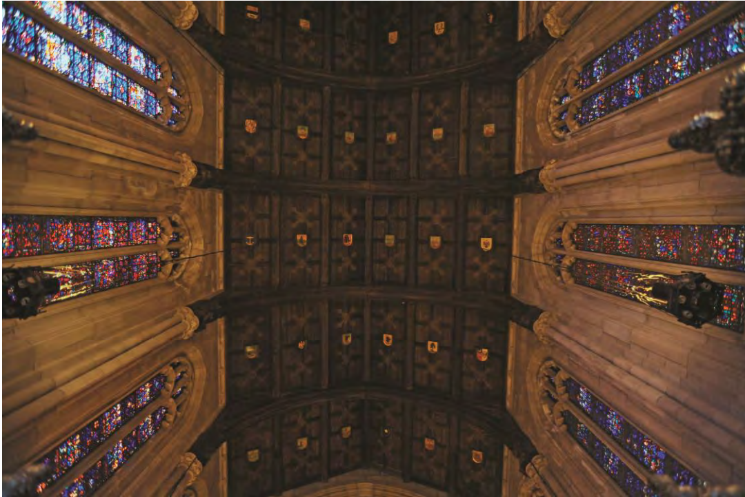
Figure 11: The Roof of the Republic, the wood ceiling of the Sanctuary, contains the seals for each state. Carved angels support the roof trusses over the nave, while carved pelicans support those over the choir area. (photo from A Guide to the History, Art & Architecture of the Washington Memorial Chapel )
