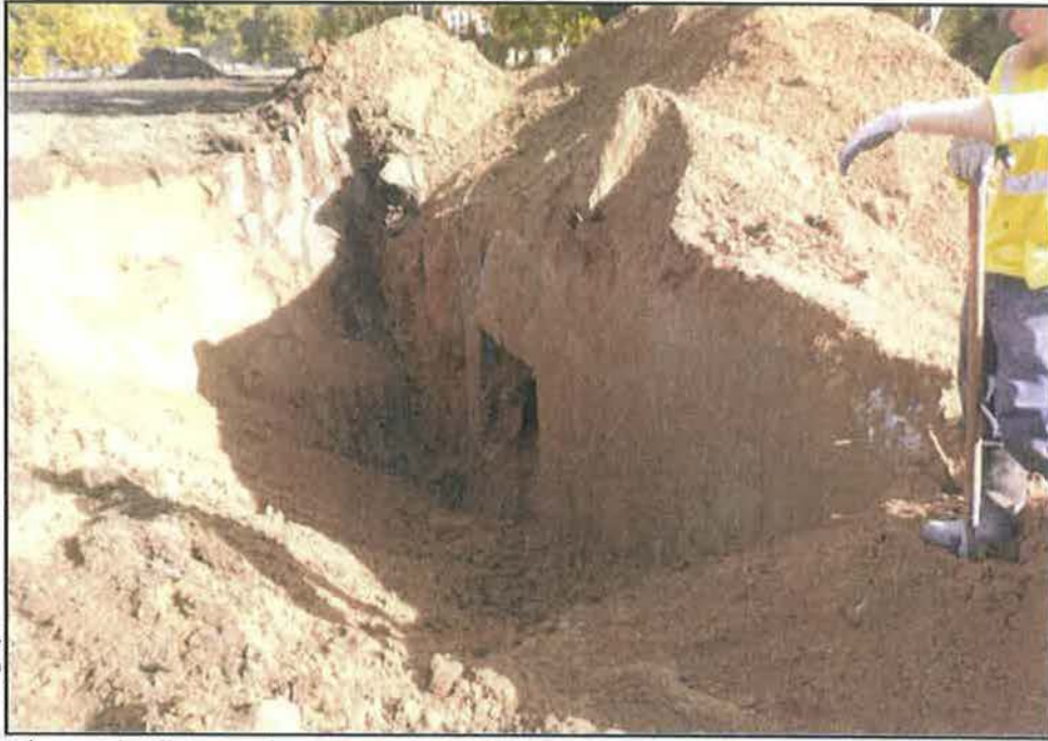
Figure 6. Connecting Tunnel, Between Winding Lane and Maintenance Building, View North
