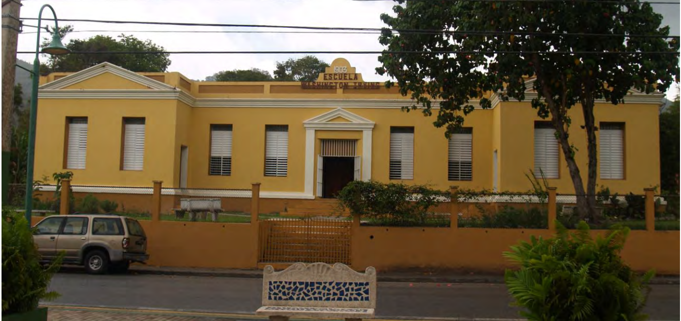
Figure 3. Washington Irving Graded School's main facade, 2014, looking east. (Source: Juan Llanes Santos)
