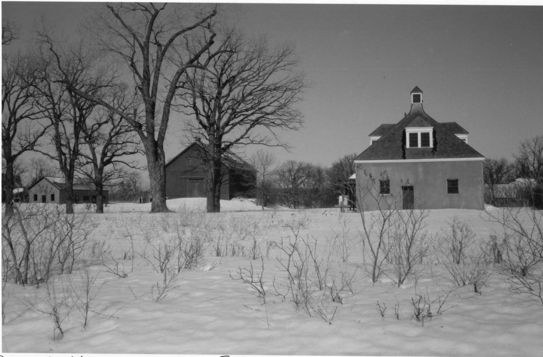
Dairy Building, North Oaks Farm Red Barn Road at Hill Farm Circle Ramsey Co., Mn 013151-1
