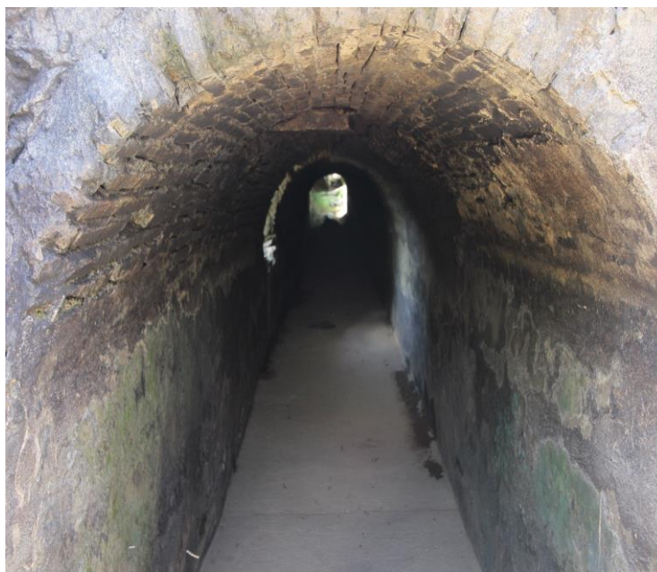
Figure 12. Left, detail of the 1868' schematic of the vaulted section on Cortadas's canal. Right, for comparison purposes, photograph of an existing vaulted section of an irrigation canal built by the joint effort of three haciendas (Florida, Santa Isabel and Destino) during the 1880's in Santa Isabel. (Juan Llanes Santos, photographer, 2016)
