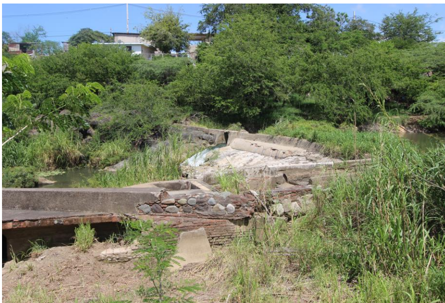
Figure 3. Partial view of a late 1800s dam, water intake and supply canal, built on the Coamo River to provide water for three haciendas: Florida , Santa Isabel and El Destino . (Photographer: Juan Llanes Santos, 2016)
