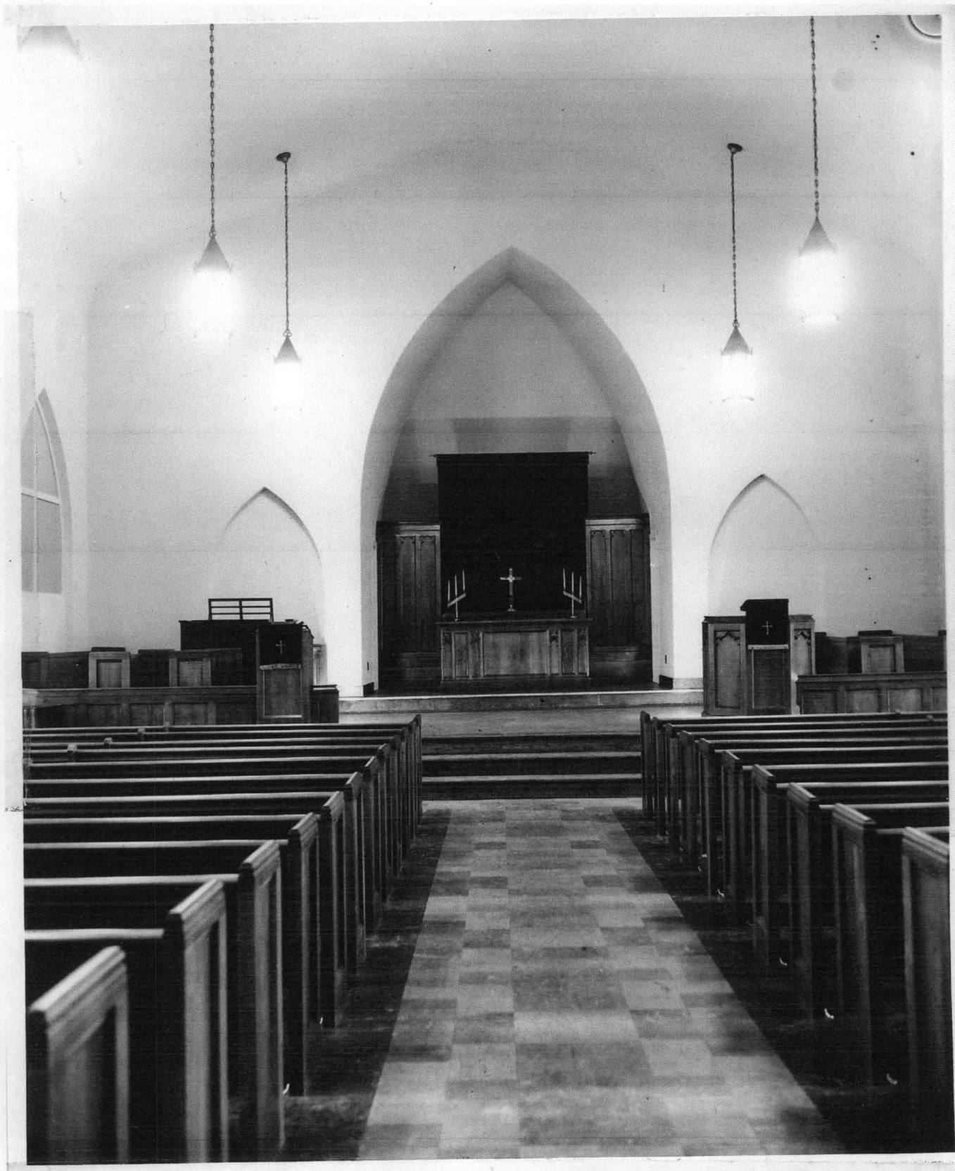
Figure 24. Interior of Tabor Congregational Church around 1949 (Bound scrapbook, Congregational Church).
