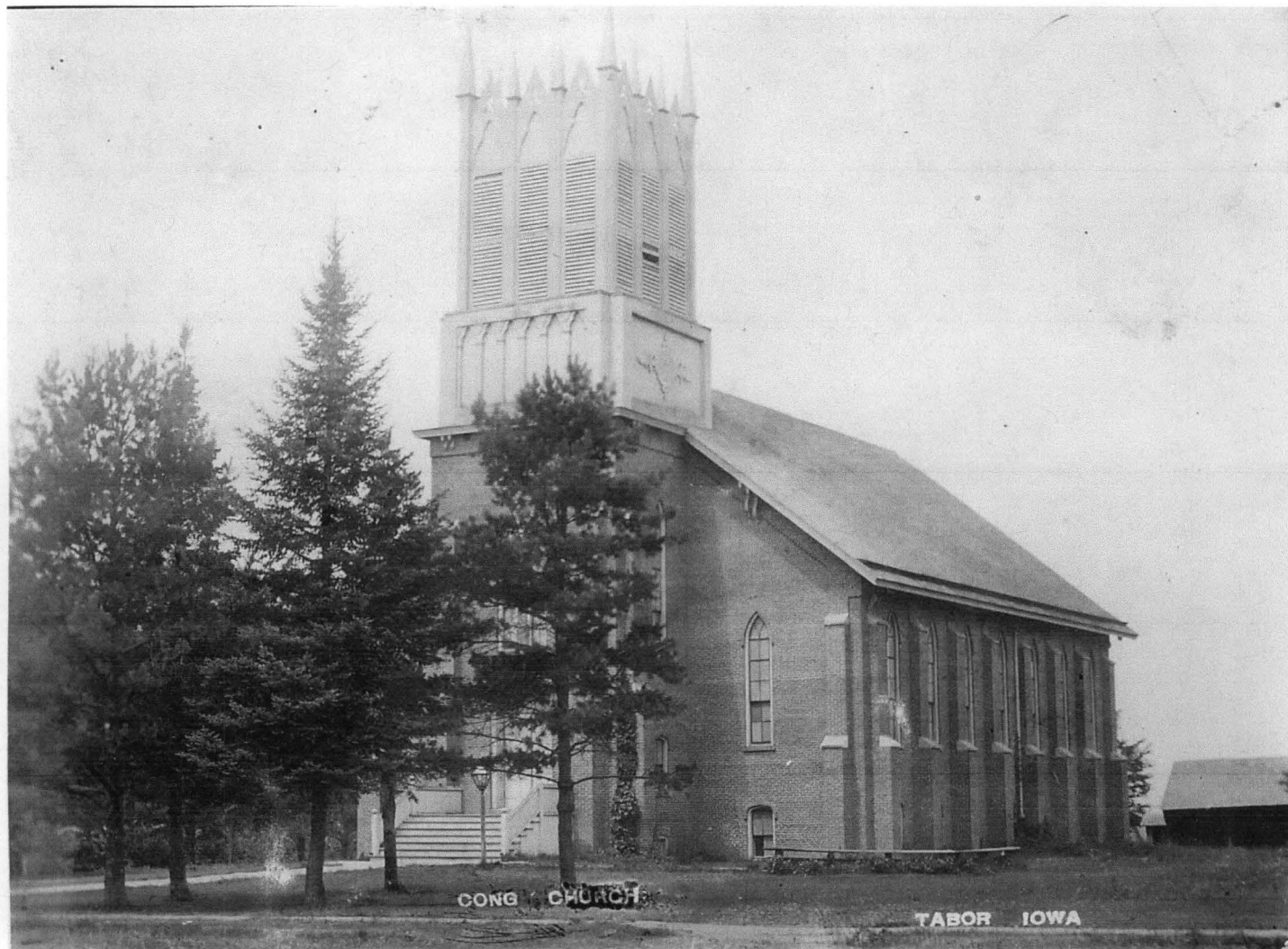
Figure 17. Tabor Congregational Church after 1907 repairs (Congregational Church files).
