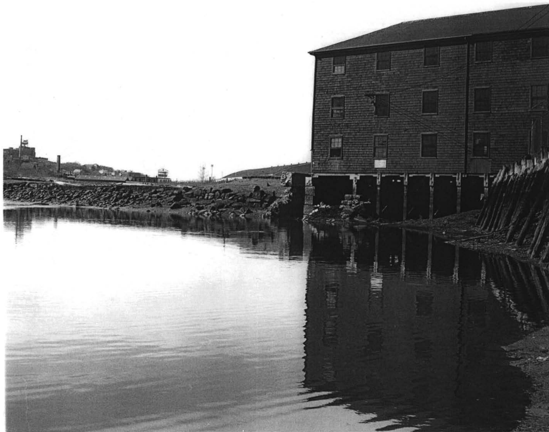
2. Southeast facade and dam (Photograph: Dr. Peveril Meigs, 1972)
