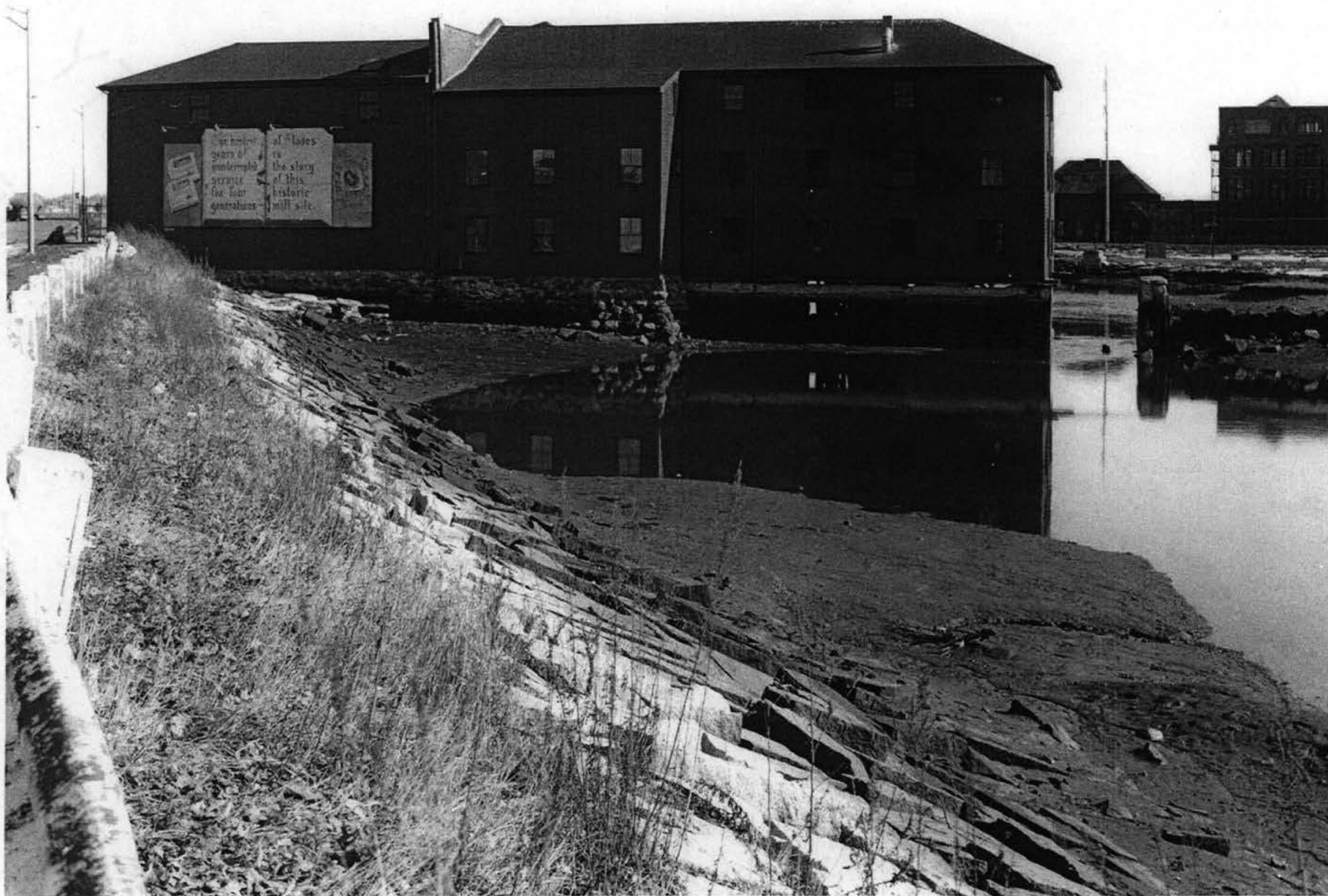
1. Northwest Facade showing mill pond (Photograph: Dr. Peveril Meigs, 1972)
