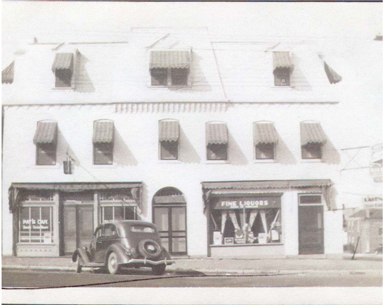
Figure 13. Late-1930s photograph of south façade
