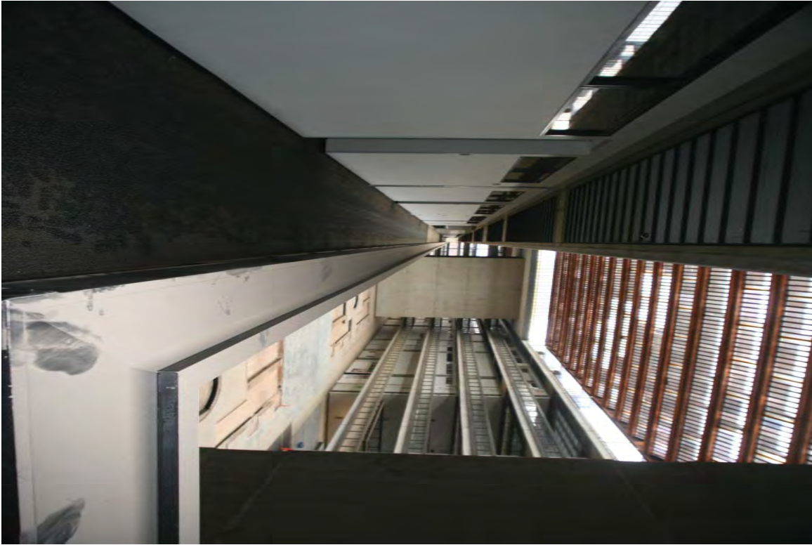
19. Fourth floor of Bell Laboratories-Holmdel, looking east at office area
