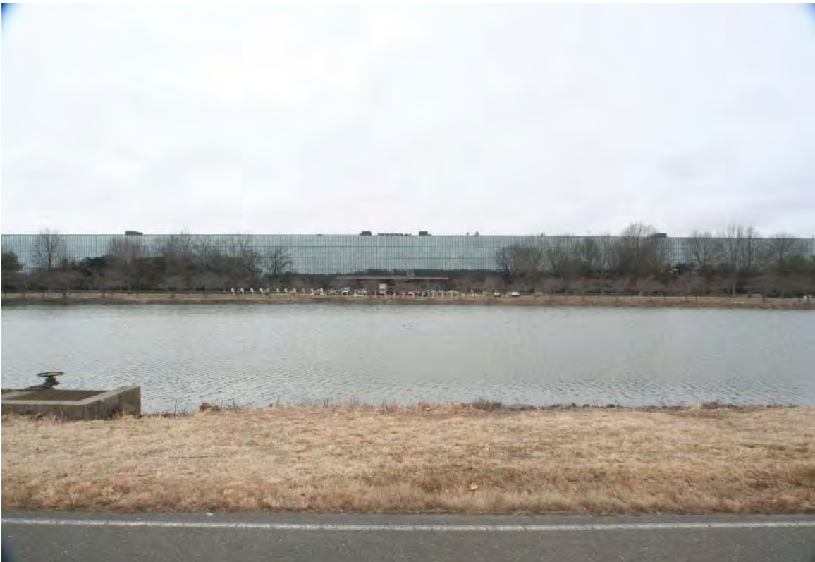
2. North elevation of Bell Laboratories-Holmdel, looking southwest
