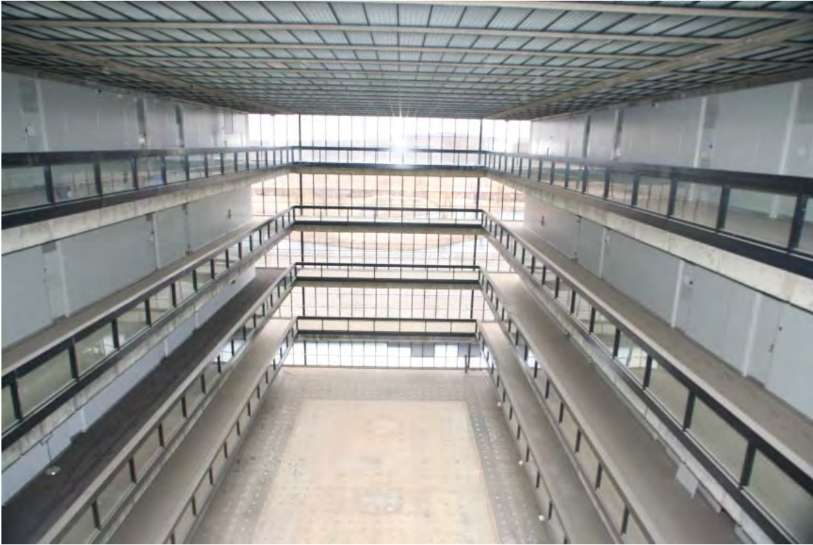
25. Sixth floor of Bell Laboratories-Holmdel, looking southeast
