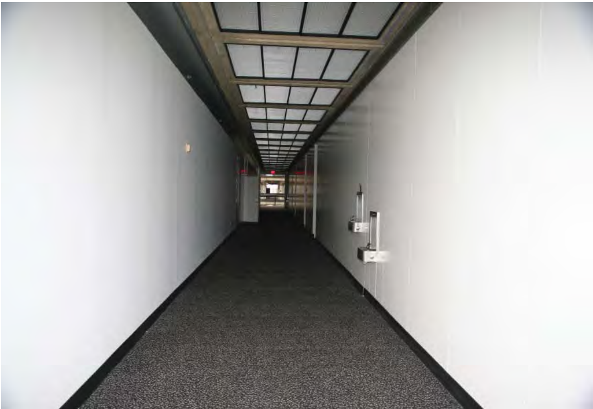
18. Fourth floor of Bell Laboratories-Holmdel, looking southeast at corridor
