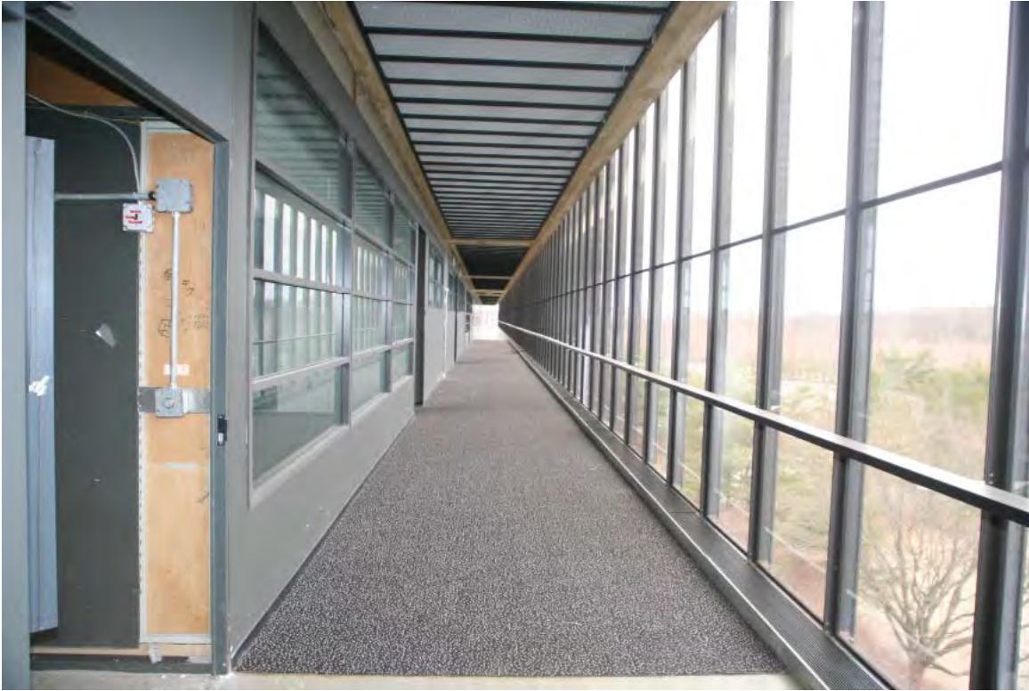
21. Fifth floor of Bell Laboratories-Holmdel, looking northeast at corridor
