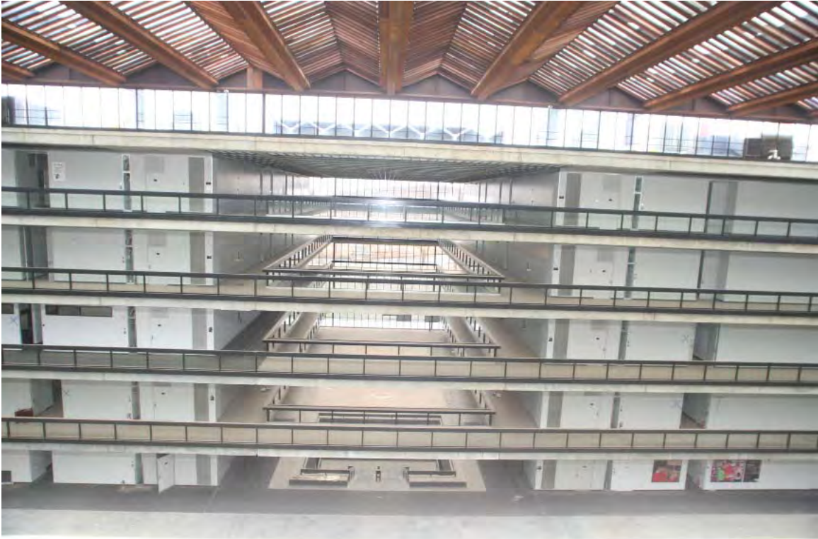
23. Sixth floor of Bell Laboratories-Holmdel, looking southeast
