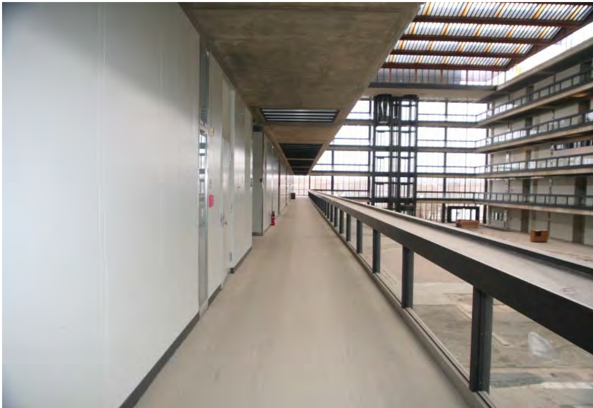
16. Third floor of Bell Laboratories-Holmdel, looking northeast at corridor
