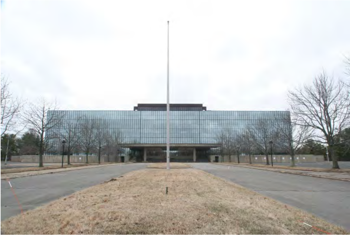
3. West elevation of Bell Laboratories-Holmdel, looking southeast
