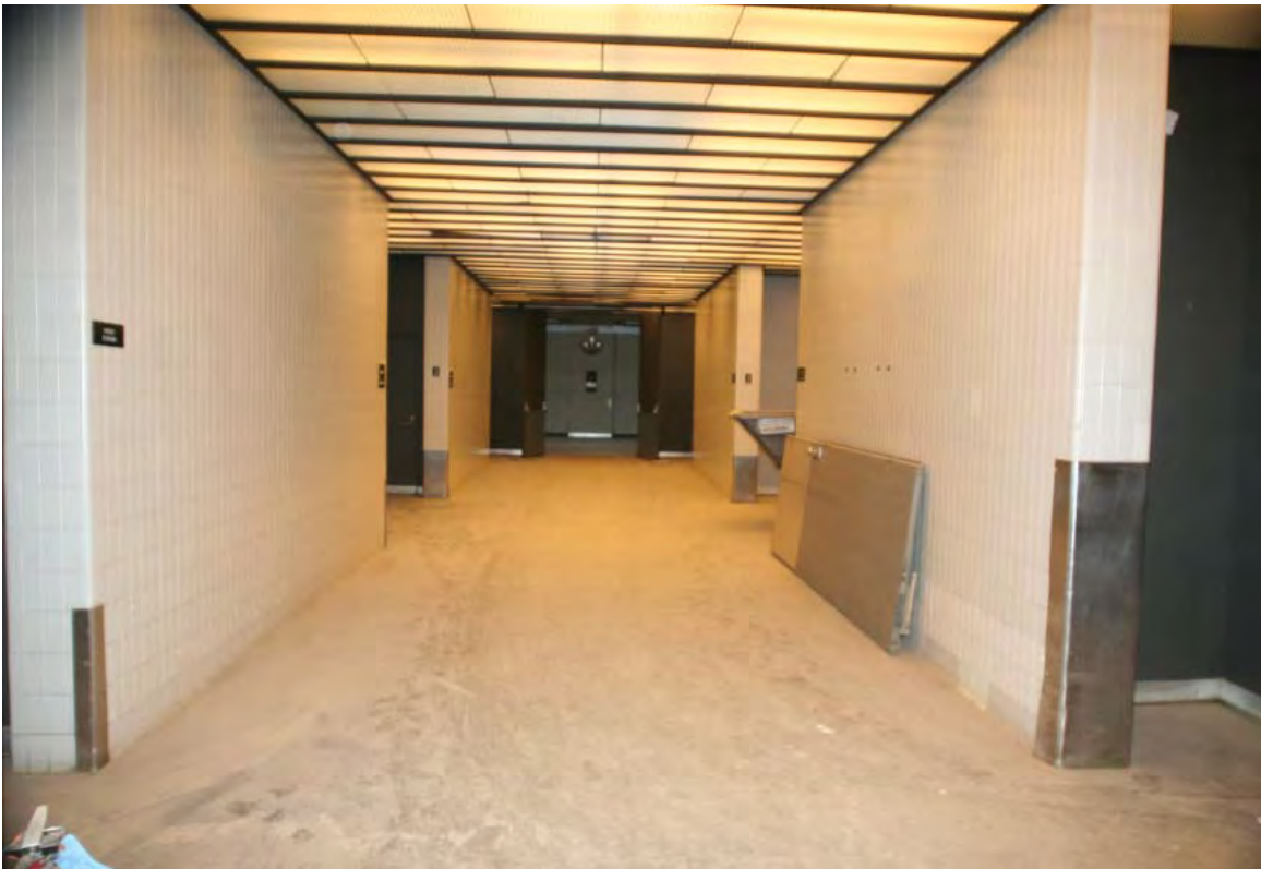
12. Second floor of Bell Laboratories-Holmdel, looking southeast at stair/elevator tower
