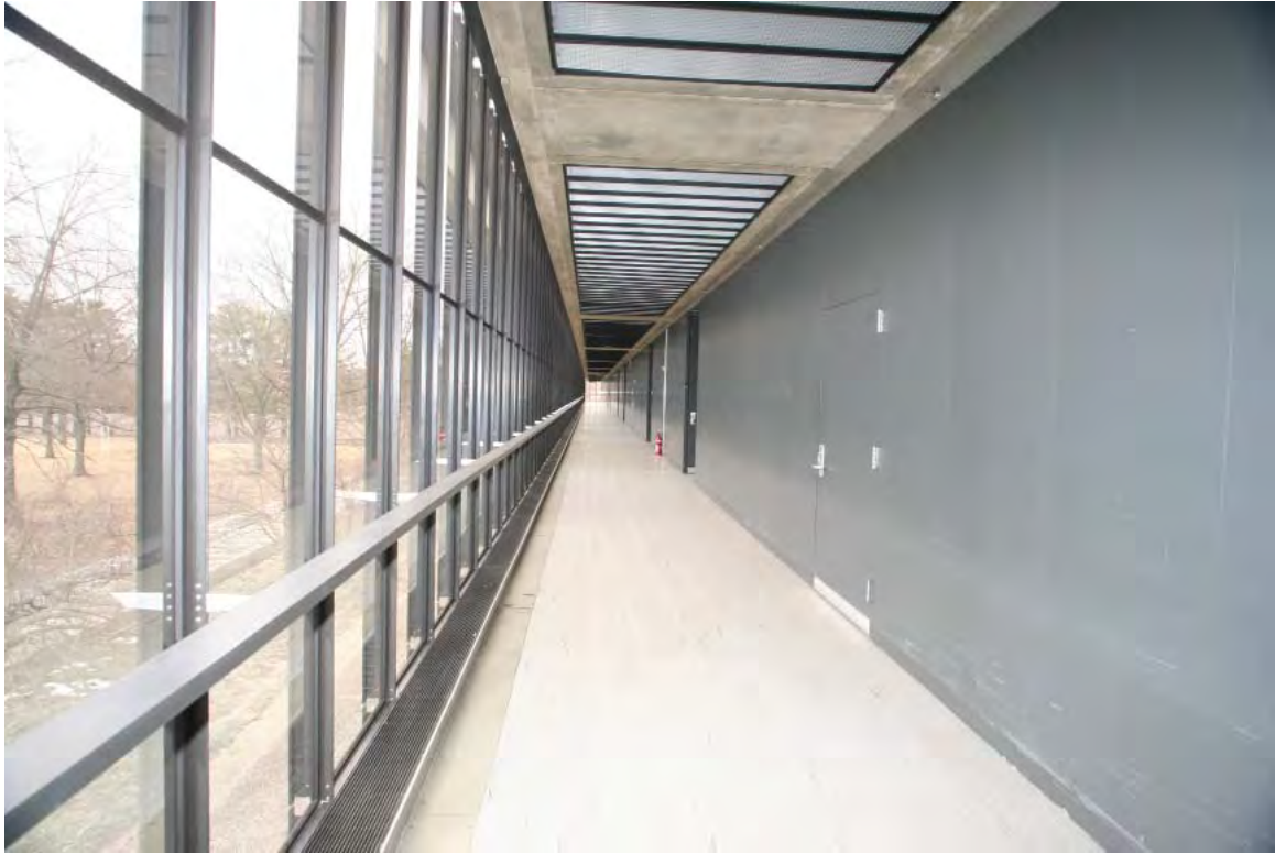
15. Third floor of Bell Laboratories-Holmdel, looking northeast at corridor
