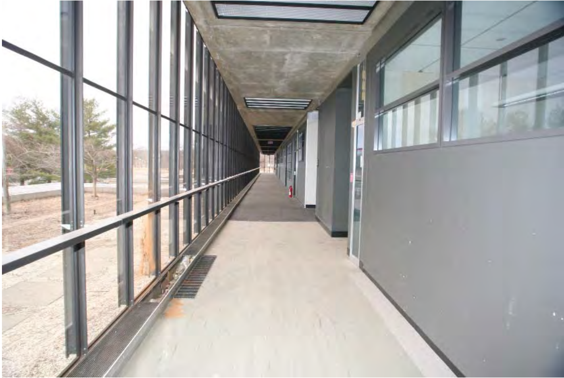
13. Second floor of Bell Laboratories-Holmdel, looking southwest at corridor
