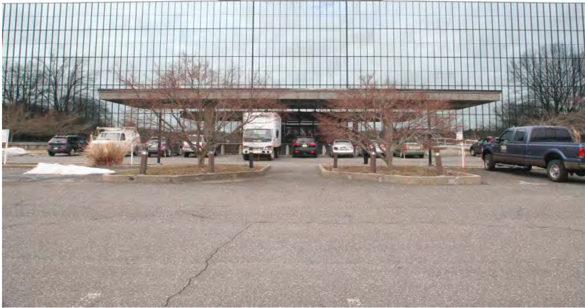
7. North elevation of Bell Laboratories-Holmdel, looking southwest at entrance
