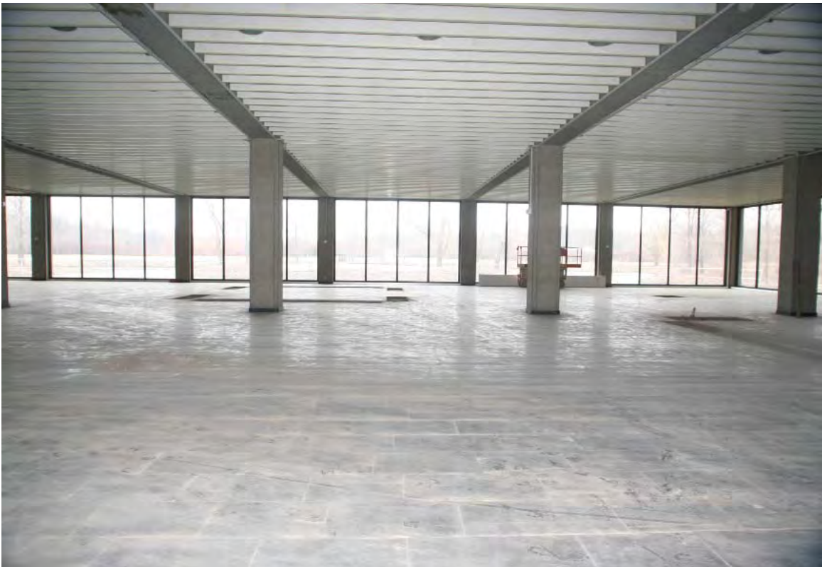
28. First floor of Bell Laboratories-Holmdel, looking southeast at cafeteria
