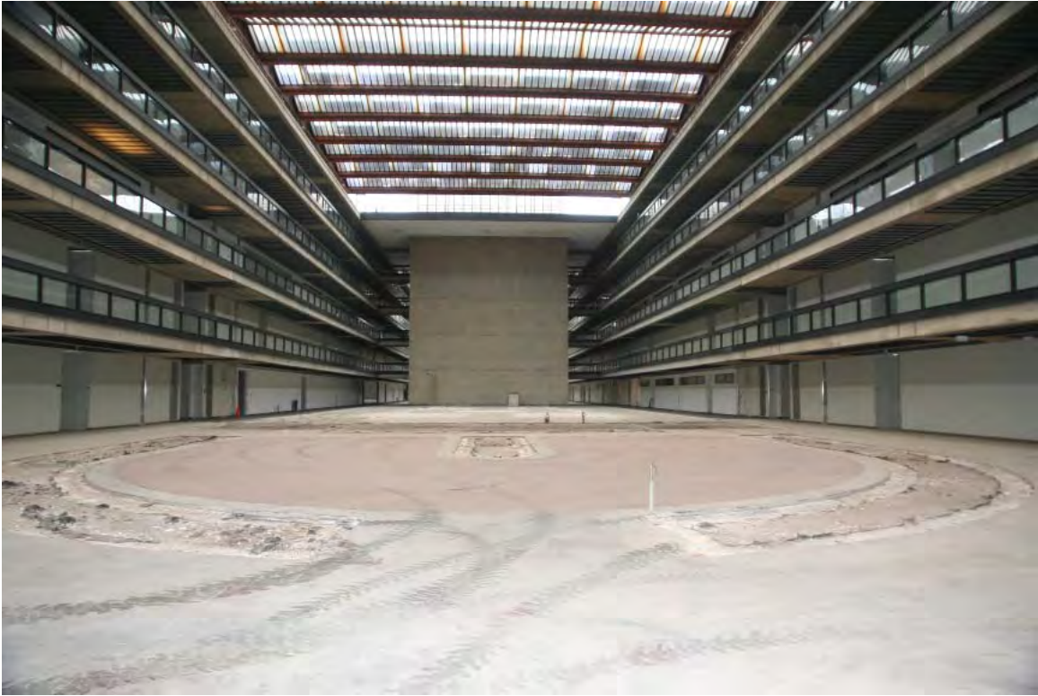
11. Second floor of Bell Laboratories-Holmdel, looking west at atrium
