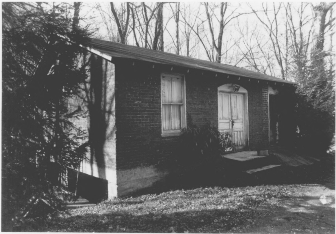
Walland Power Plant, Blount Co., TN, Photo 1 of 3
