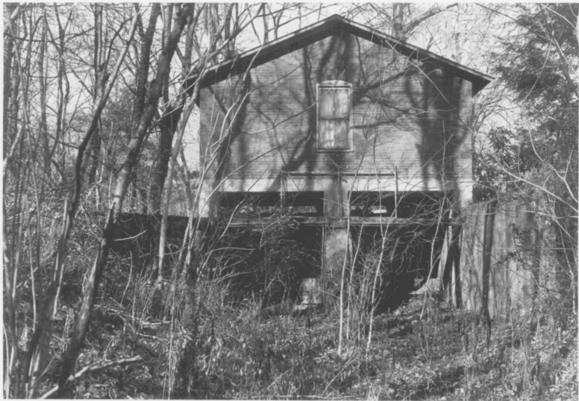
Walland Power Plant, Blount Co., TN, Photo 3 of 3
