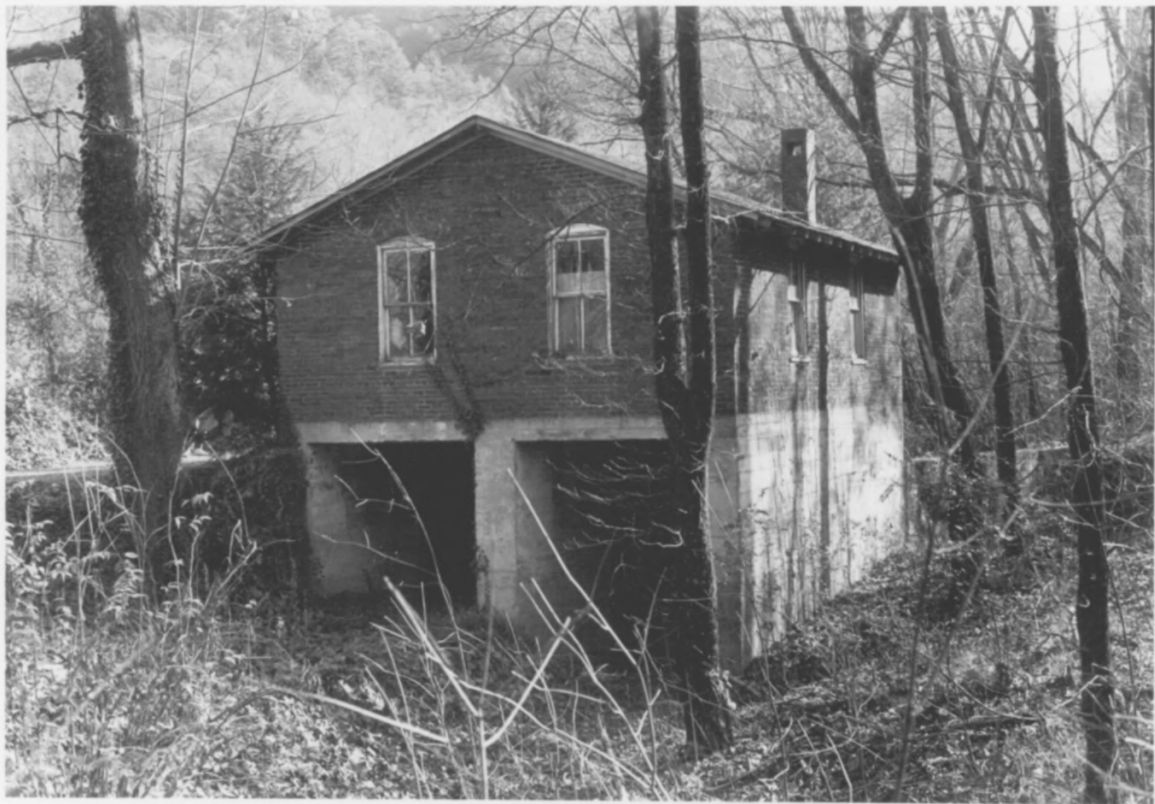
Walland Power Plant, Blount Co., TN, Photo 2 of 3
