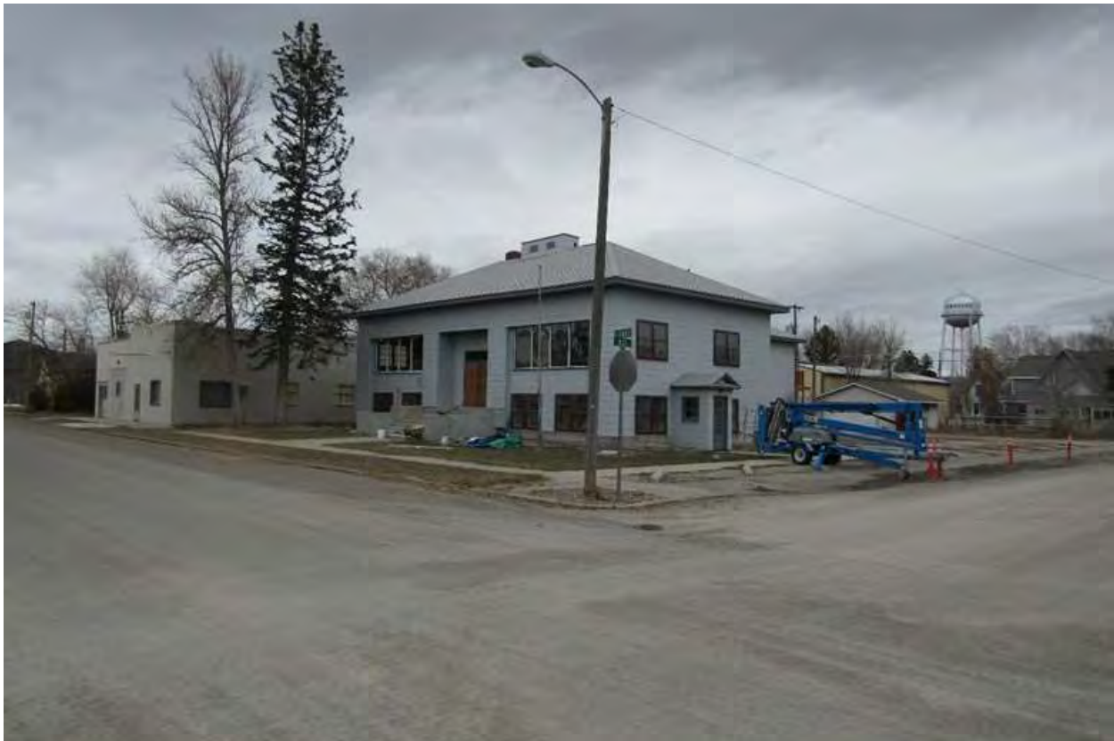
Valley Masonic Lodge No. 21, view to northeast. MT_BroadwaterCounty_ValleyMasonicLodgeNo.21_0001
