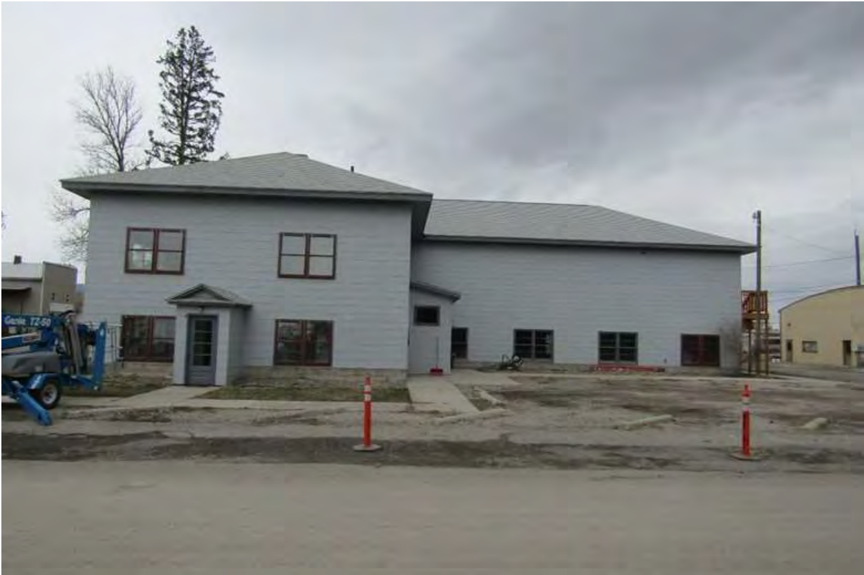
Valley Masonic Lodge No. 21, view to north. MT_BroadwaterCounty_ValleyMasonicLodgeNo21_0004.
