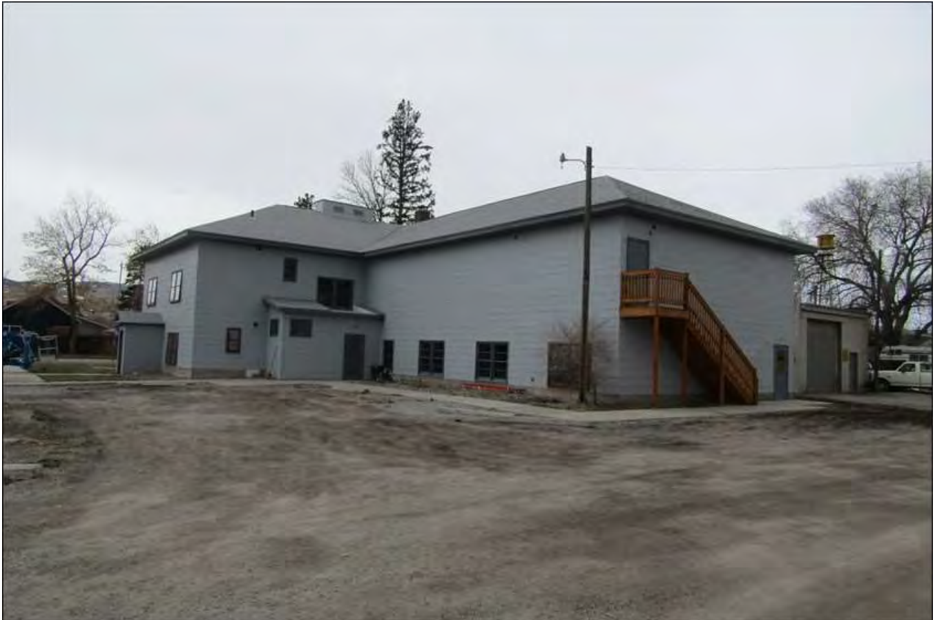
Valley Masonic Lodge No. 21, view to northeast. MT_BroadwaterCounty_ValleyMasonicLodgeNo21_0006.
