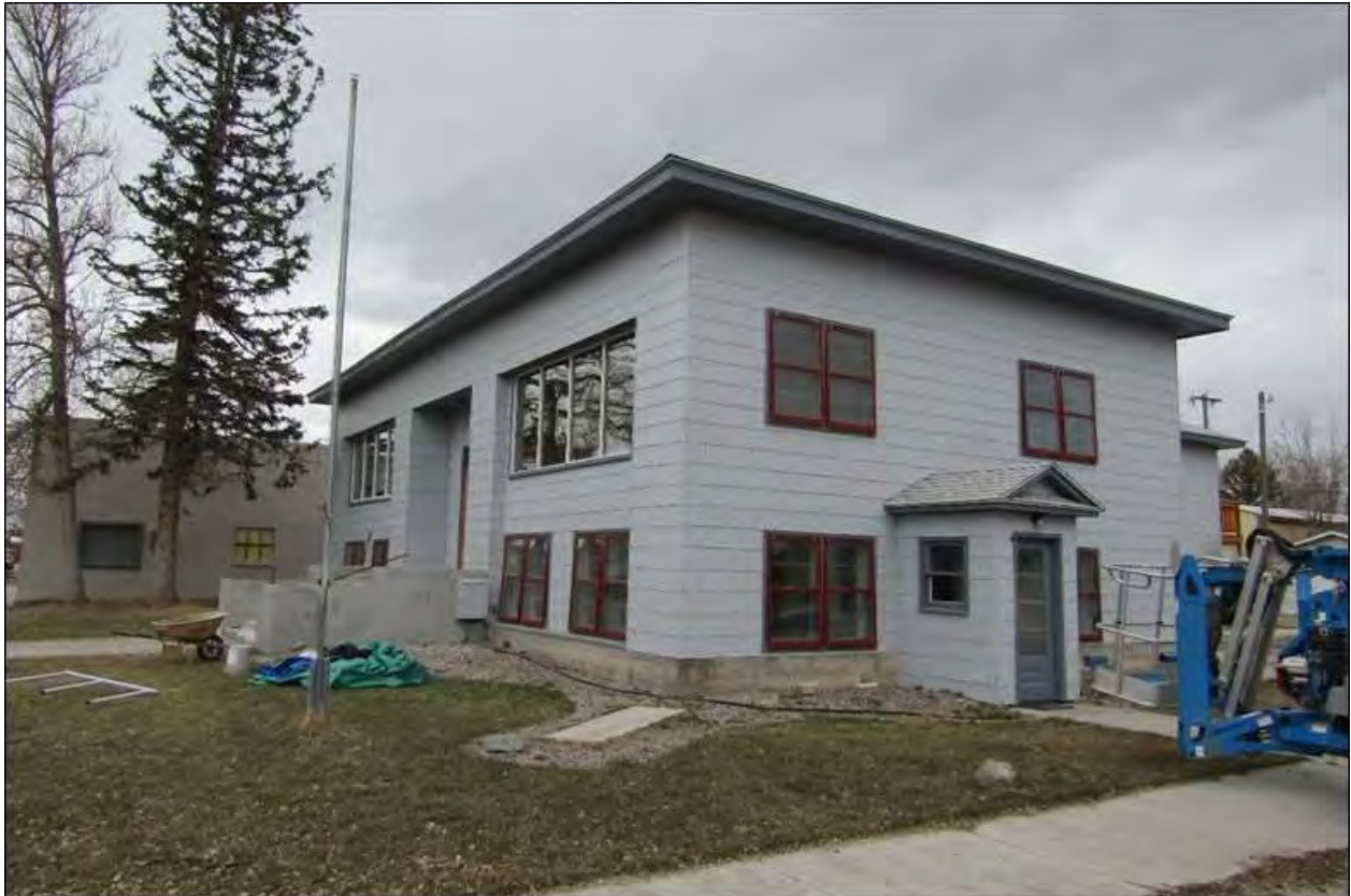
Valley Masonic Lodge No. 21, view to northeast. MT_BroadwaterCounty_ValleyMasonicLodgeNo21_0003.
