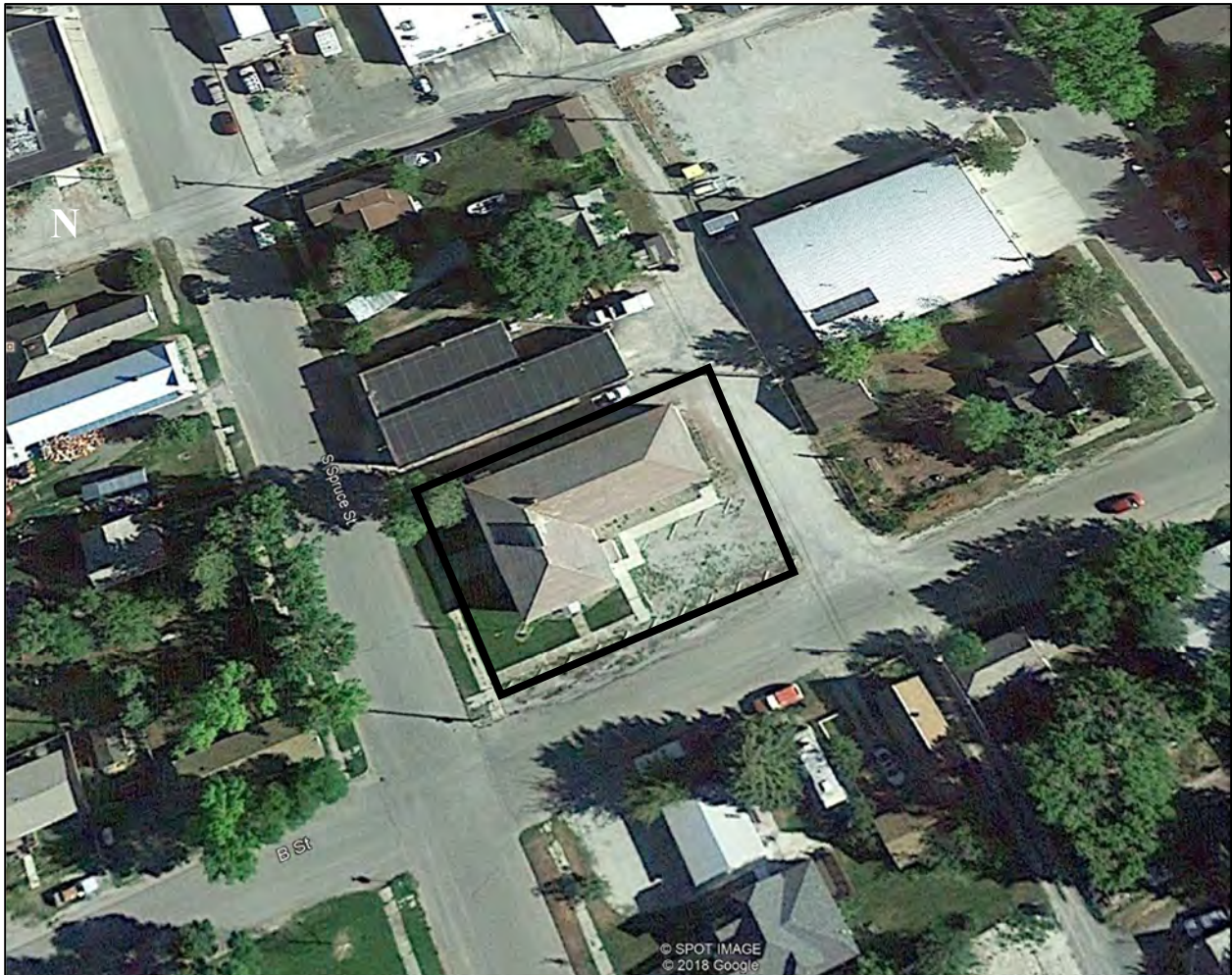
Aerial view of the Valley Masonic Lodge No. 21 (center of image, outlined in black box), Townsend, MT
