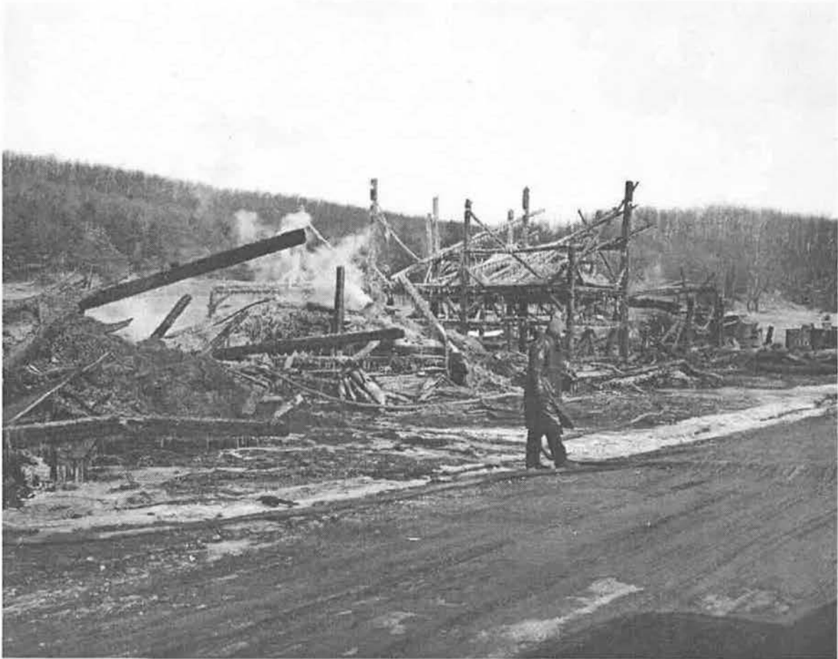
Figure 4. Company Farm Barn Fire (1959)
