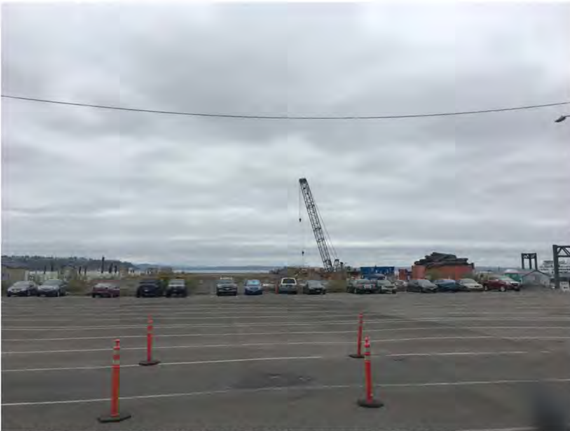
1 of 3: Ballast Island Overview View from Main to west with Pier 48.
