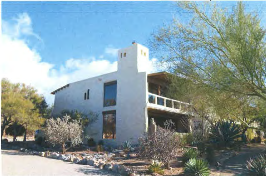
Photo 5. Overview of 1964 complex, south side, Catalina Foothills Estates Apartments, view facing northeast (2014).
