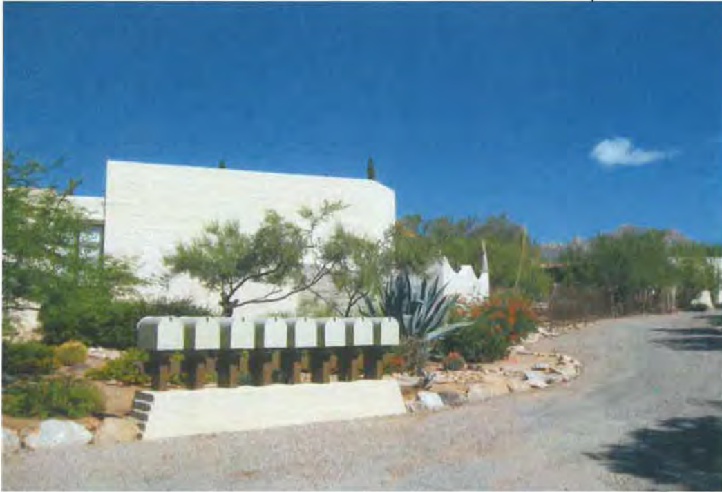
Photo 15. Overview of original communal mailboxes, Catalina Foothills Estates Apartments, view facing southwest (2014).
