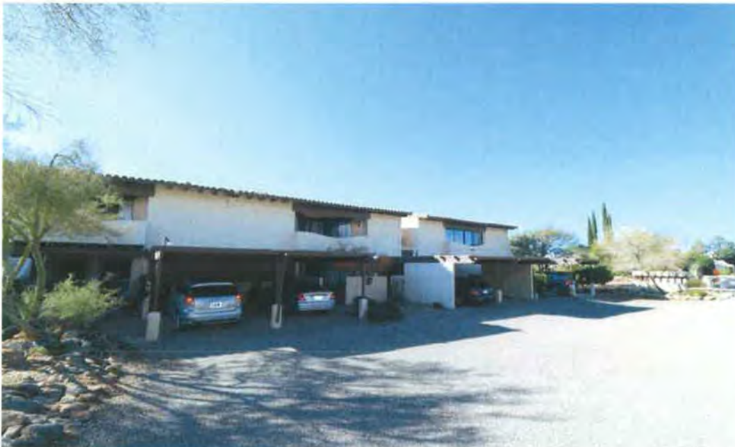
Photo 4. Overview of 1964 complex, north side, Catalina Foothills Estates Apartments, view facing southwest (2014).
