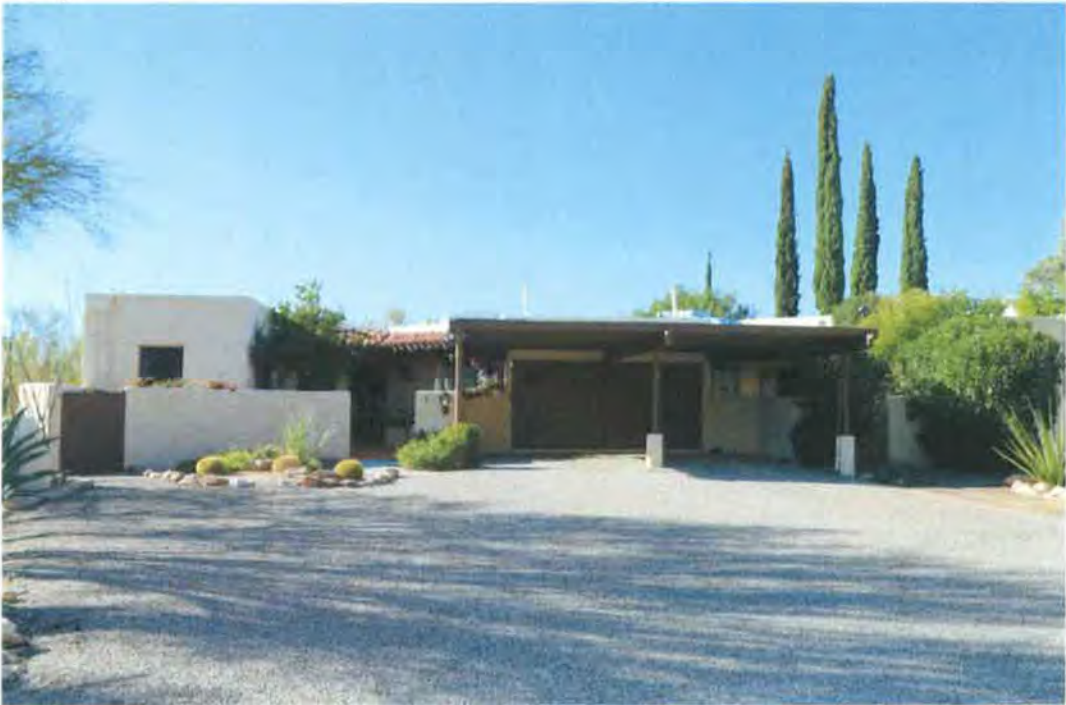
Photo 2. Overview of a 1963 unit, north side, Catalina Foothills Estates Apartments, view facing south (2014).
