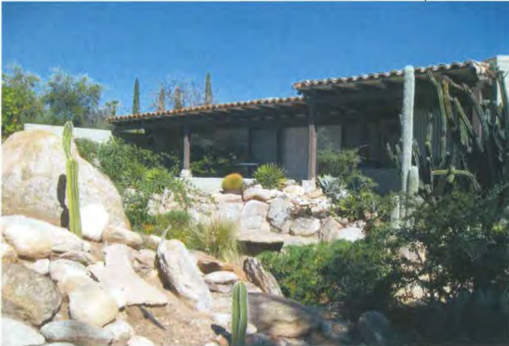
Photo 11. South façade of Caretaker's Residence with rock-lined water feature in foreground, Catalina Foothills Estates Apartments, view facing northwest (2014).
