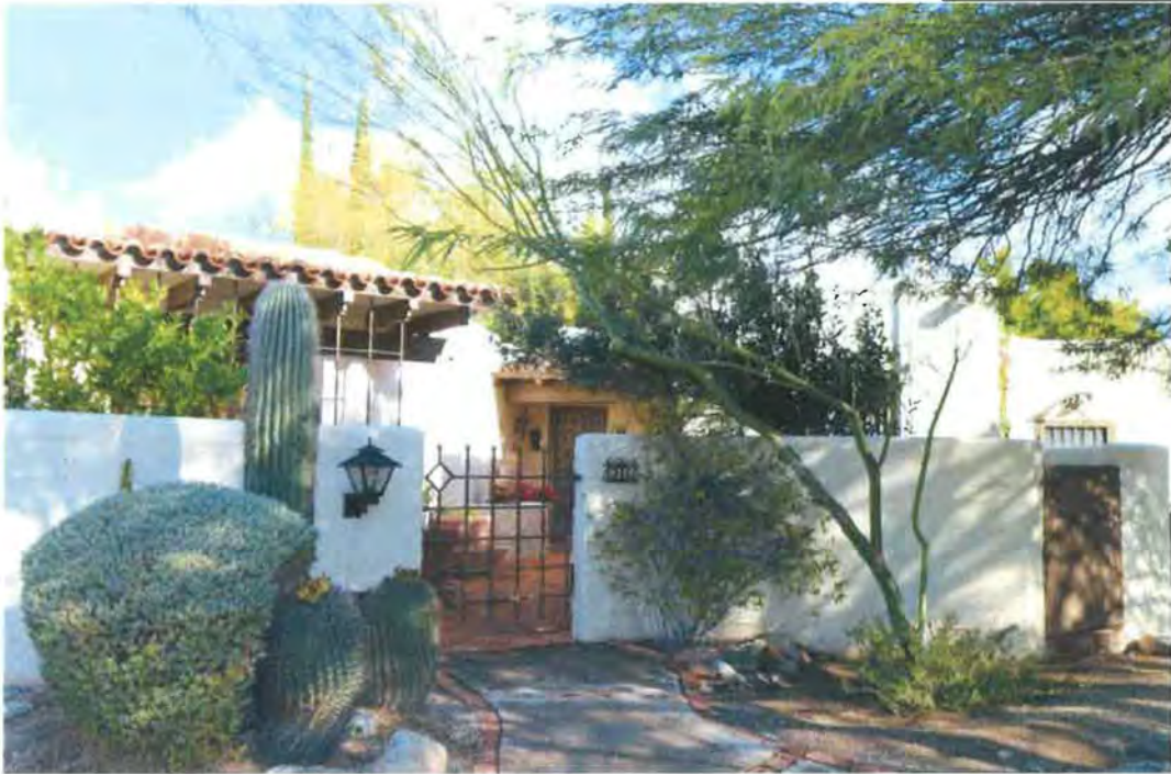
Photo 1. Detail of 1963 façade, south side, Catalina Foothills Estates Apartments, view facing northeast (2014).
