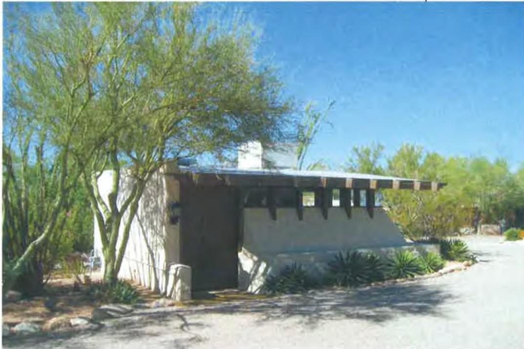
Photo 13. Overview of laundry building, Catalina Foothills Estates Apartments, view facing southwest (2014).
