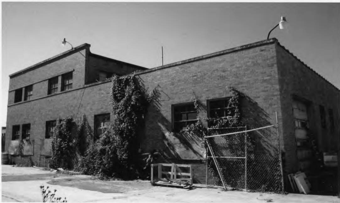
5. Columbia Central Fire Station 1001 Senate Street, Columbia Richland County, S.C.
