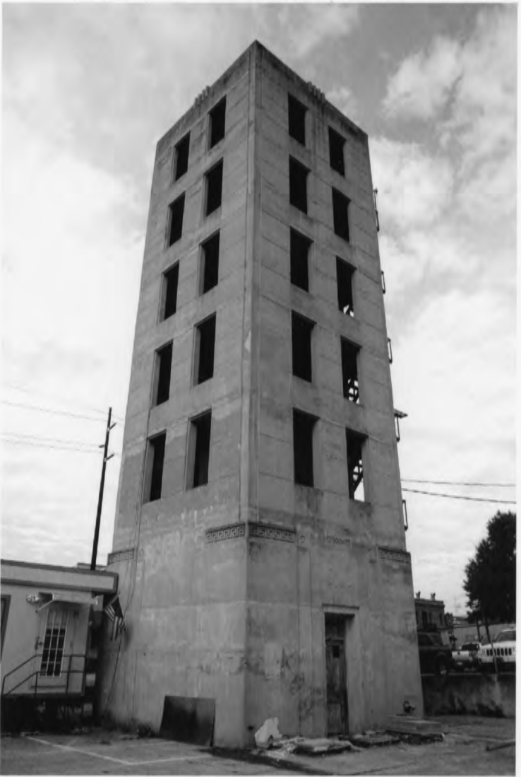
13. Columbia Central Fire Station 1001 Senate Street, Columbia Richland County, S.C.
