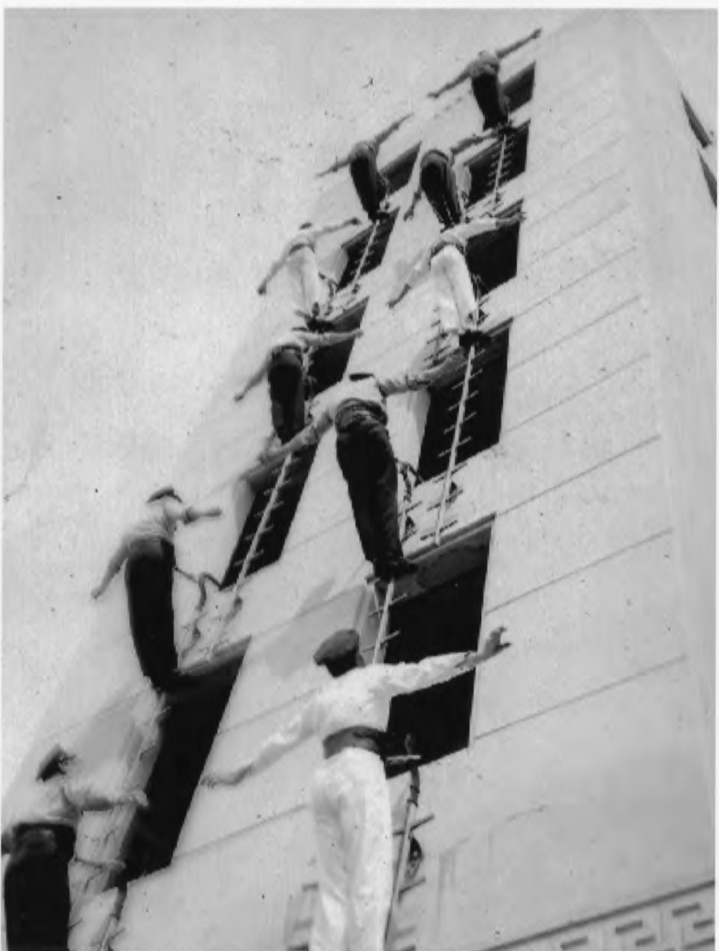
15. Columbia Central Fire Station
