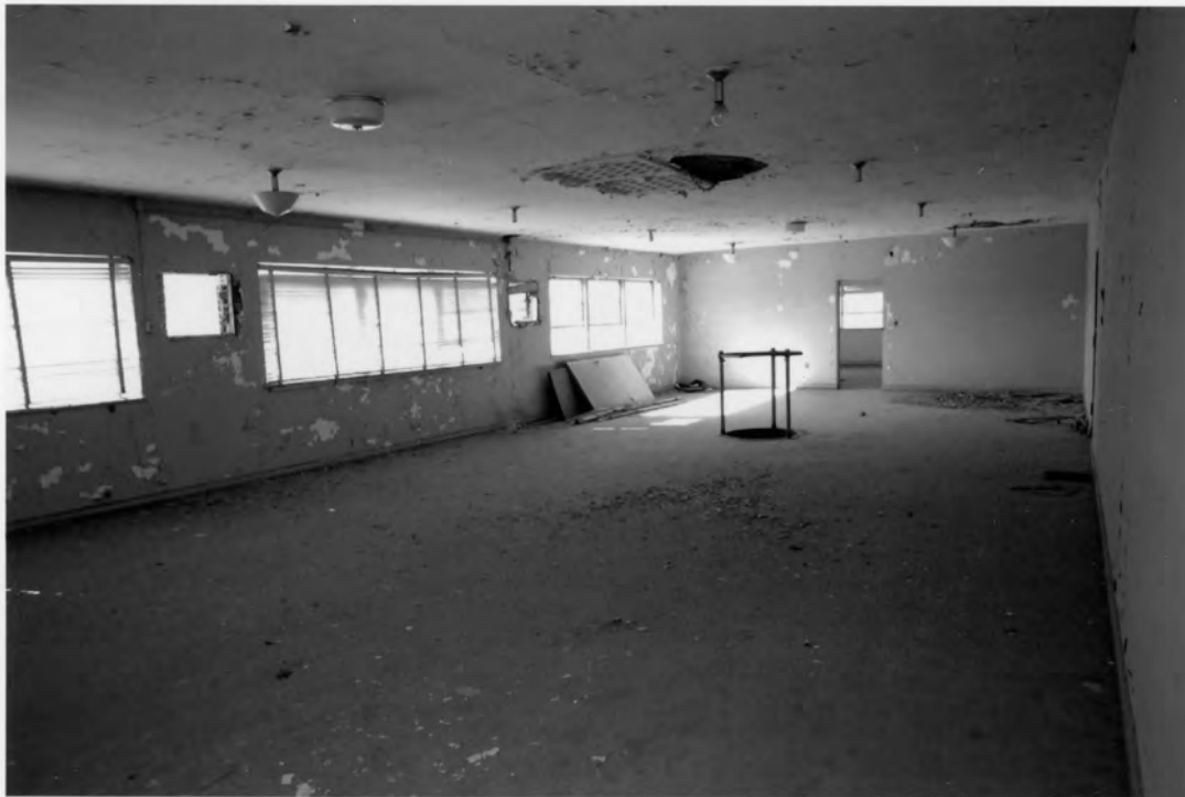
9. Columbia Central Fire Station 1001 Senate Street, Columbia Richland County, S.C.
