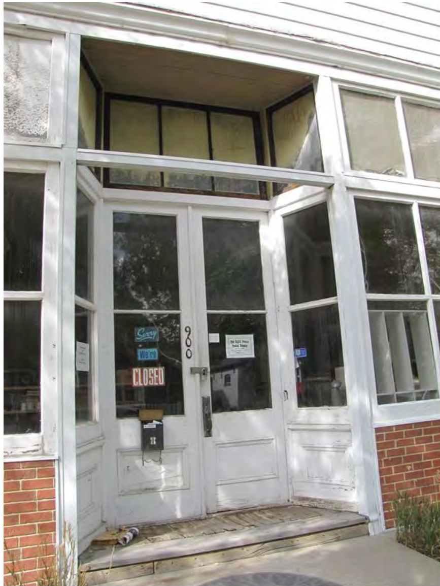
MT_LewisAndClarkCounty_DorseyGroceryAndResidence_0004. Grocery, façade (south), entry detail, view to N-NE.
