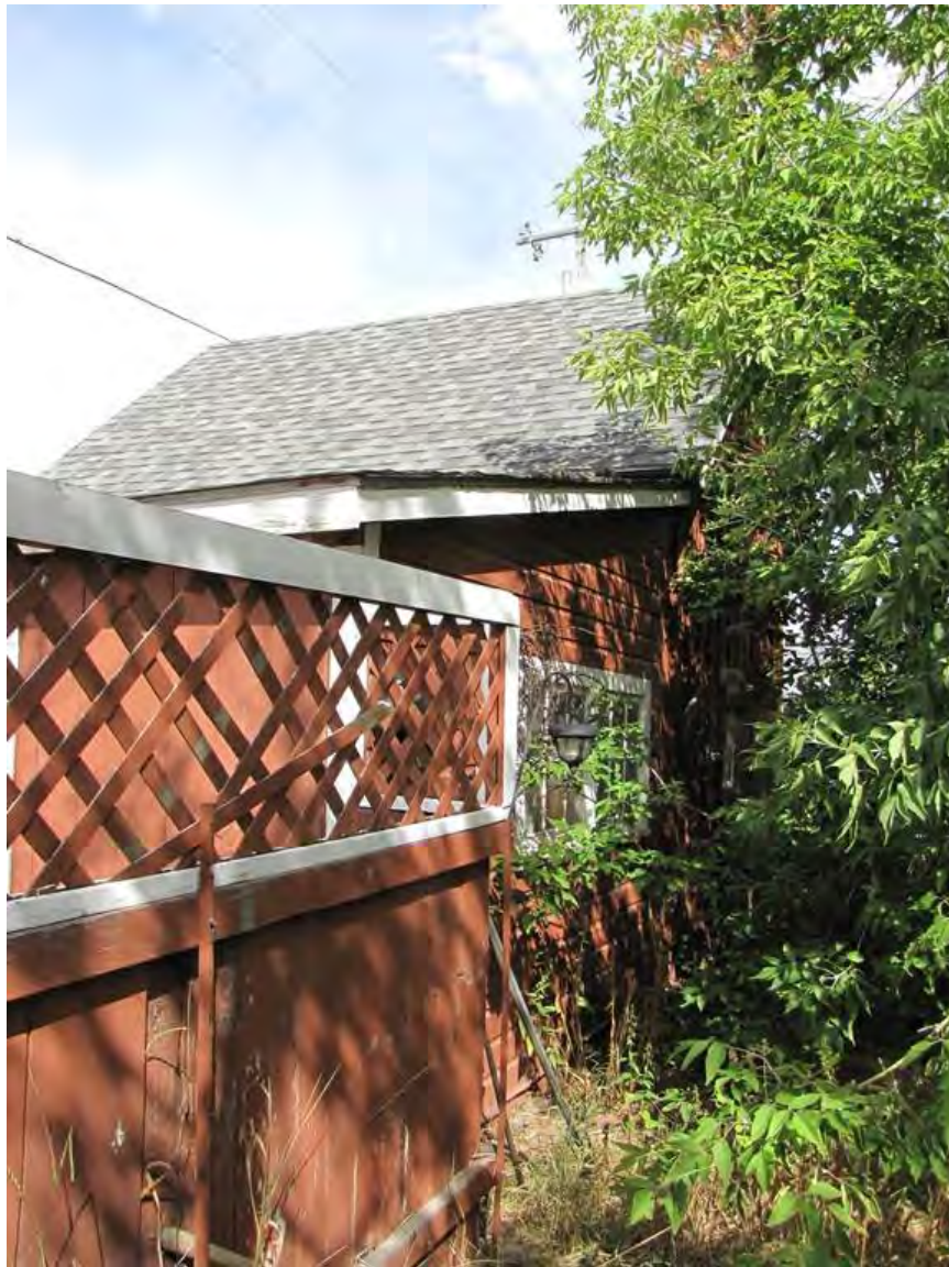
MT_LewisAndClarkCounty_DorseyGroceryAndResidence_0023. Garage/Carriage House, south wall, view to NE.
