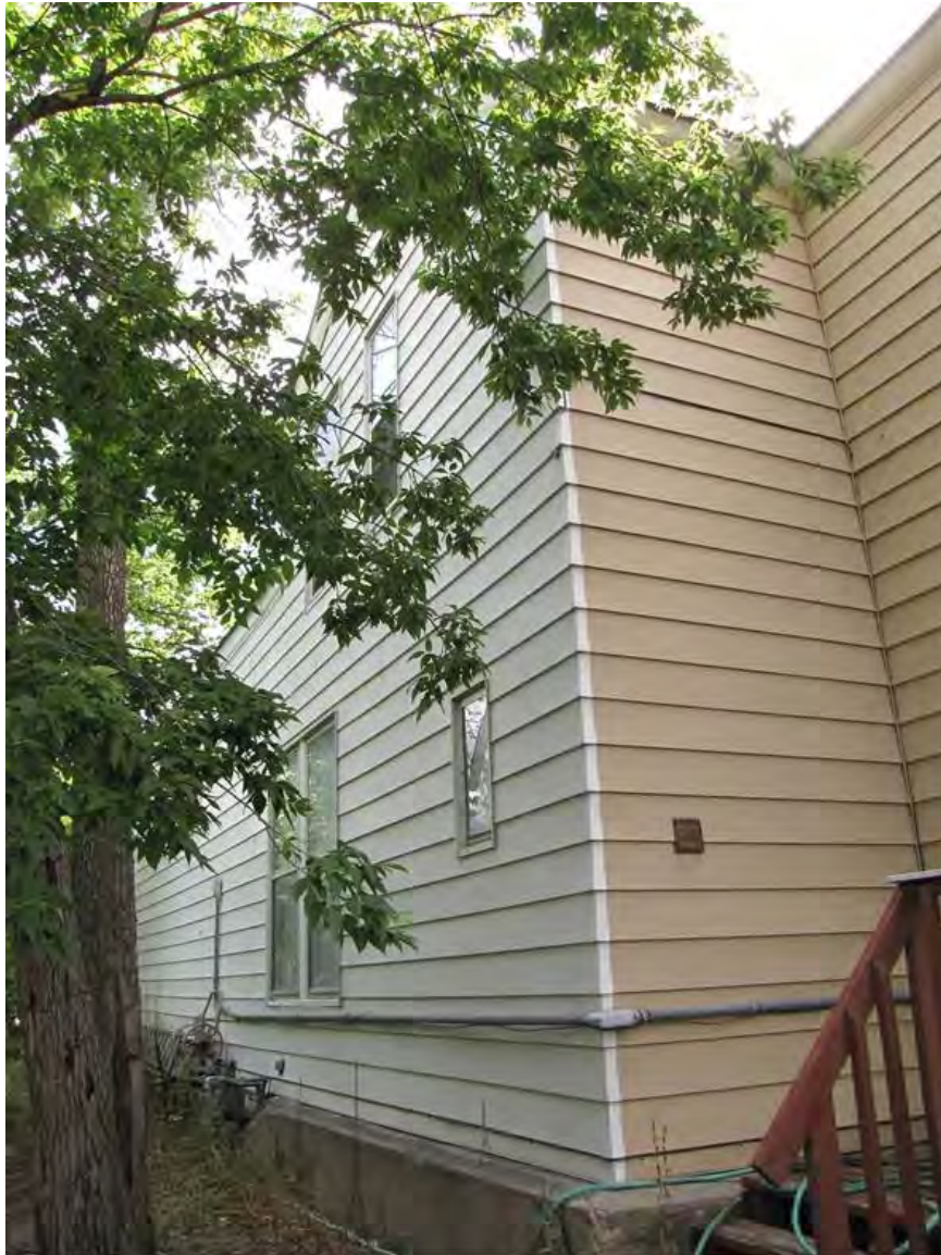
MT_LewisAndClarkCounty_DorseyGroceryAndResidence_0010. Residence, east wall, view to SW.
