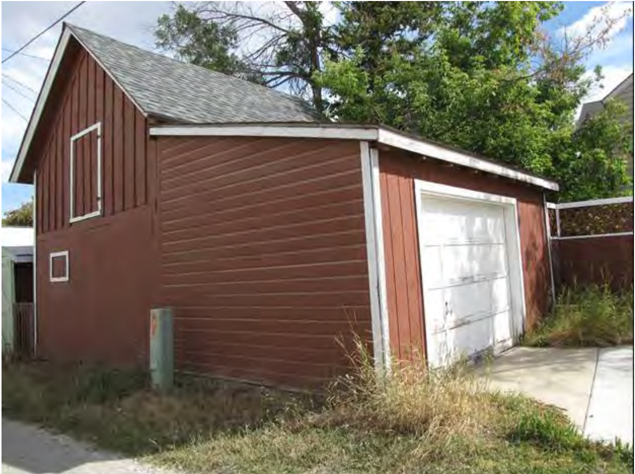
MT_LewisAndClarkCounty_DorseyGroceryAndResidence_0021. Garage/Carriage House, north and west walls, view to SE.
