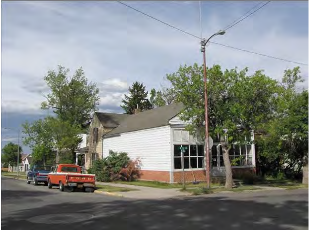
MT_LewisAndClarkCounty_DorseyGroceryAndResidence_0001. Overview, west wall and south façade, view to NE.
