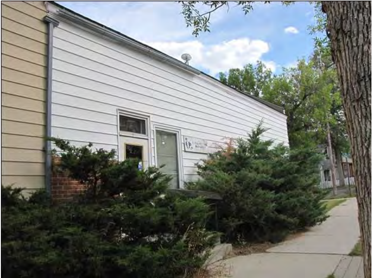
MT_LewisAndClarkCounty_DorseyGroceryAndResidence_0005. Grocery, west wall, view to SE.
