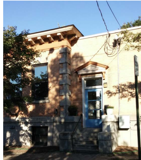
4. West elevation, original portion, and addition joined
