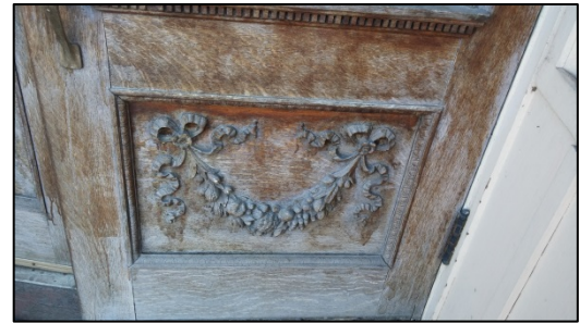
2. Close up of the door detailing
