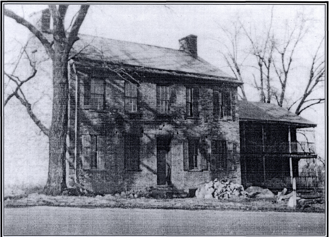
Fig. 2 This view of the property may date from the Mish family's 1929 remodeling, since it appears that construction debris is piled beside the main door. By this time, the original portico shown in Fig. 1 has been removed, but the joist morticing in the bricks is still visible.
