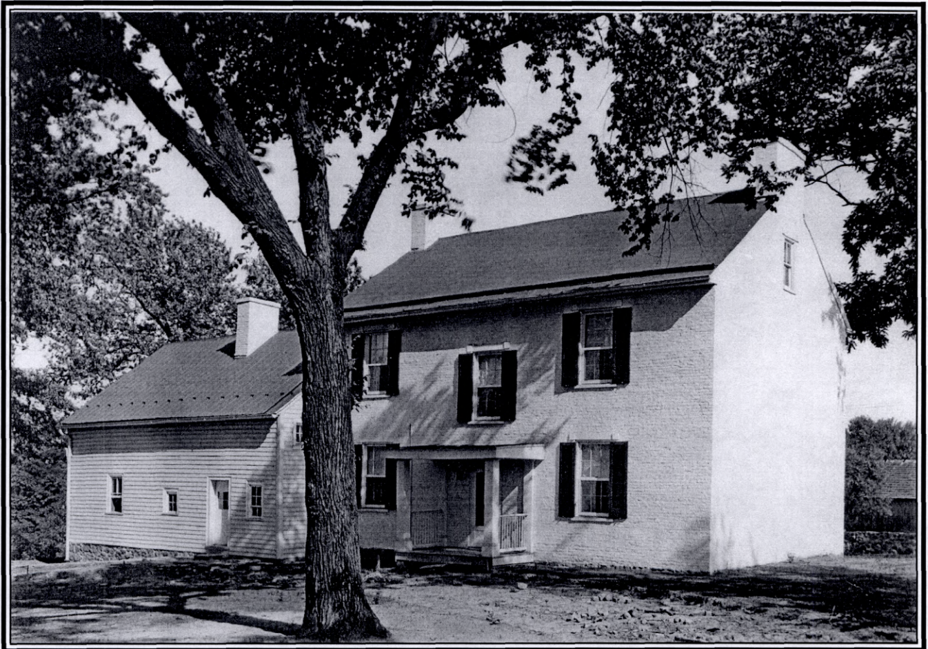
Fig. 4 Taken shortly after the Mish family completed their 1929 renovation of the house, this view shows the rear elevation of "Maidstone on the Potomac," including the eighteenth-century wood section at the left and the west elevation of the 1845 brick section.
