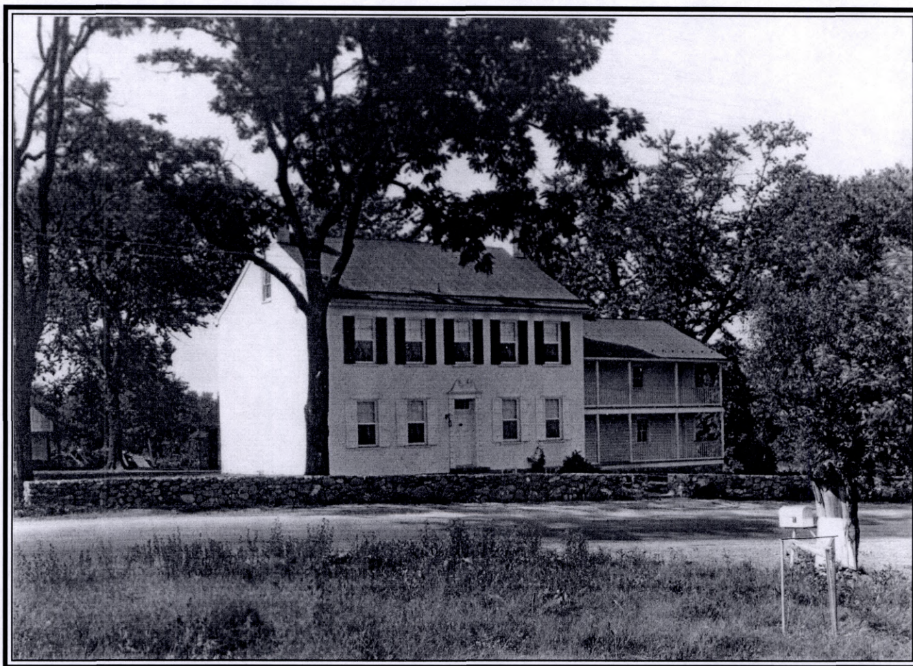
Fig. 3 This view of the facade and south gable end of "Maidstone on the Potomac" likely was taken shortly after the Mish family completed their 1929 renovation of the house. It shows the broken pediment-and-quoins frontispiece which replaced the original modest portico on the 1845 brick section. Also clearly shown is the earlier log section at the right, with the double-gallery porch.
