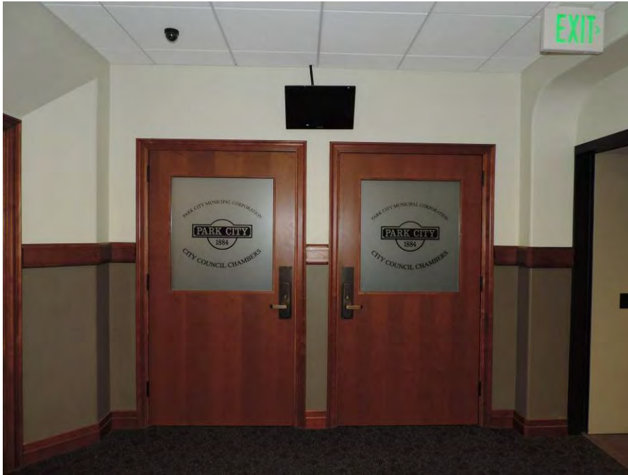
Photo 19 of 21: Corridor wainscoting detail, which replaced historically nonconforming finishes in 2009 renovation. August 29, 2014.
