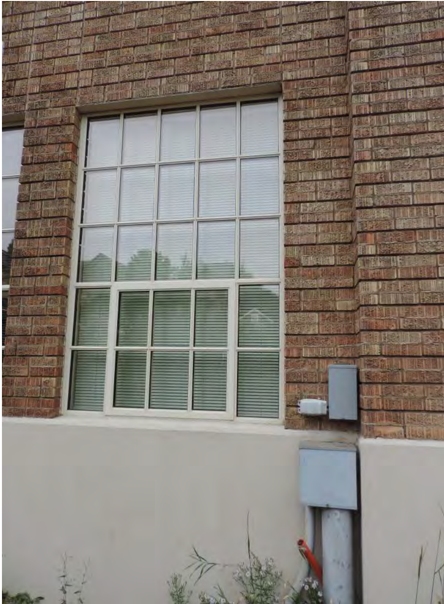
Photo 13 of 21: Typical window detail. Outdated windows were replaced in 2009 with high efficiency ones. August 27, 2014.
