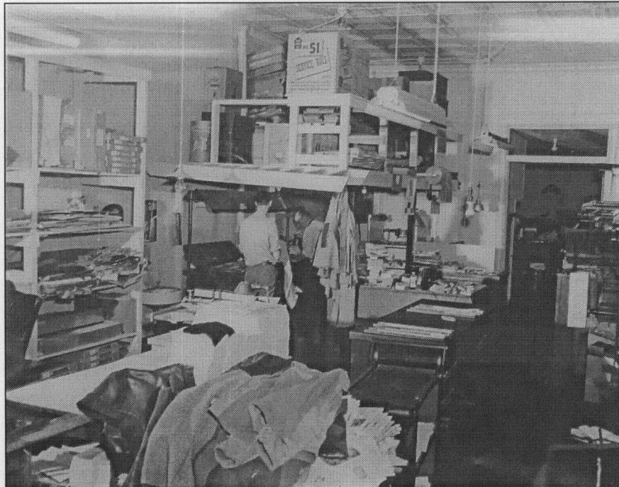
Figure 16: Pre-1953 remodeling, view southeast, the suspended storage area at center, set beneath the pressed metal ceiling, evolved into an enclosed attic with drop stairs (Courtesy of Linda Sidey)
