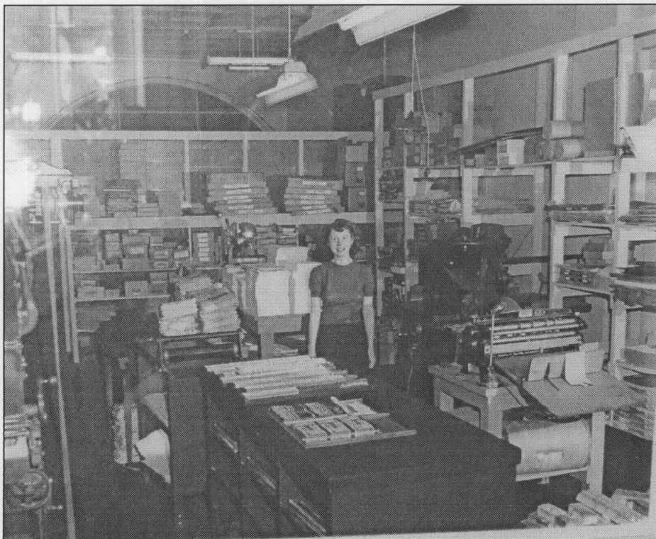
Figure 17: Pre-1953 remodeling photo showing dividing wall for front office, view northeast, c.1950 (note ceiling) (Courtesy of Linda Sidey)
