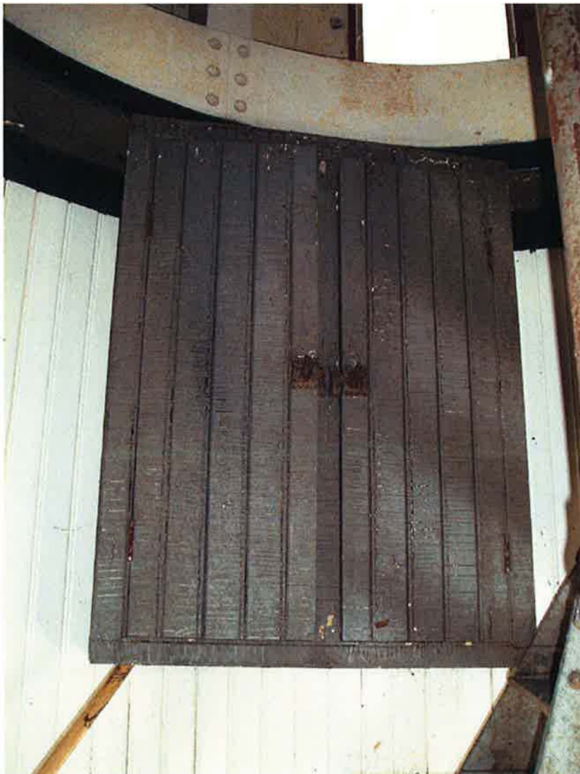
Photo 3. Lighthouse watch room storage cabinet, camera facing north.
