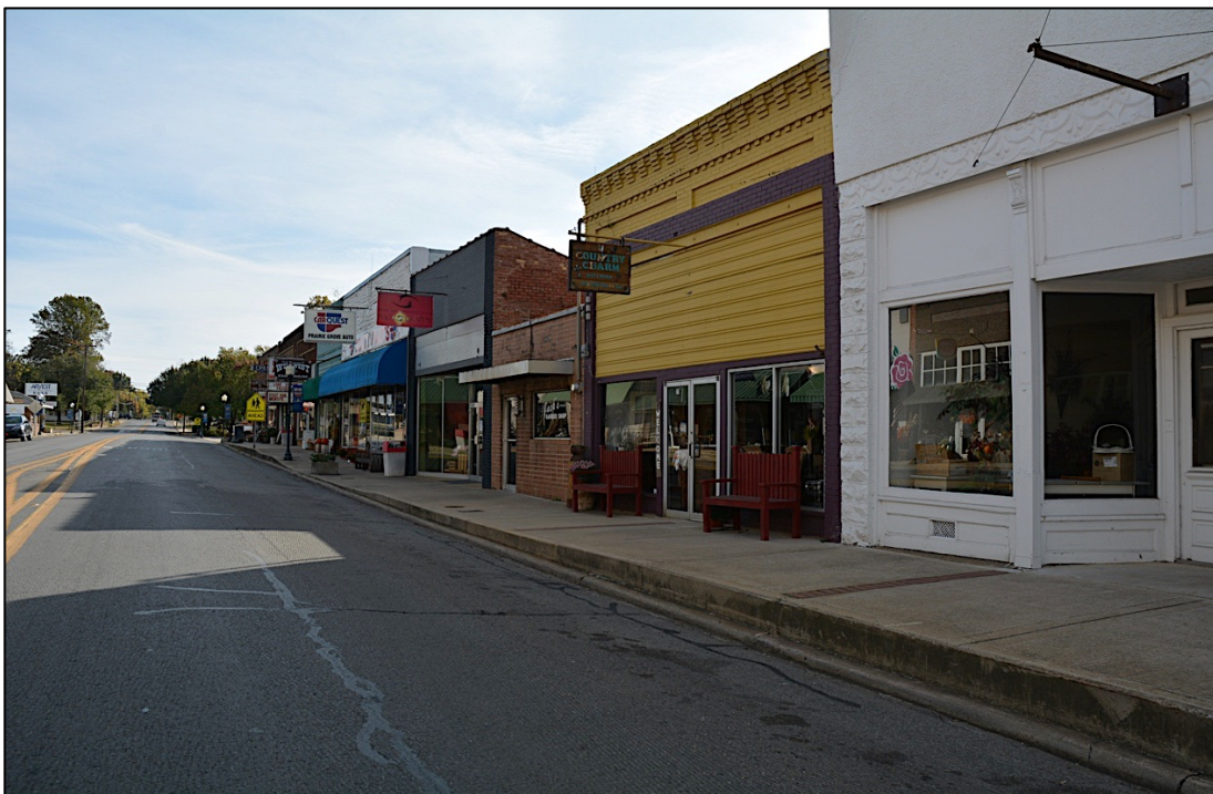
Photo 4. View of the Prairie Grove Commercial District (southern side of East Buchanan Street); facing southeast.
