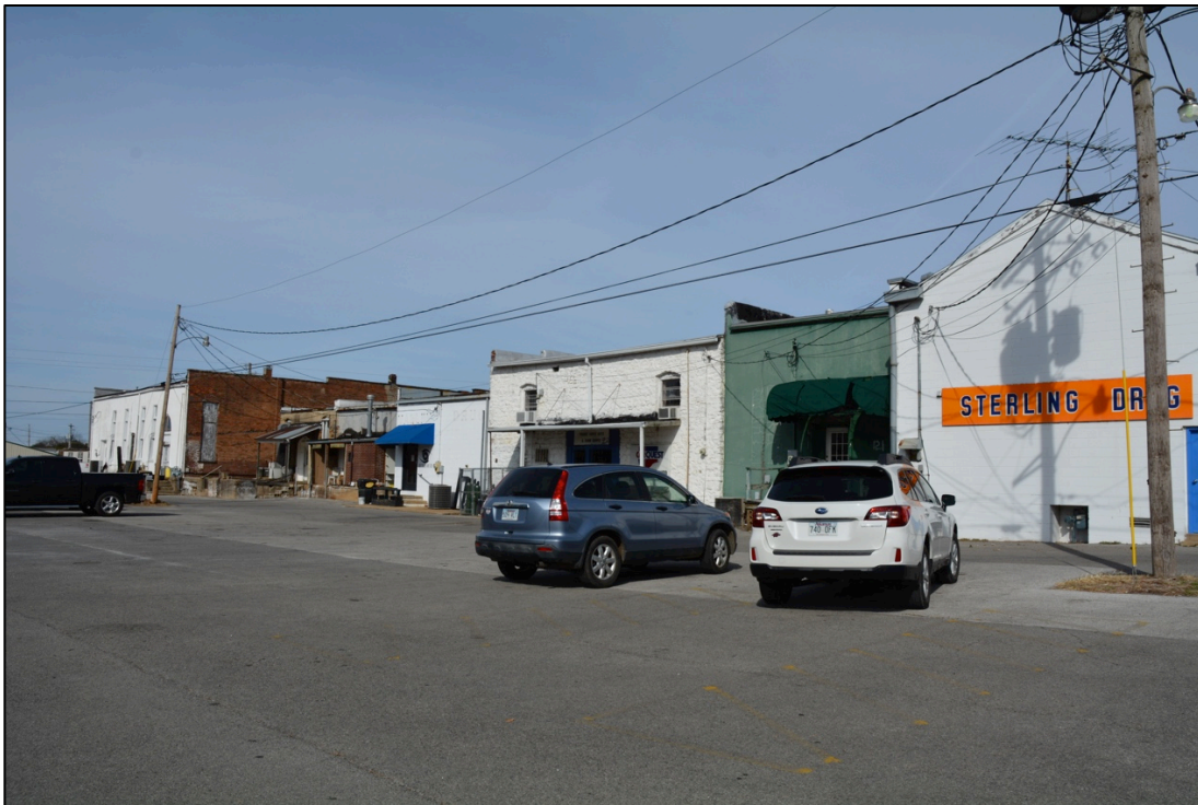
Photo 14. View of rear entrances from southern parking lot; facing northwest.
