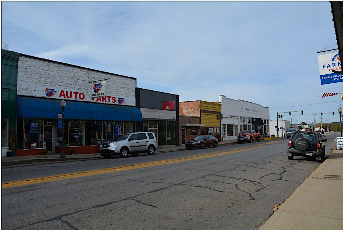
Photo 5. View of western part of the Prairie Grove Commercial Historic District (119–107 East Buchanan Street); facing southwest.
