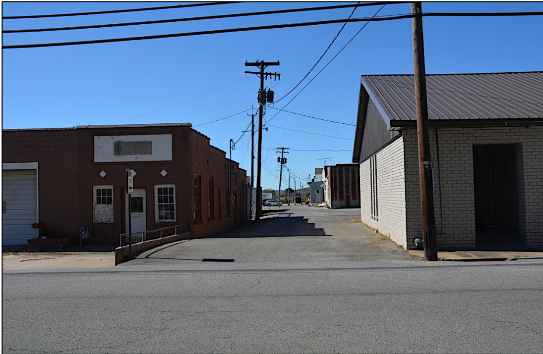
Photo 13. View of southern boundary line (alley/parking lot) from 123 South Neal Street; facing west.
