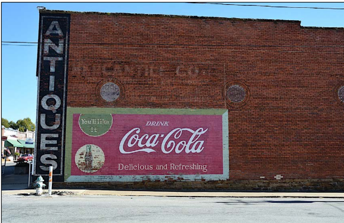
Photo 22. Signage on western side of 107 East Buchanan Street (Southern Mercantile Company); facing east.
