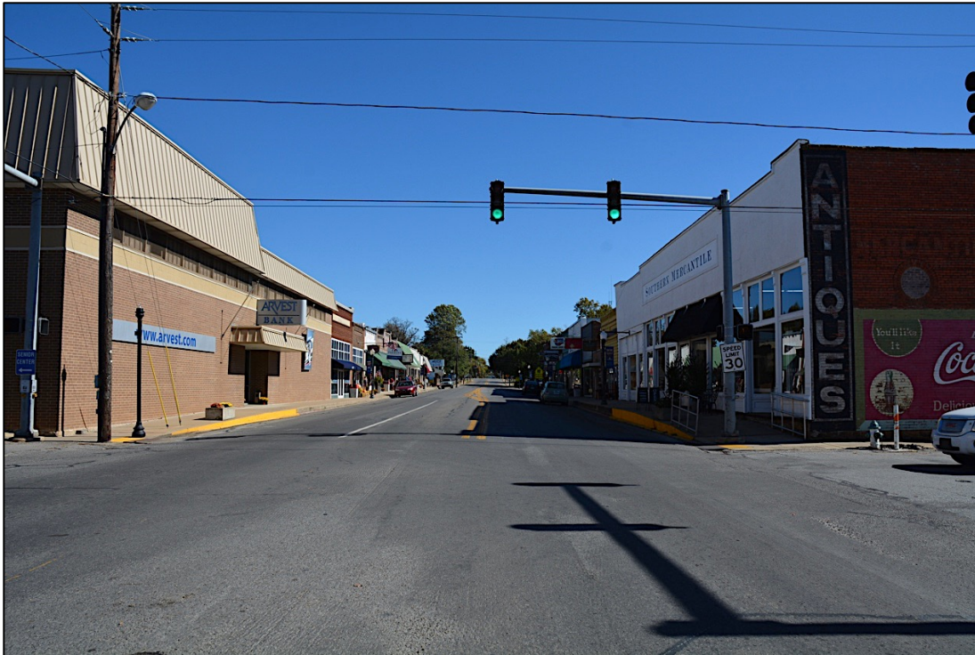
Photo 1. View from East Buchanan Street from Mock Street; facing east. The Prairie Grove Commercial Historic District (WA1652) is on the right side of the photograph.
