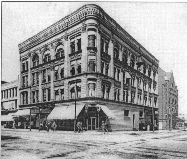
Figure 17: 1897 view of the Security Building (Loras College; Center for Dubuque History)
