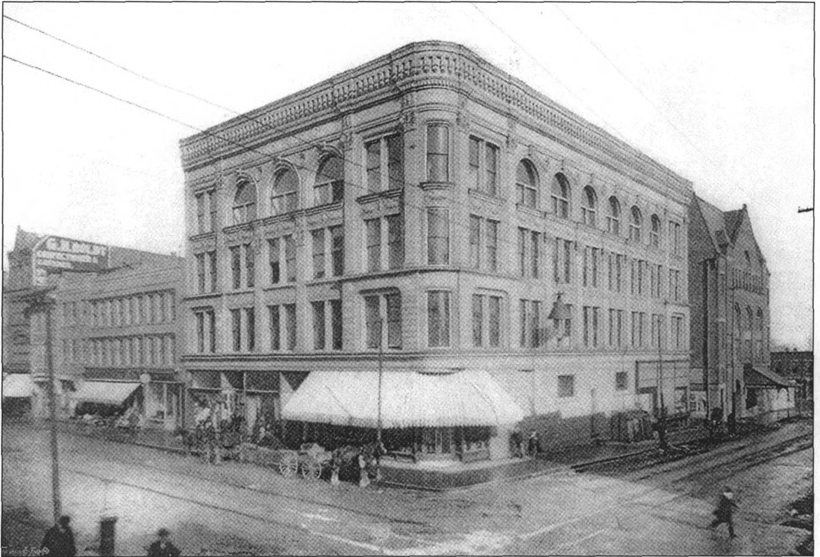
Figure 16: Newly completed Security Building, 1897, Grand Opera House visible at the right, Althauser Building, removed for 1907 expansion, is to the left
