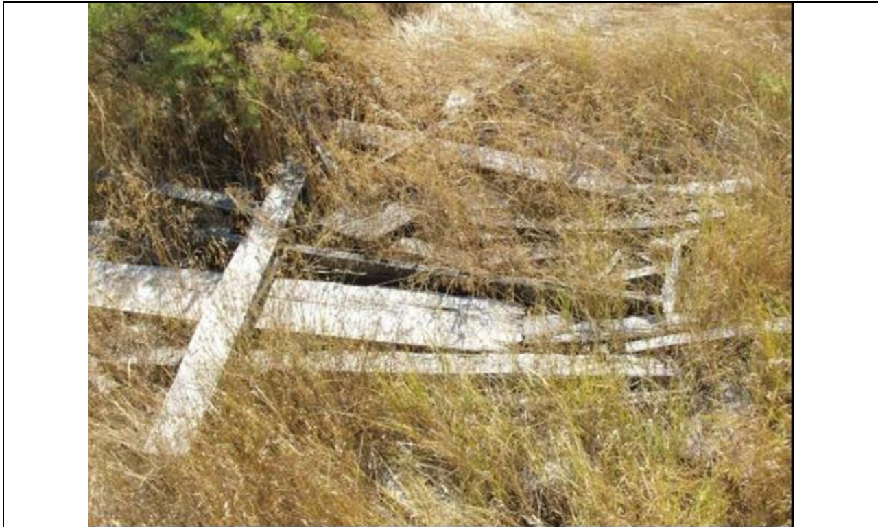
MT_Blaine County_Ervin Homestead/GistBottom_HD_0012 Ervin Outhouse. View looking south.
