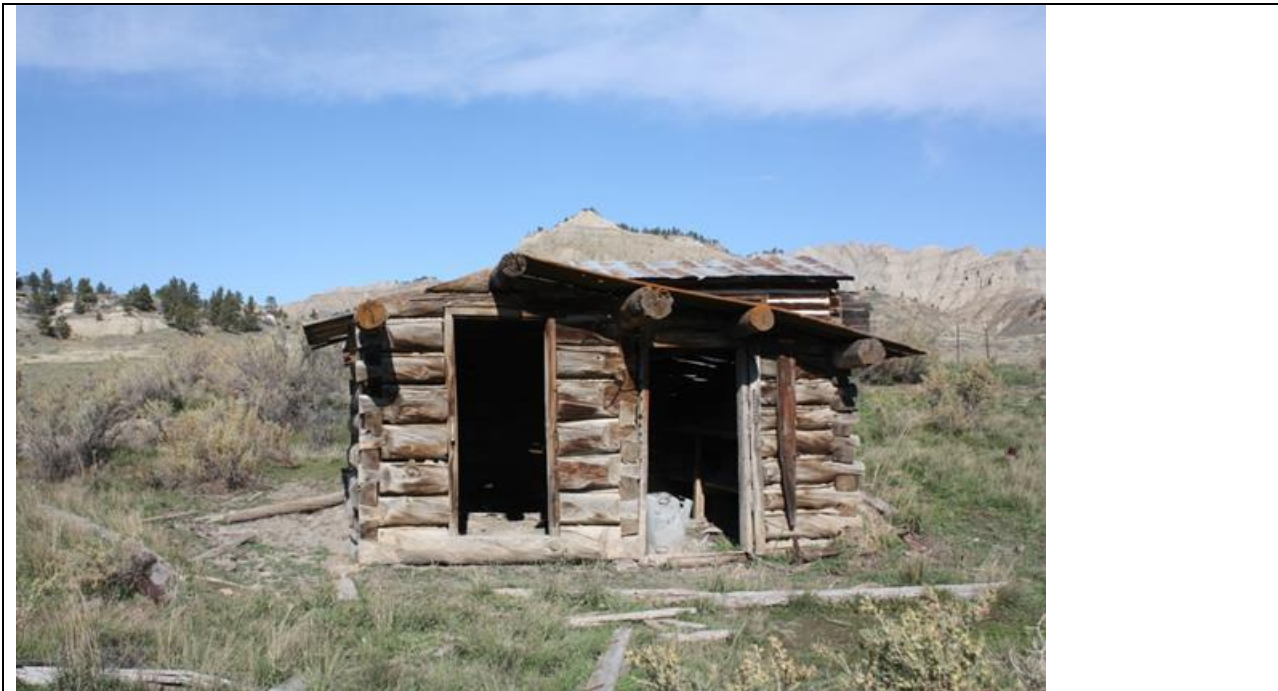
MT_Blaine County_Ervin Homestead/GistBottom_HD_0016 Gist Cabin #1. South elevation. View to the north.
