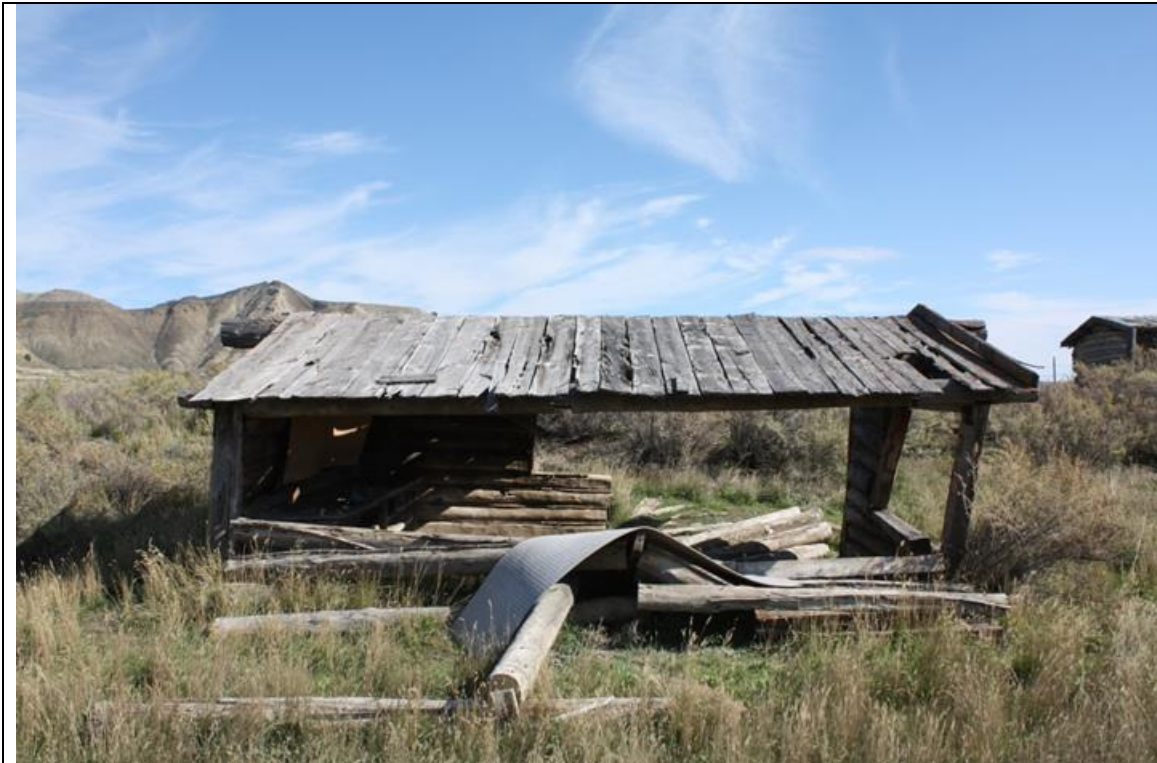
MT_Blaine County_Ervin Homestead/GistBottom_HD_0036 Gist Log shop. West elevation. View to the east.
