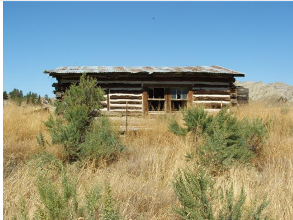
MT_Blaine County_Ervin Homestead/GistBottom_HD_0022 Gist Residence. South elevation. View to the north.
