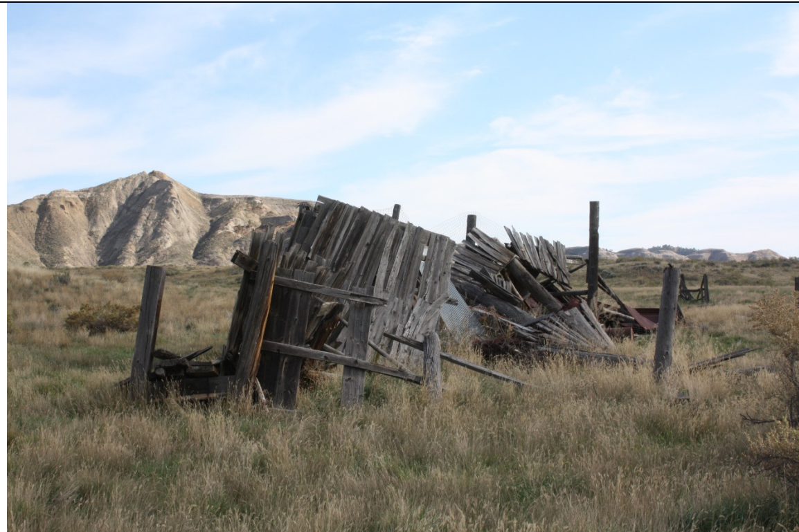
MT_Blaine County_Ervin Homestead/GistBottom_HD_0053 Gist Barn. View to the west.
