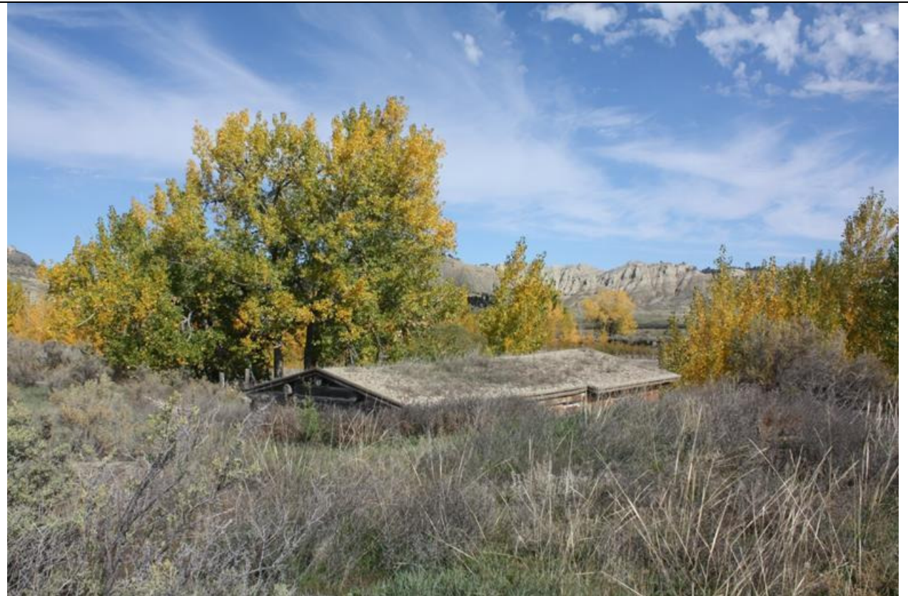
MT_Blaine County_Ervin Homestead/GistBottom_HD_0003 West and south elevations of Ervin Cabin, view to the northeast.
