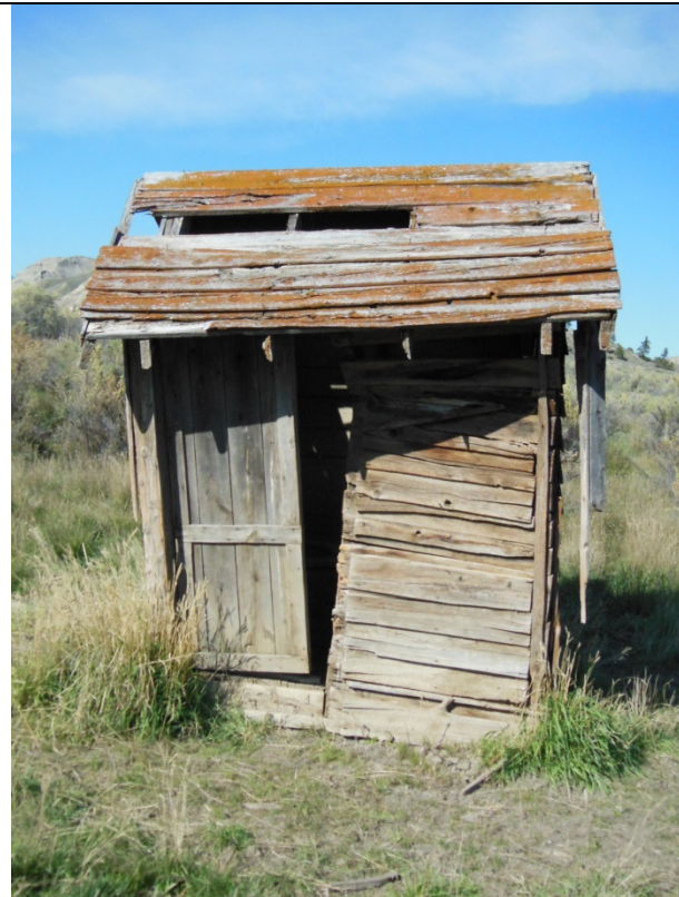
MT_Blaine County_Ervin Homestead/GistBottom_HD_0043 Gist Outhouse. South elevation. View to the north.
