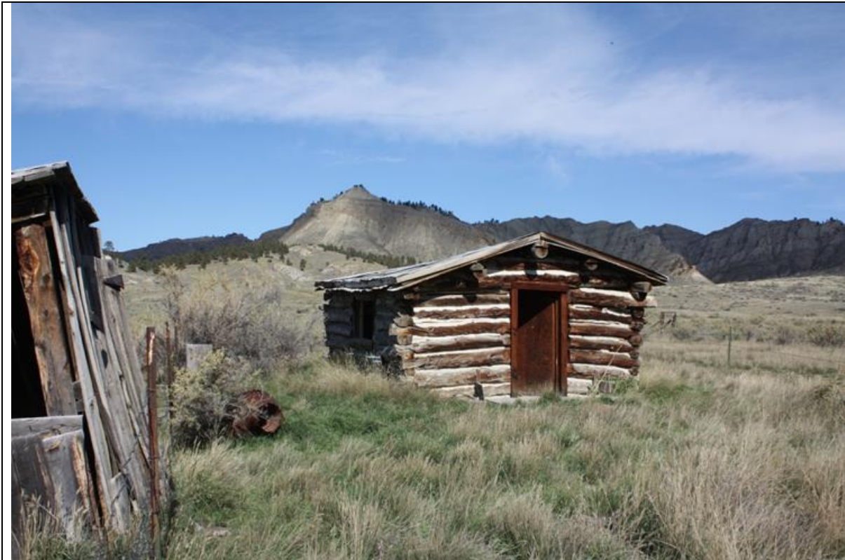
MT_Blaine County_Ervin Homestead/GistBottom_HD_0032 Gist Cabin #2. West and south elevations. View to the northeast.
