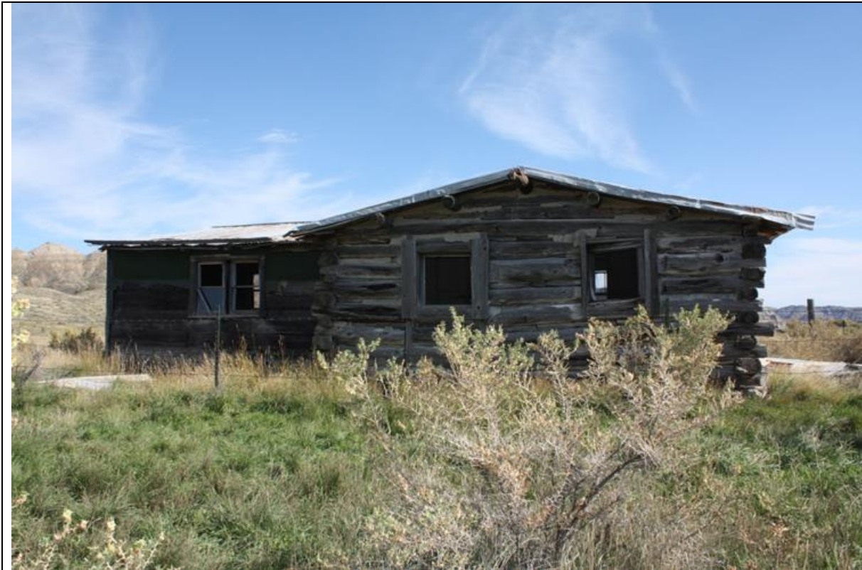
MT_Blaine County_Ervin Homestead/GistBottom_HD_0027 Gist Residence. West elevation. View to the east.
