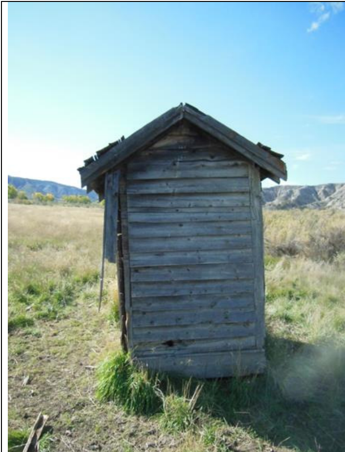
MT_Blaine County_Ervin Homestead/GistBottom_HD_0046 Gist Outhouse. West elevation. View to the east.
