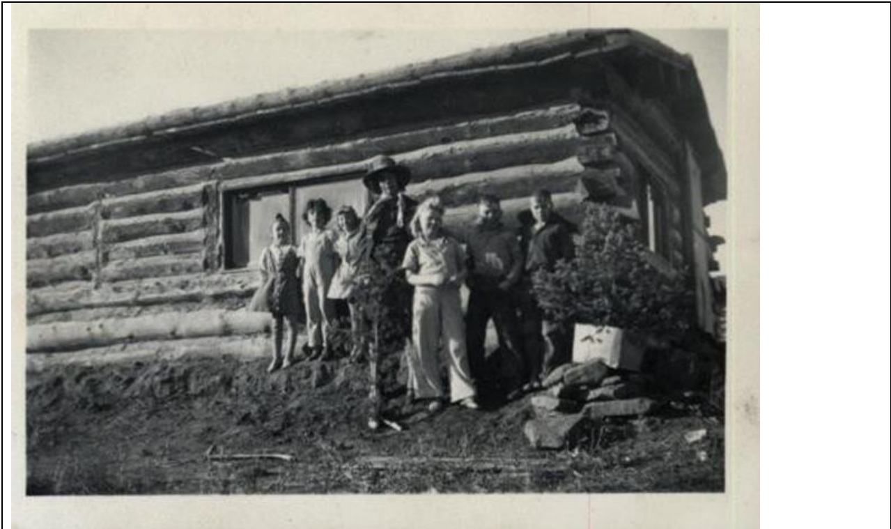
MT_Blaine County_Ervin Homestead/GistBottom_HD_0063 Gist children, ca. 1940. Standing on south side of Building #2, when it was still the Gist School. View to the northwest. Photo courtesy Jack Gist.
