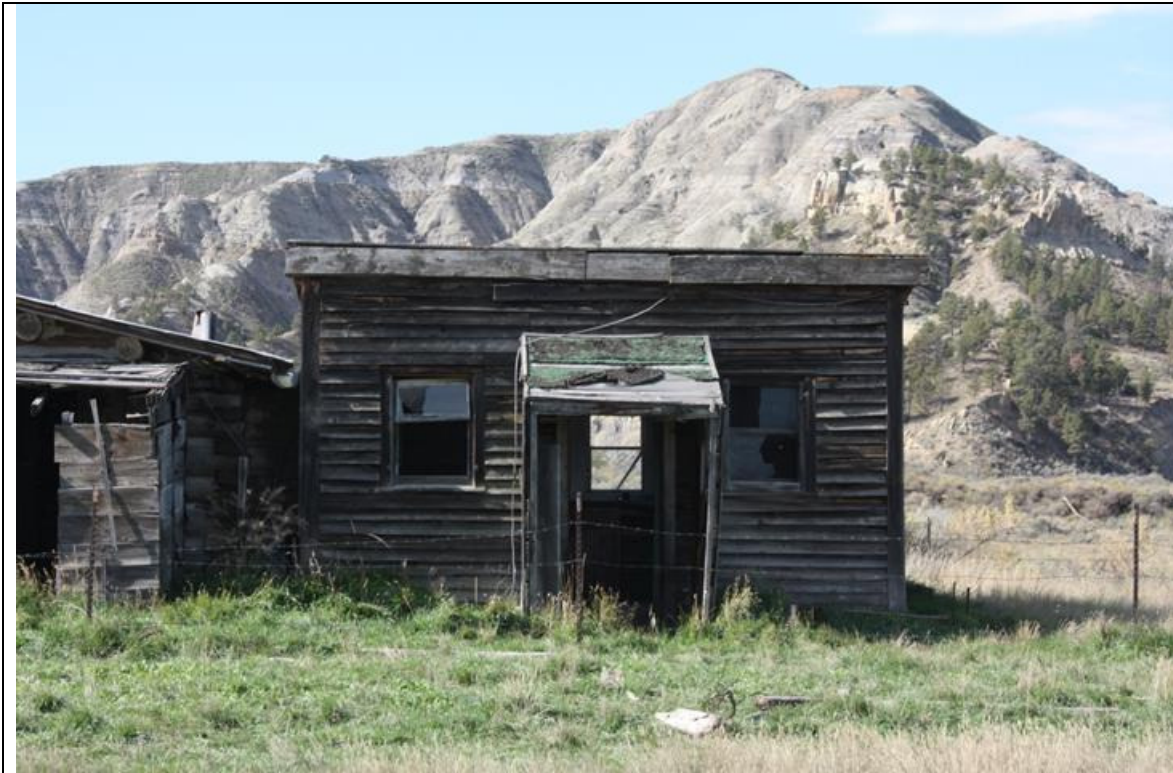
MT_Blaine County_Ervin Homestead/GistBottom_HD_0025 Gist Residence. Detail of north wing. East elevation. View to the west.
