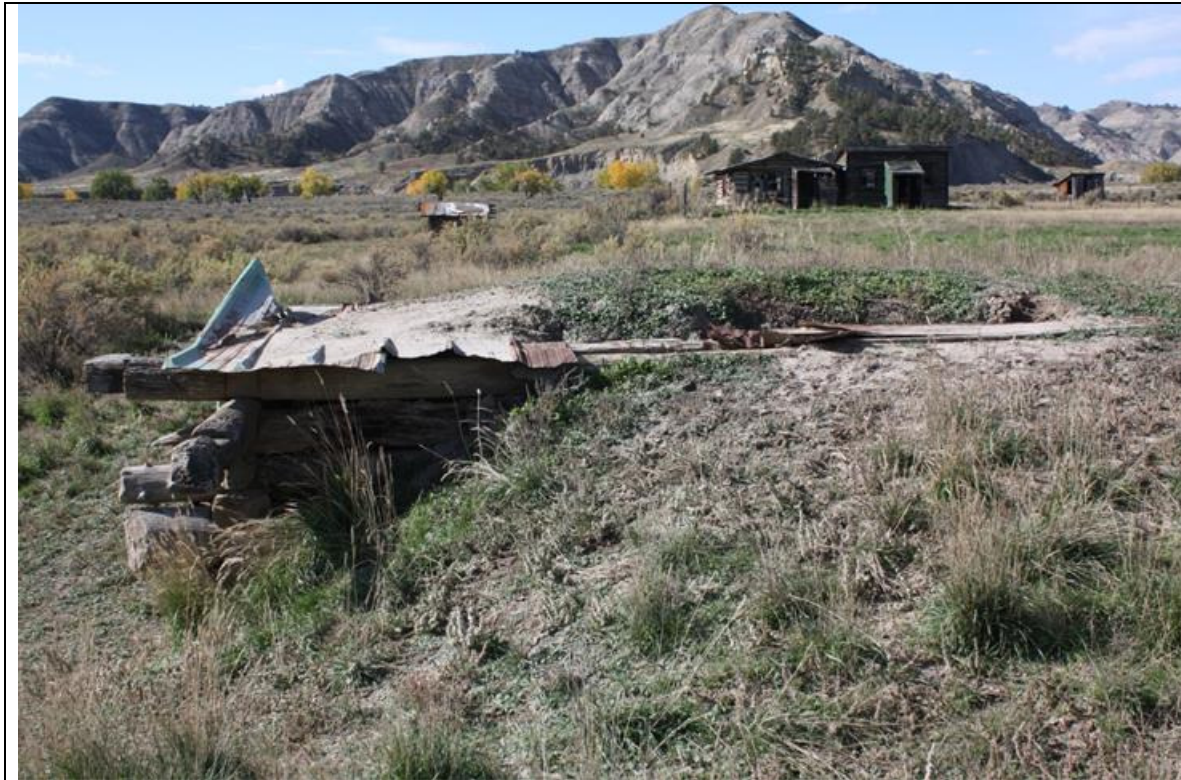
MT_Blaine County_Ervin Homestead/GistBottom_HD_0040 Gist Dugout Shed #1, Dugout shed. East elevation. View to the west.
