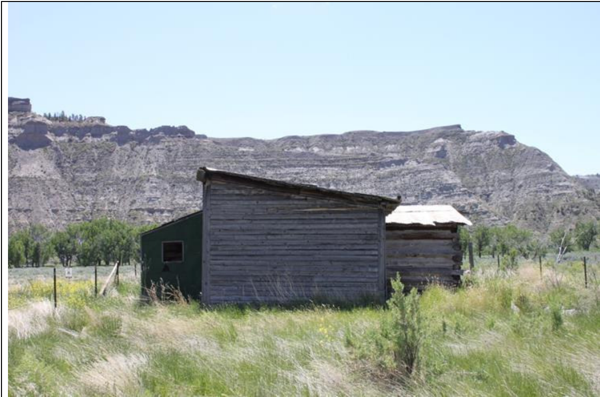
MT_Blaine County_Ervin Homestead/GistBottom_HD_0026 Gist Residence. North elevation. View to the south.
