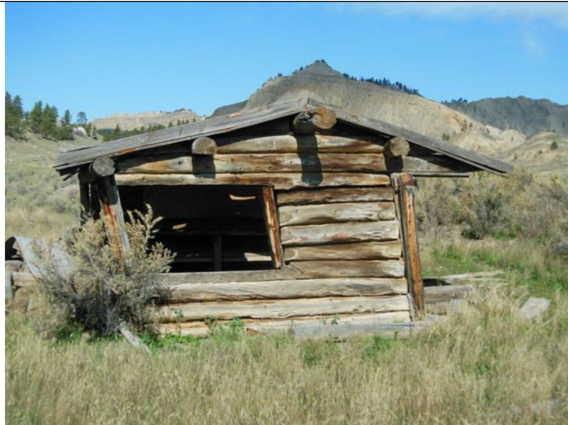
MT_Blaine County_Ervin Homestead/GistBottom_HD_0035 Gist Log shop. South elevation. View to the north.
