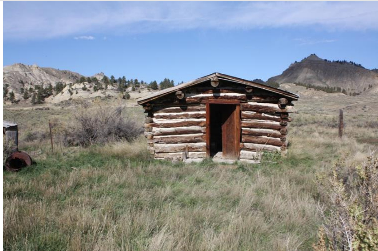
MT_Blaine County_Ervin Homestead/GistBottom_HD_0029 Gist Cabin #2. South elevation. View to the north.
