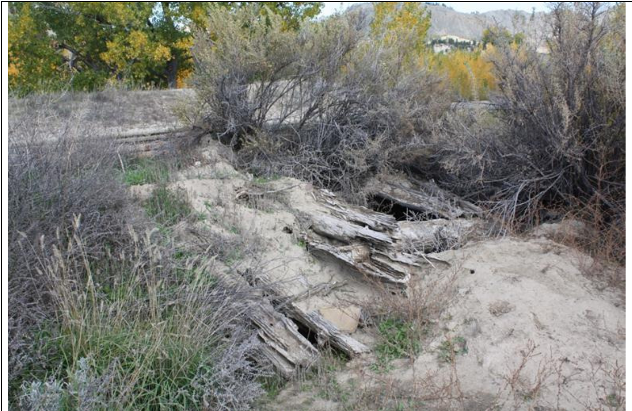
MT_Blaine County_Ervin Homestead/GistBottom_HD_0010 Ervin Cellar, view looking south at roof.
