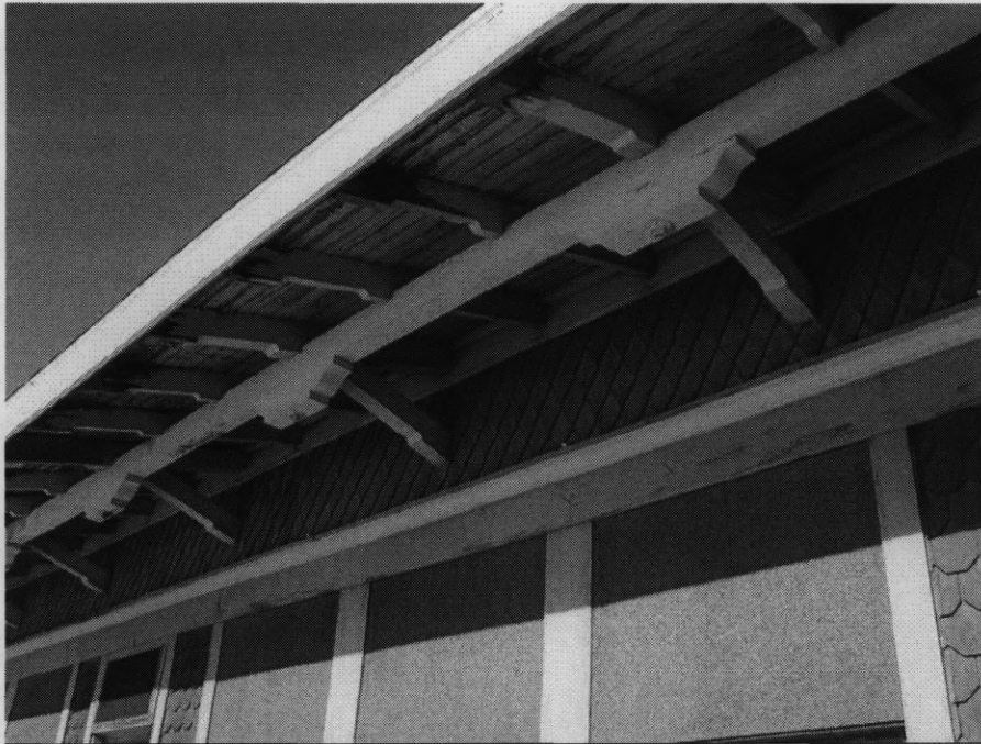
Photo 0021. Detail of frieze, rafters, and brackets of Montana, Wyoming & Southern Railroad Depot. View to the northwest.
