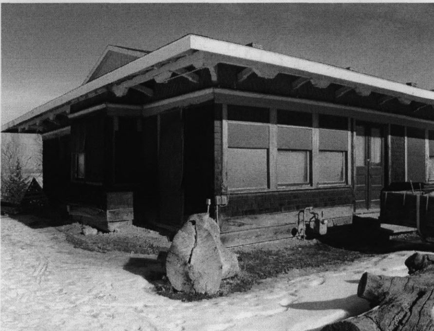
Photo 0020. West elevation and south façade of Montana, Wyoming & Southern Railroad Depot. View to the northeast.
