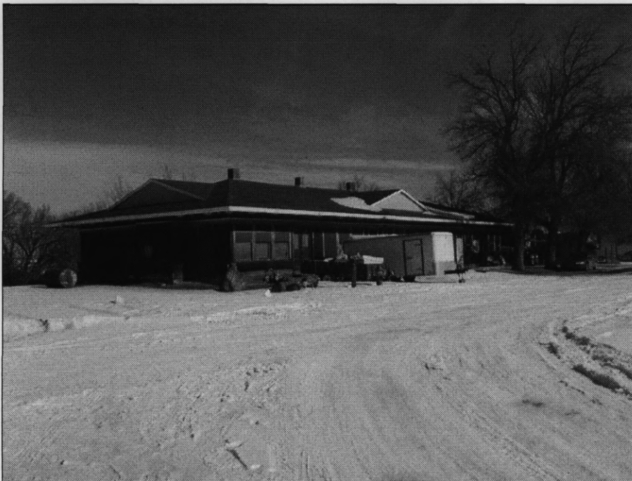
Photo 0004. South façade of Montana, Wyoming & Southern Railroad Depot. View to the northeast.
