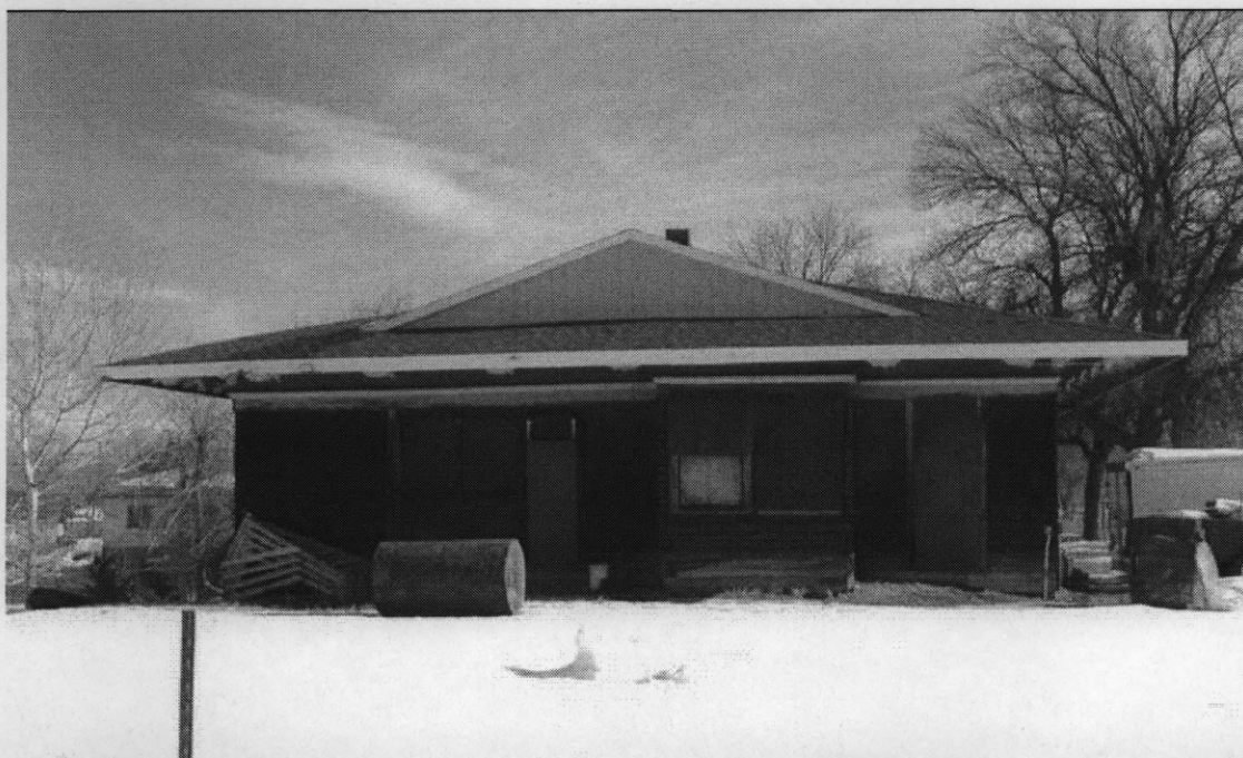
Photo 0018. West elevation of the Montana, Wyoming & Southern Railroad Depot. View to the east.
