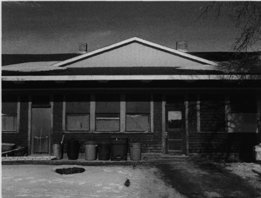
Photo 0007. Detail of entry into railroad office of Montana, Wyoming & Southern Railroad Depot. South façade. View to the north.
