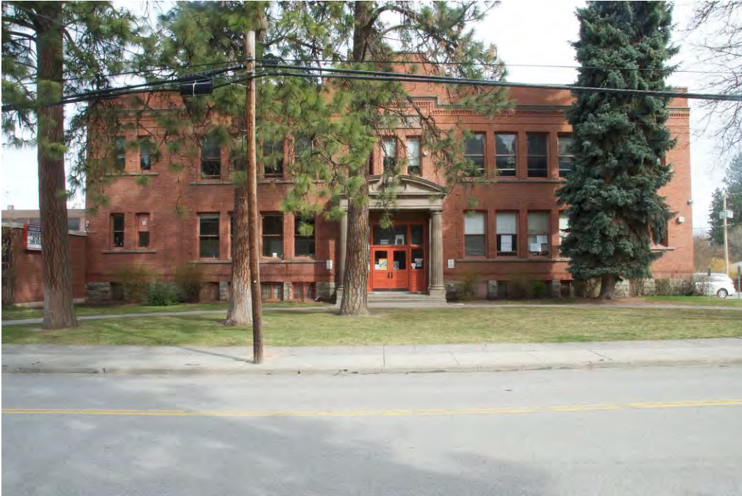
2 of 28 Main Façade - Looking north
