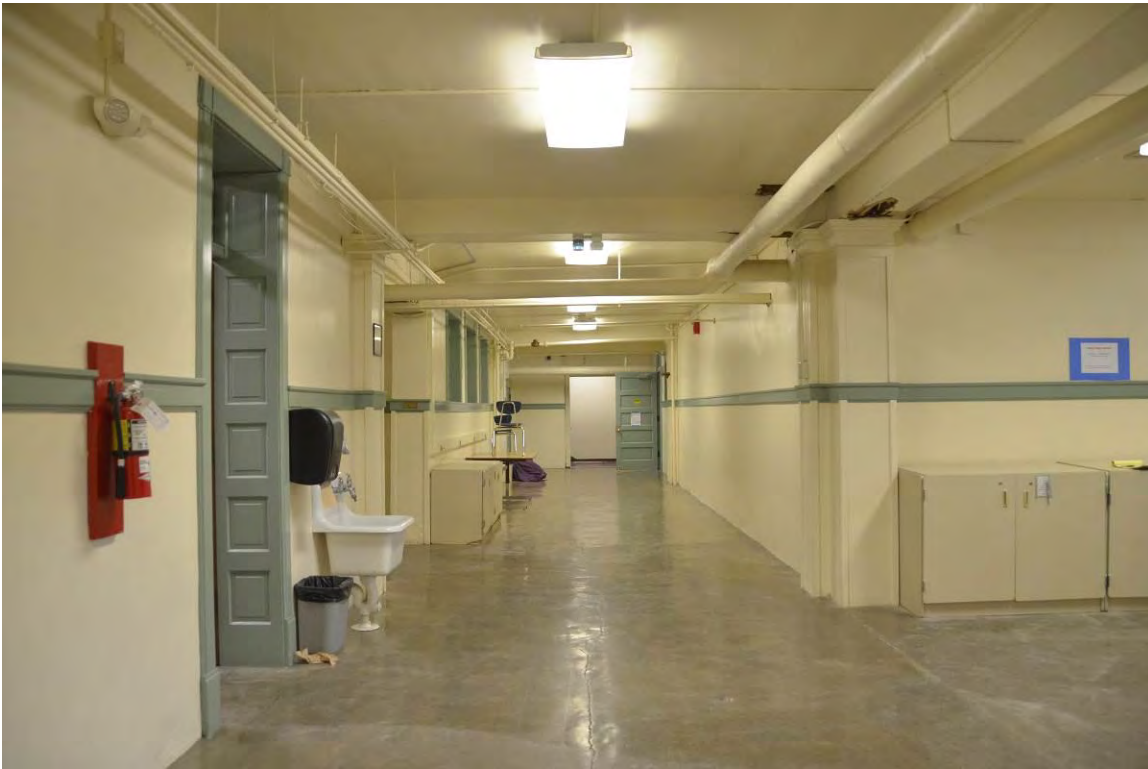
20 of 28 1909 building, Basement Hall looking west
