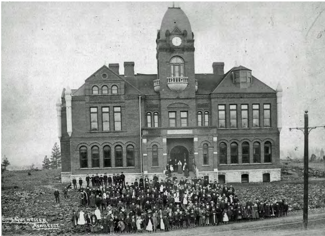
View of original Franklin School located at Front St (now E. Spokane Falls Blvd & S. Grant St) directly across from the Northern Pacific Roundhouse. (Emil Guenther, architect)
