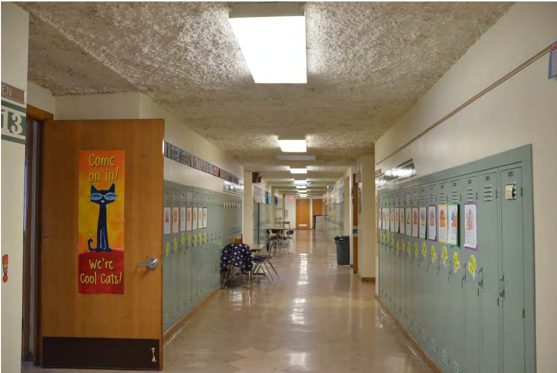
22 of 28 1953 addition, classroom hallway looking west.
