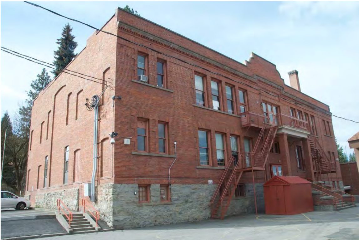
4 of 28 Rear façade, northeast corner - Looking southwest
