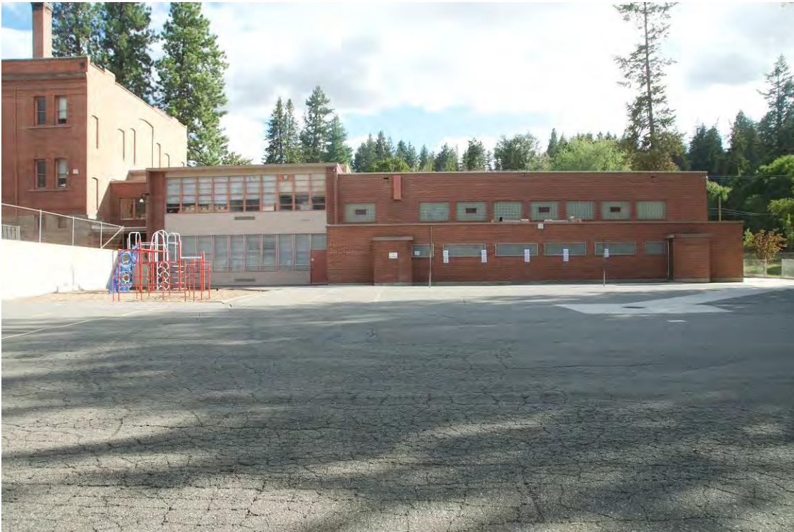
8 of 28 Rear facade of 1953 addition - Looking south
