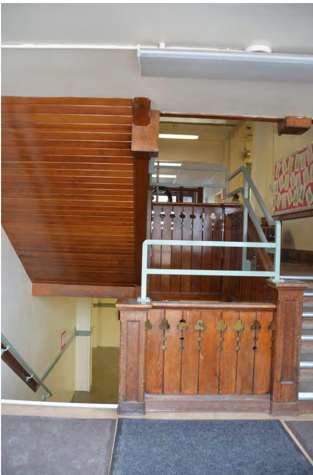
19 of 28 1909 building, Stair railing detail.
