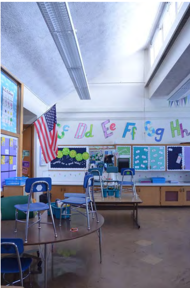
25 of 28 1953 addition, Typical classroom with clearstory window.
