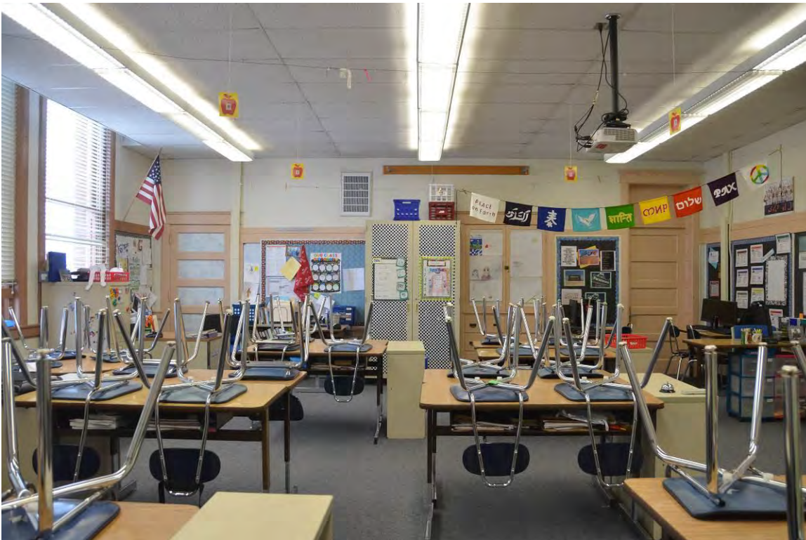
15 of 28 1909 building, Typical classroom space (room 106).
