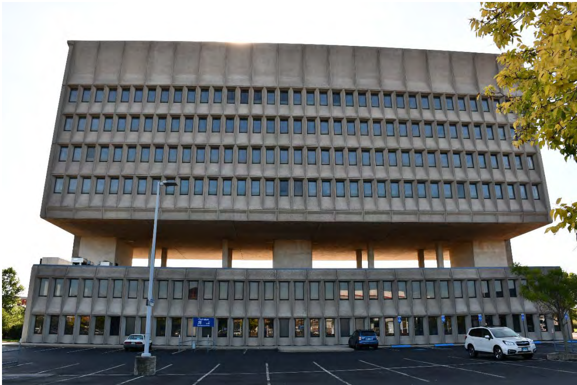
6 of 38. West elevation, facing east (9/13/19).
