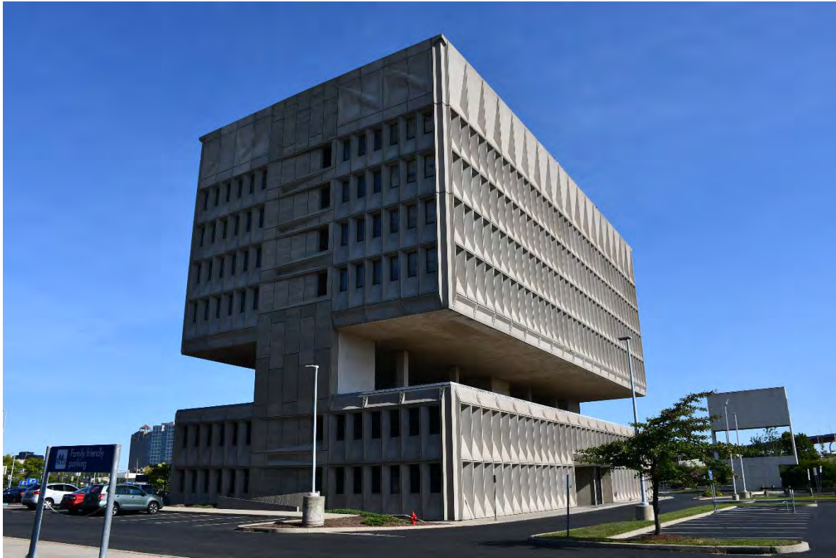
8 of 38. East and south elevations, facing northwest (9/13/19).
