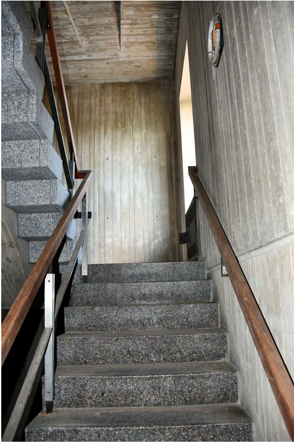
14 of 38. First floor stairwell, facing west (9/13/19).
