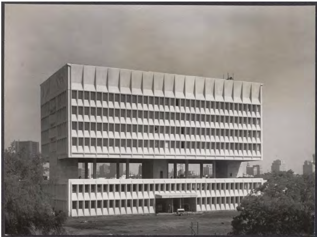
Figure 6: Construction photograph of the Armstrong Rubber Company Building, view towards east elevation, 1969 (Source: Syracuse University Libraries 2018)
