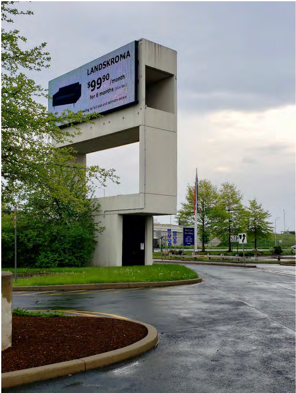
9 of 38. Sign Structure, north and west elevations, facing southeast (5/17/19).
