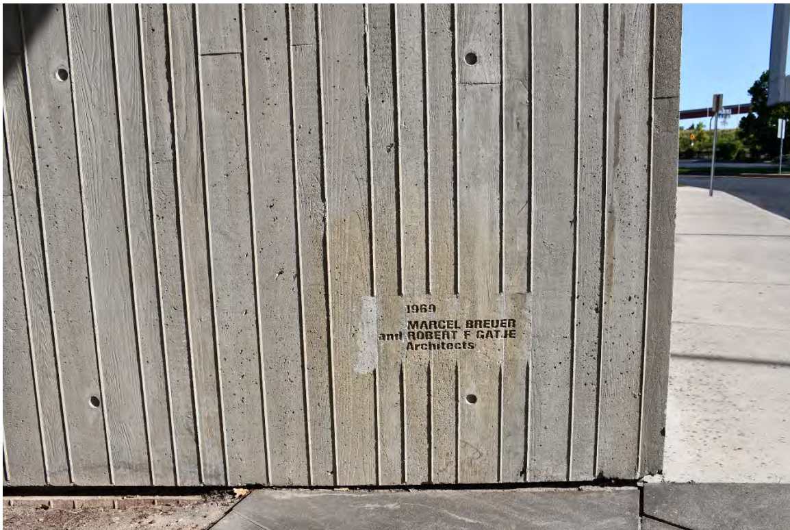
4 of 38. East elevation, date stamp detail, facing north (9/13/19).
