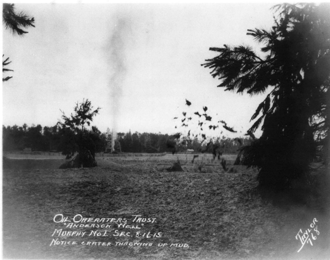
Figure 1: The Oil Operator's Trust, Murphy No. 1 on the 15th of May. The great rush of escaping natural gas can be clearly seen at the destroyed derrick. Escaping gas also opened smaller craters nearby. Courtesy the Arkansas Museum of Natural Resources (1996-041-0016).
