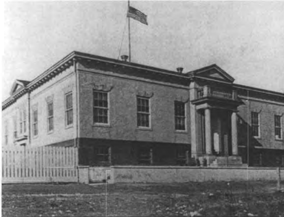
Jesse Reno School, photograph from the 1908 Report of the Schoolhouse Commission, Martin Luther King, Jr. Library, Washingtoniana Division, reproduced in Helm, Tenleytown, D.C., p. 138.
