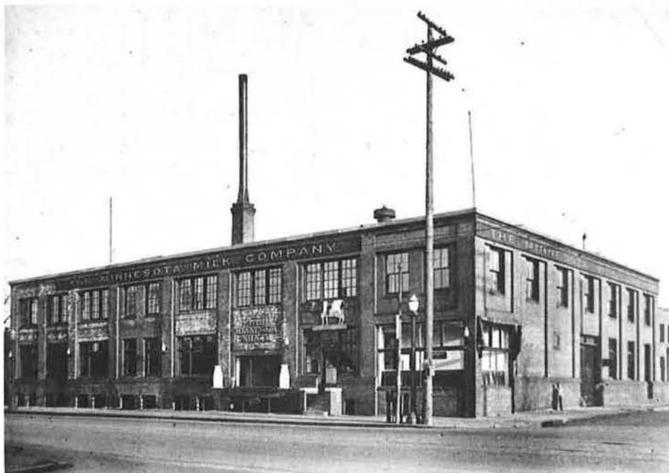
Figure 5: 1931 photograph of the Minnesota Milk Company building looking southeast.
