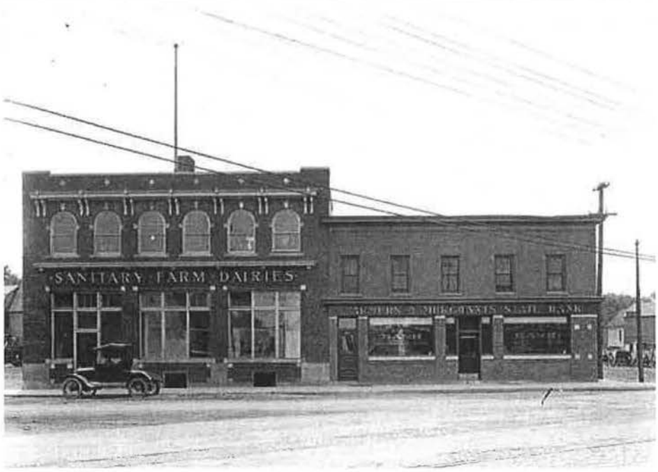
Figure 26: Early photograph of the Sanitary Farm Dairies plant shortly after it was constructed in 1915 at 880-888 E. Minnehaha Avenue.
