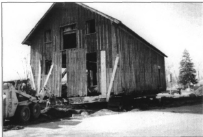
Figure 1. Lenoir Cotton Mill Warehouse shortly after renovation efforts began in 2004.
