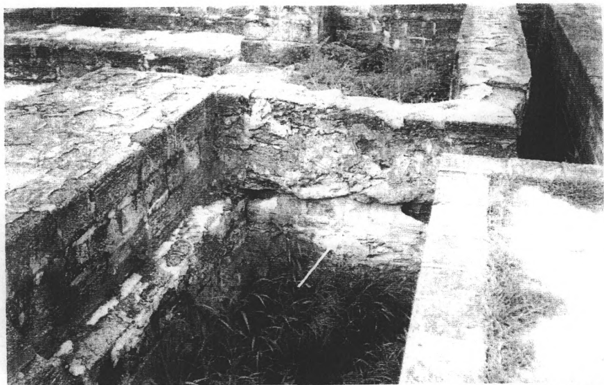
Figure 11. View of southern extension of the coquina ruins at Old Fort Park, facing east, showing different construction episodes. Note differences in materials from bottom (Hull) to top (WPA).
