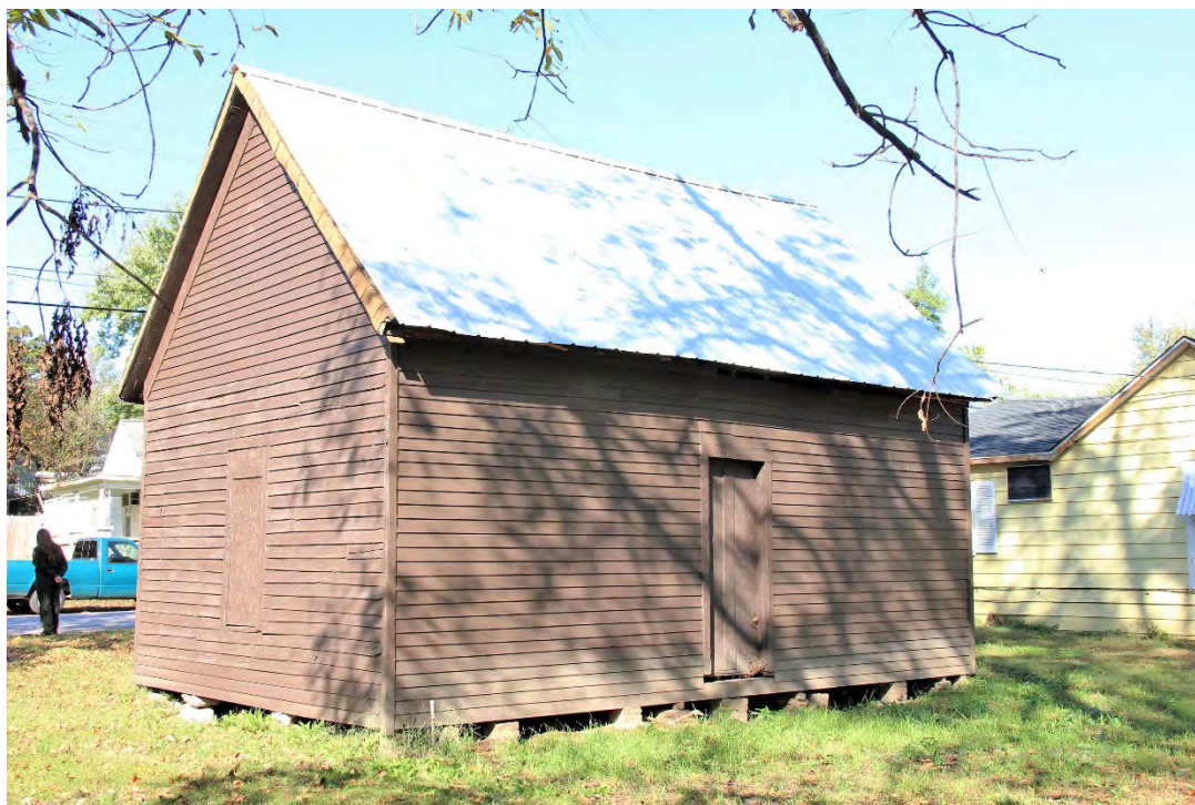
4 of 17: Southeast corner.
