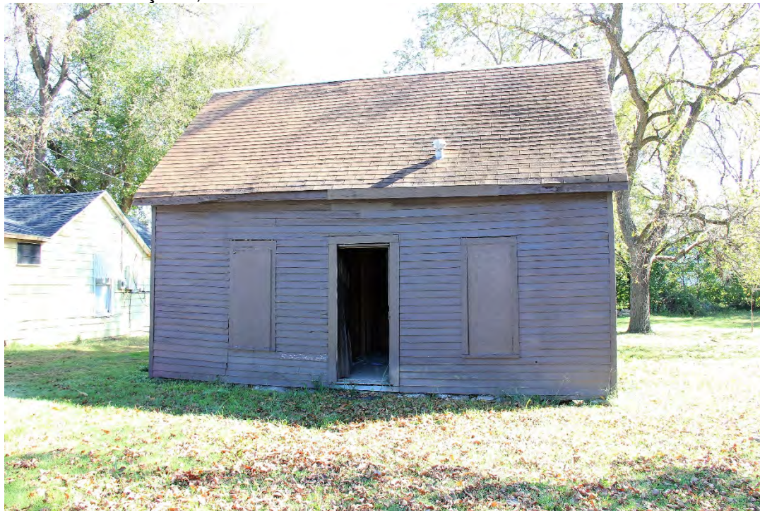
1 of 17: Façade, west wall.
