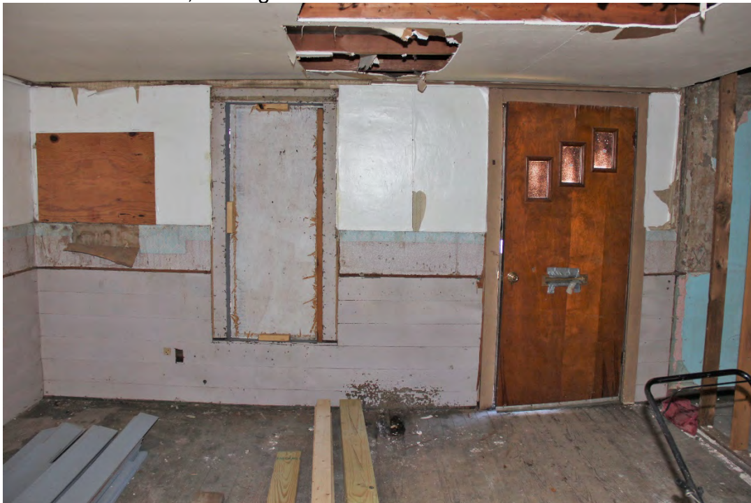
9 of 17: Room 101, looking west.
