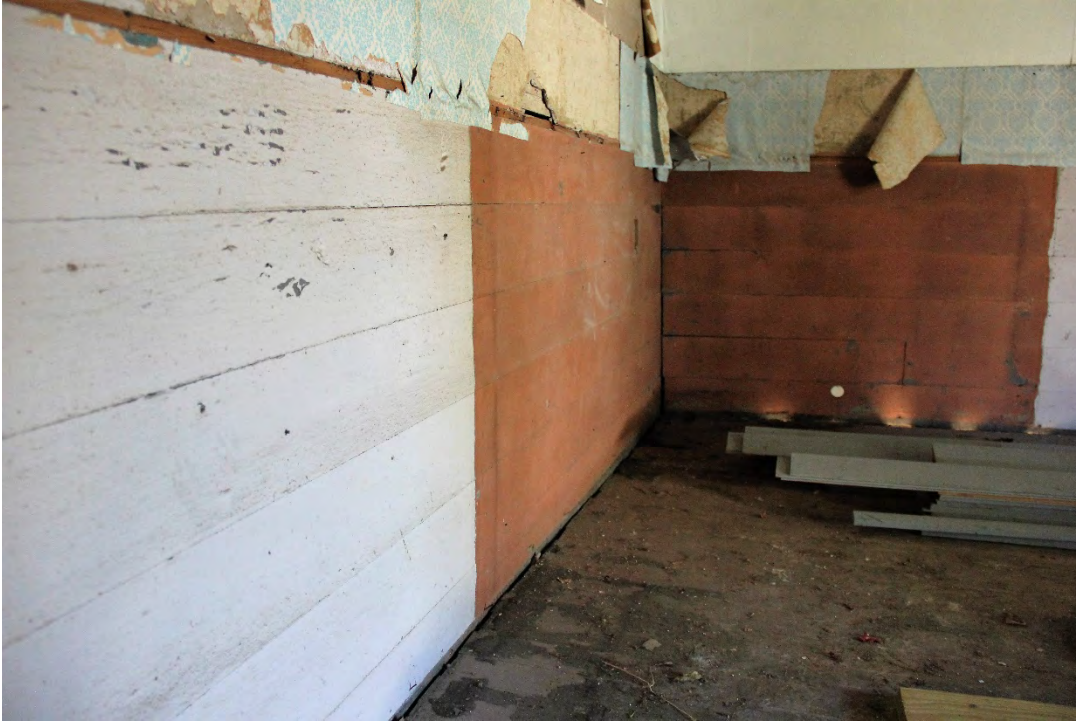
11 of 17: Room 101, east wall, looking south at wainscoting.
