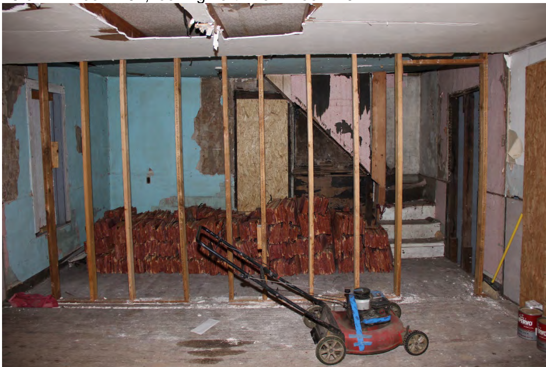
15 of 17: Room 102, looking north from Room 101.
