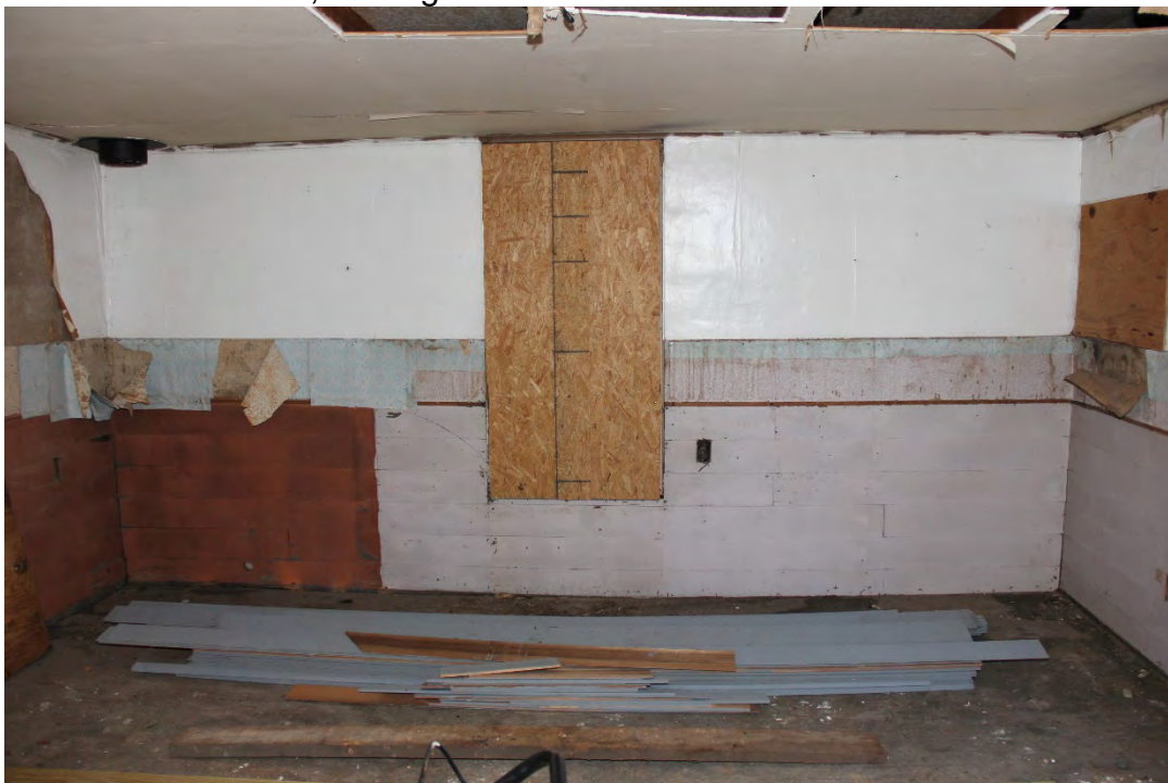
10 of 17: Room 101, looking south.
