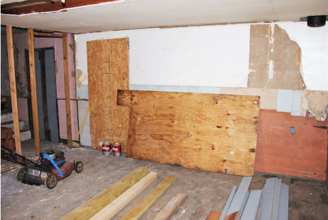
13 of 17: Room 101, looking east.
