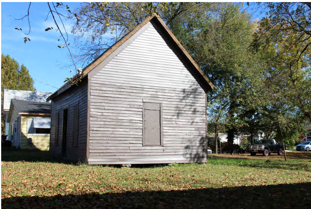
2 of 17: South side wall.
