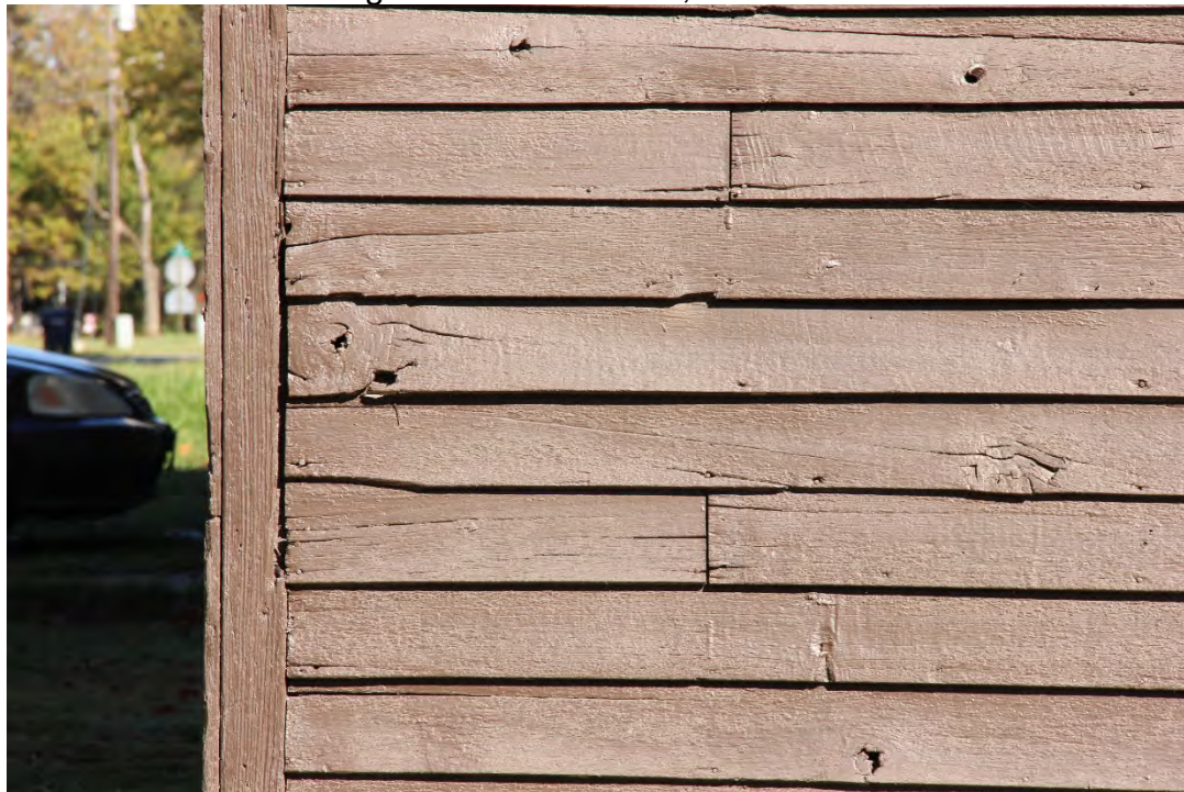
3 of 17: Detail of original weatherboards, south side wall
