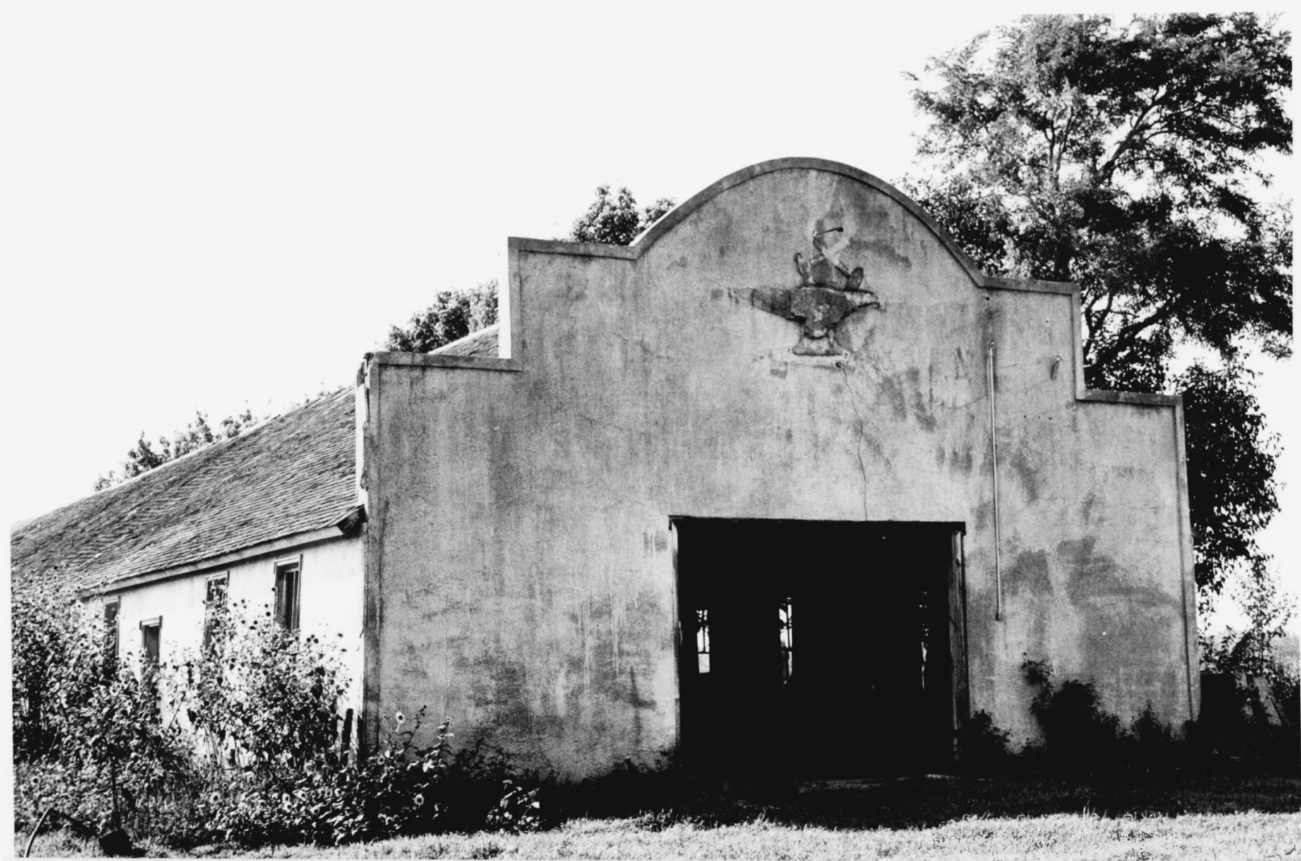
101 Ranch Historic District (Blacksmith Shop), Marland, Oklahoma Photo by Peavler and Associates for ABC and NPS, 1974
