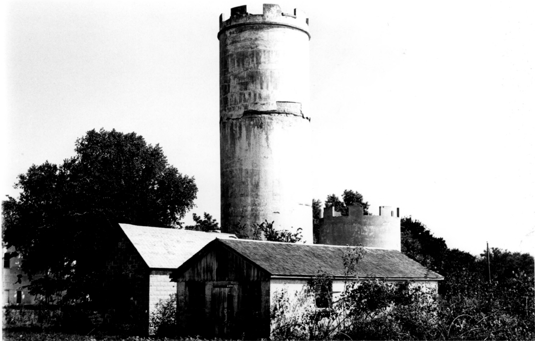
101 Ranch Historic District (Silos, Granery and Milk Storage), Marland, Oklahoma
