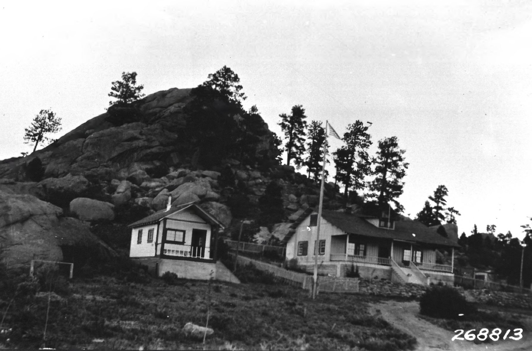
TRES PIEDRAS RANGER DISTRICT TAOS CO., NM PHOTO # 3
