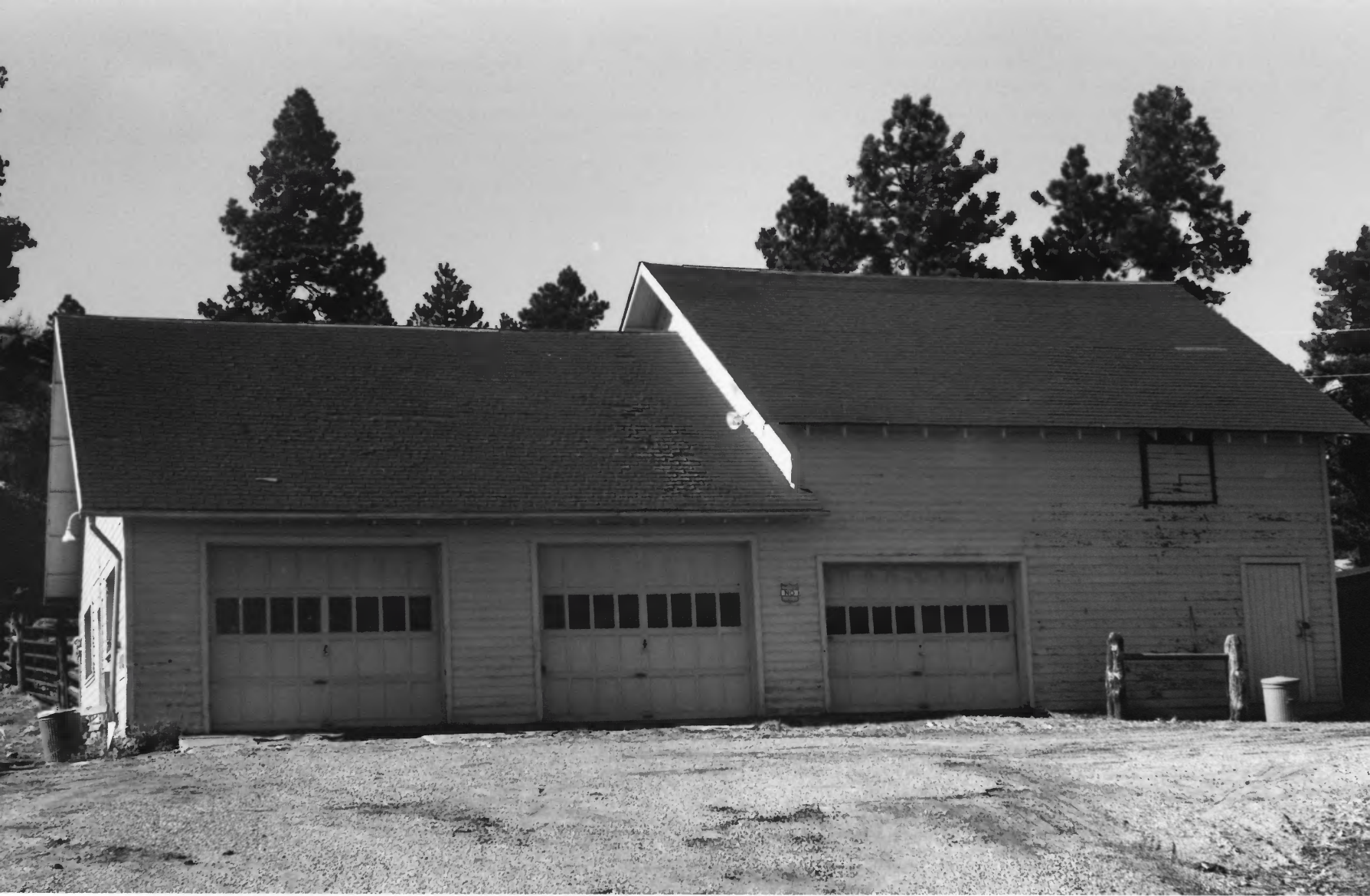
TRES PIEDRAS RANGER DISTRICT TAOS CO., NM PHOTO # 12
