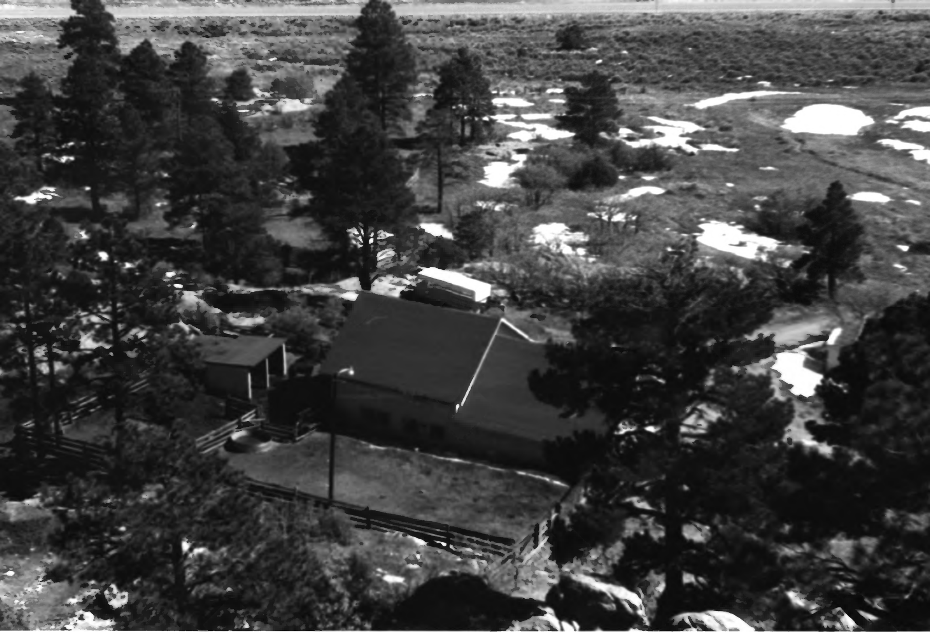
TRES PIEDRAS RANGER DISTRICT TAOS CO., NM PHOTO # 13
