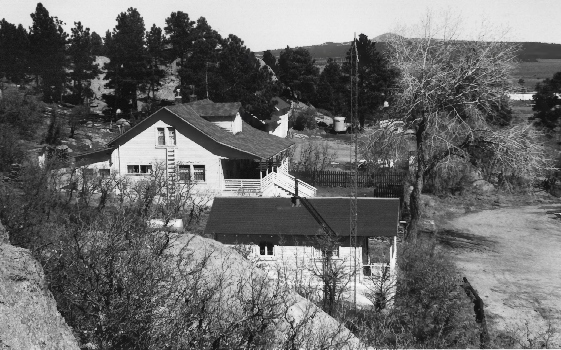
TRES PIEDRAS RANGER DISTRICT TAOS CO., NM PHOTO # 7
