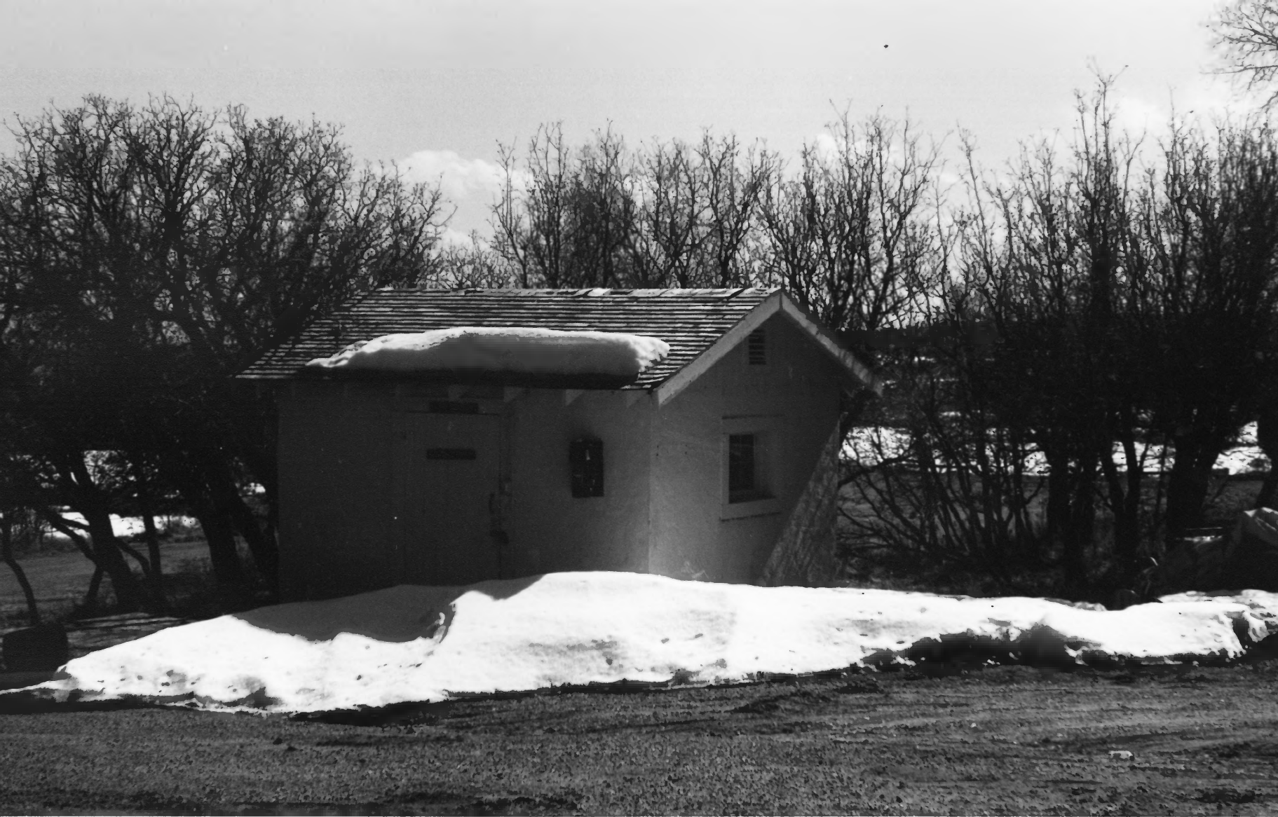
TRES PIEDRAS RANGER DISTRICT TAOS CO., NM PHOTO # 15
