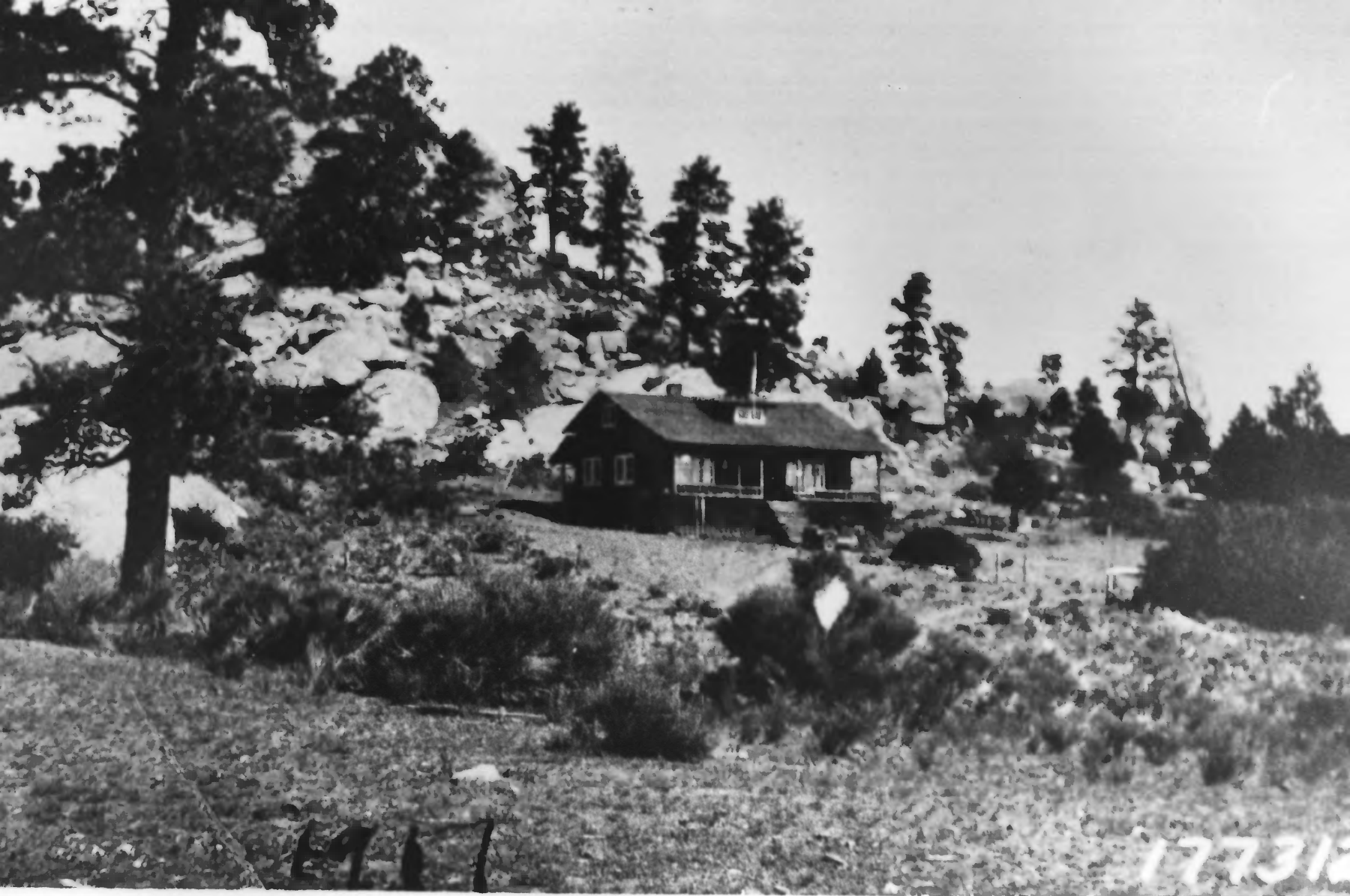
TRES PIEDRAS RANGER DISTRICT TAOS CO., NM PHOTO # 8
