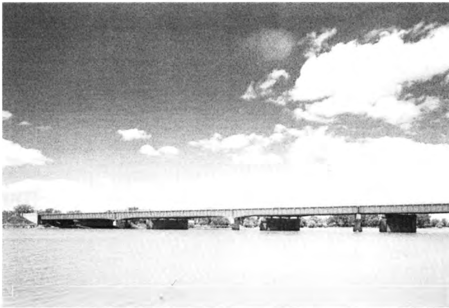
Photo 0002. O. S. Warden Bridge. South elevation. View to the northwest.
