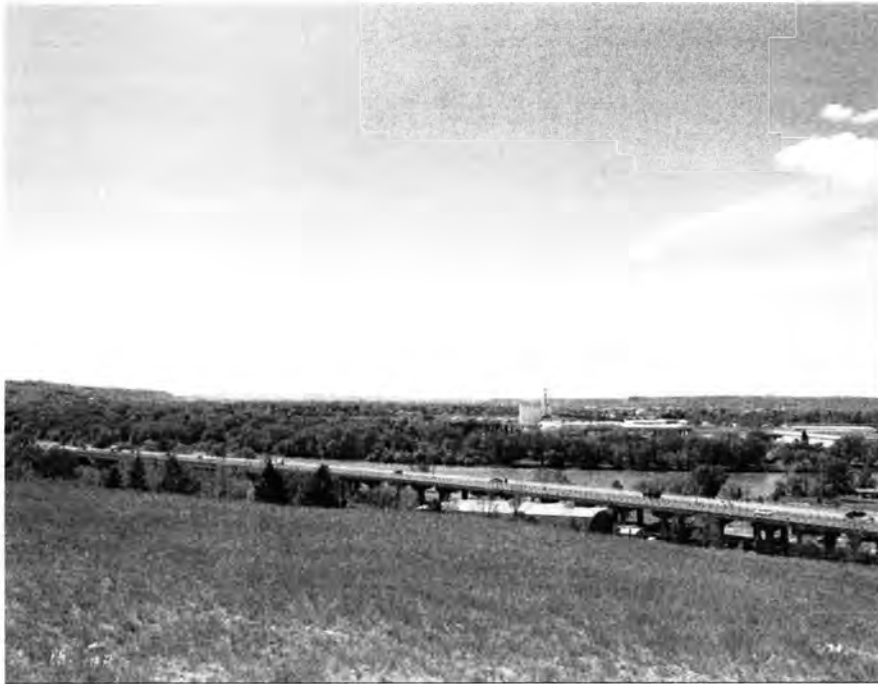
Photo 0001. O. S. Warden Bridge. South elevation. View to the northwest.
