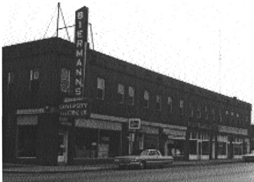
Photo 3: The brick stringcourse, vents, and decorative brick recesses on the second story above the windows are prominent in this 1968 photograph, part of an appraisal report for the Biermann Electric Co. (2300 University Avenue L.L.C.)
