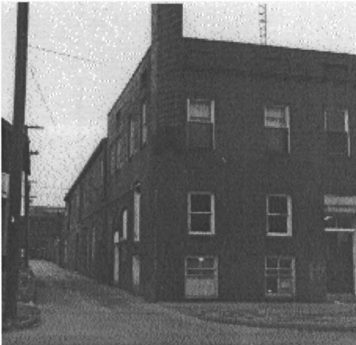
Photo 4: Windows on the first story had not been bricked up yet when this photograph of the west and rear sides of the building was taken in 1968 as part of an appraisal report for the Biermann Electric Co. The brick on the first story of the building appears to be a different shade than that used on the second story. Note the remnant of the decorative stringcourse at the base of the chimney. (2300 University Avenue L.L.C.)
