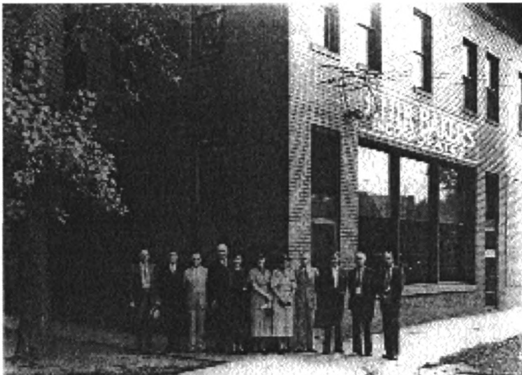
Photo 2: This circa-1936 photograph shows how the corner facade looked before it was remodeled. The sign painted on the building reads "Better Bakers Incorporated," the name of the business that rented the dairy's former front office for about a year, according to city directory listings. Better Bakers was listed as being located at 2300 University Avenue in the 1936 city directory. (William Biermann)
