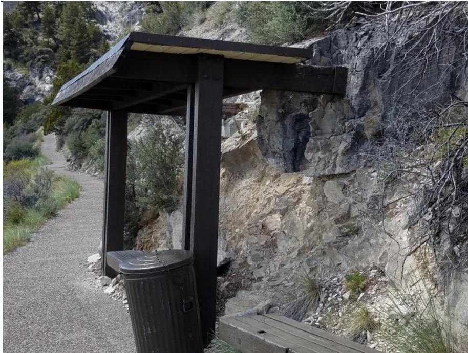
MT_JeffersonCounty_Lewis&ClarkCavernsHD_0005: Above: Stopping bench along Upper Trail, view to west.
