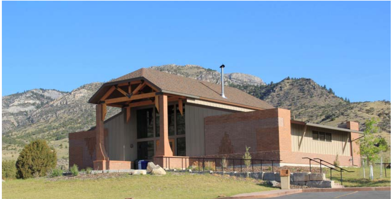
MT_JeffersonCounty_Lewis&ClarkCavernsHD_0041: 2010 Visitor Center, looking northwest. Photo courtesy C. Van West. (Outside of NR Boundary).
