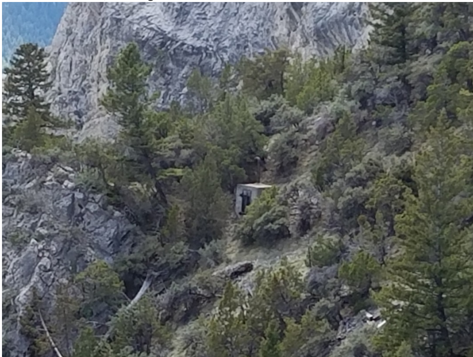
MT_JeffersonCounty_Lewis&ClarkCavernsHD_0032: Below: Feature 5, Tram Operations Building below caverns entrance, looking southwest.
