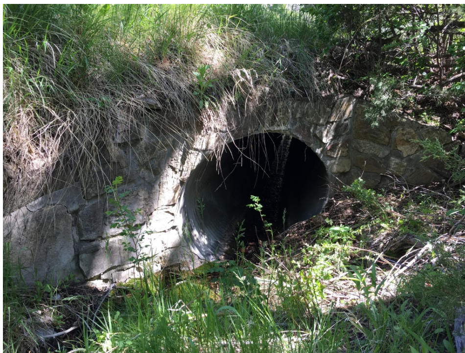
MT_JeffersonCounty_Lewis&ClarkCavernsHD_0024: Feature 12, Lower Culvert, looking east.
