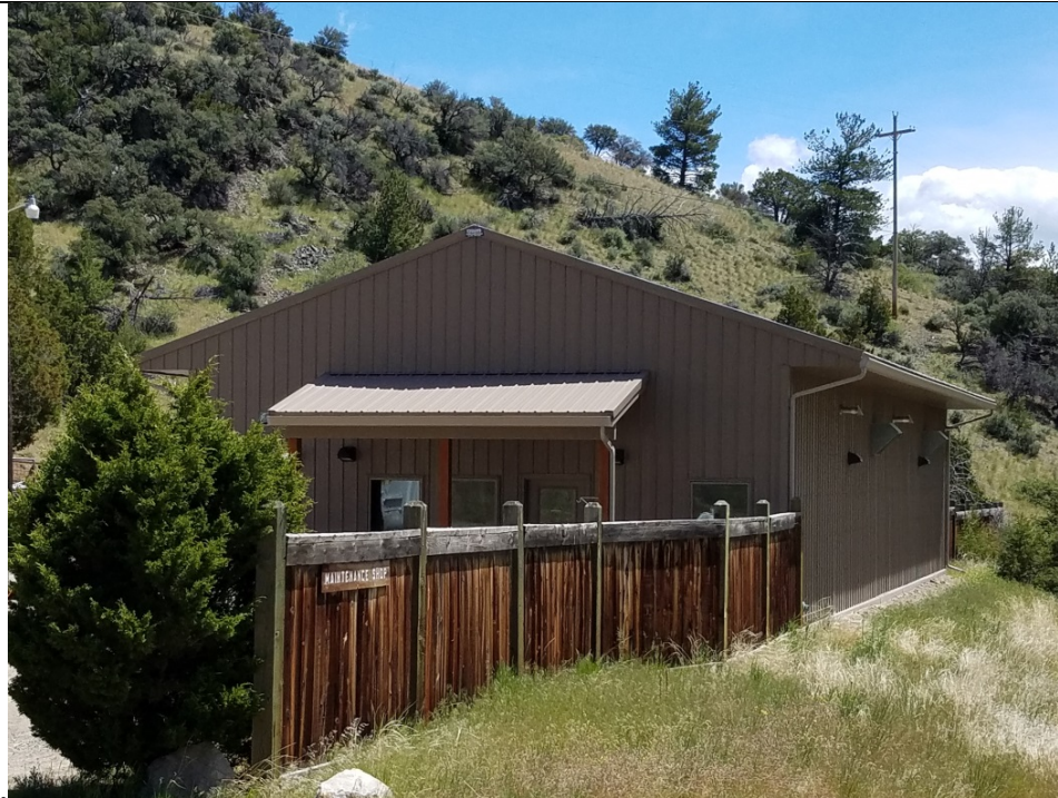
MT_JeffersonCounty_Lewis&ClarkCavernsHD_0037: Above Feature 16 Maintenance Shop, looking southeast.
