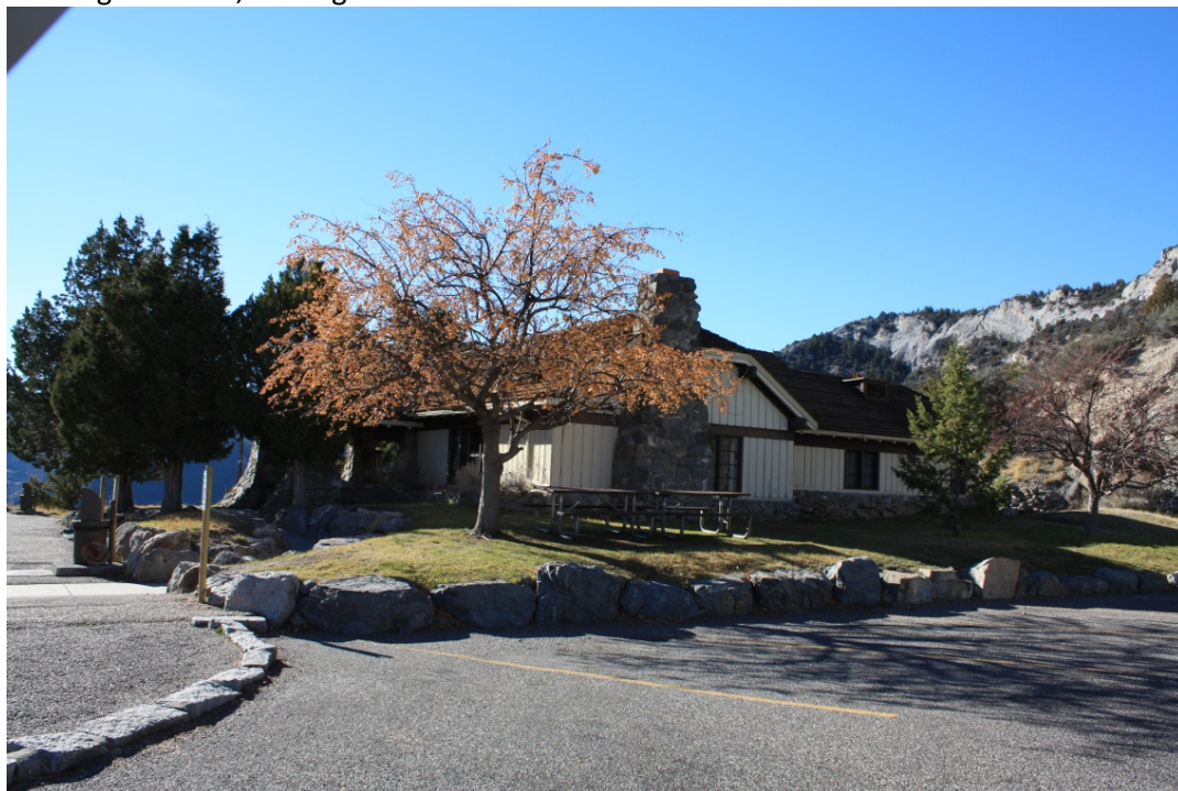
MT_JeffersonCounty_Lewis&ClarkCavernsHD_0010: Feature 6, Lewis and Clark Caverns Headquarters Building Entrance, looking west.
