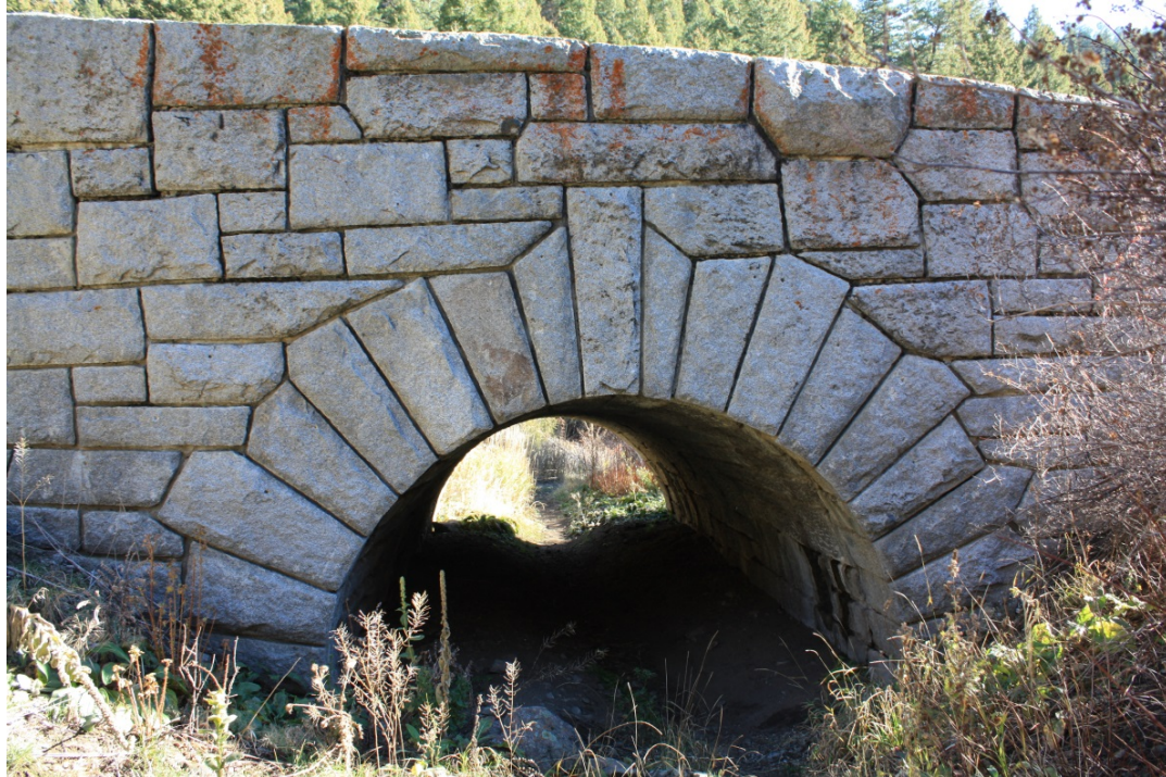
MT_JeffersonCounty_Lewis&ClarkCavernsHD_0030: Above: Feature 9, Granite Arch Bridge, detail looking to the east.
