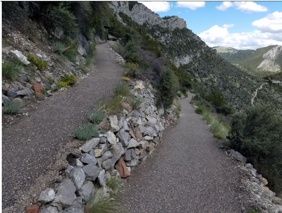
MT_JeffersonCounty_Lewis&ClarkCavernsHD_0007: Below: Feature 3, switchback in upper trail as it approaches caverns, looking northeast.
