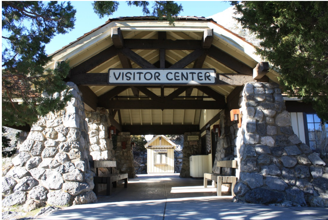
MT_JeffersonCounty_Lewis&ClarkCavernsHD_0009: Feature 6, Lewis and Clark Caverns Headquarters Building Entrance, looking northwest.
