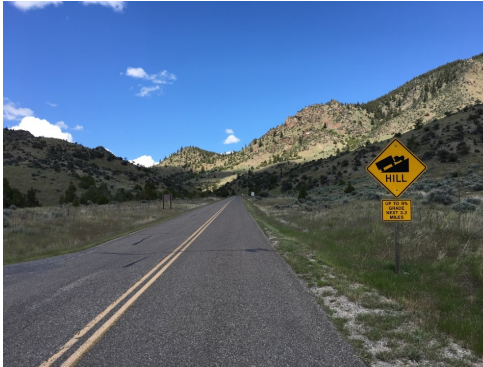
MT_JeffersonCounty_Lewis&ClarkCavernsHD_0033: Above: Feature 15, Beginning of CCC Roadway, looking north up Greer Gulch.
