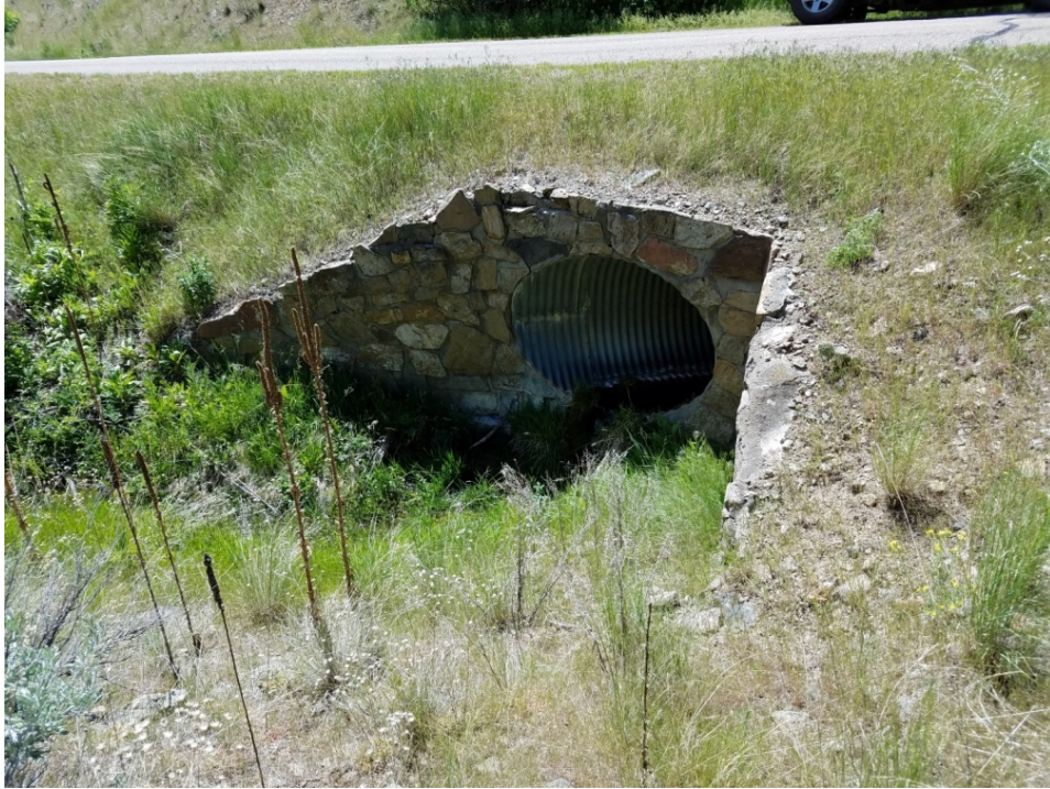
MT_JeffersonCounty_Lewis&ClarkCavernsHD_0025: Feature 12, Lower Culvert, looking west.
