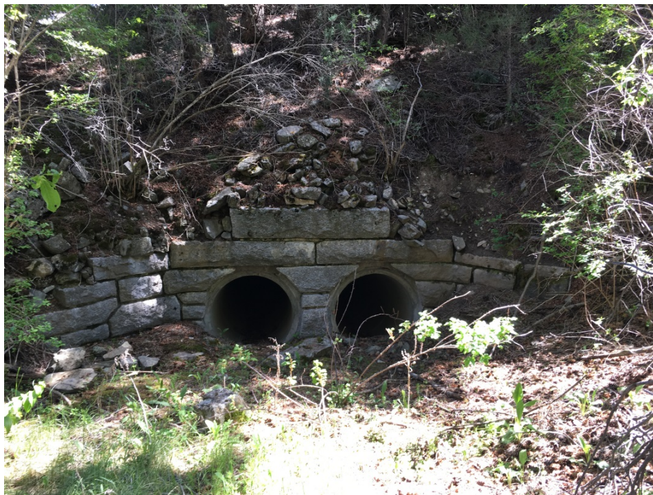
MT_JeffersonCounty_Lewis&ClarkCavernsHD_0021: Feature 10, Culvert, looking west.
