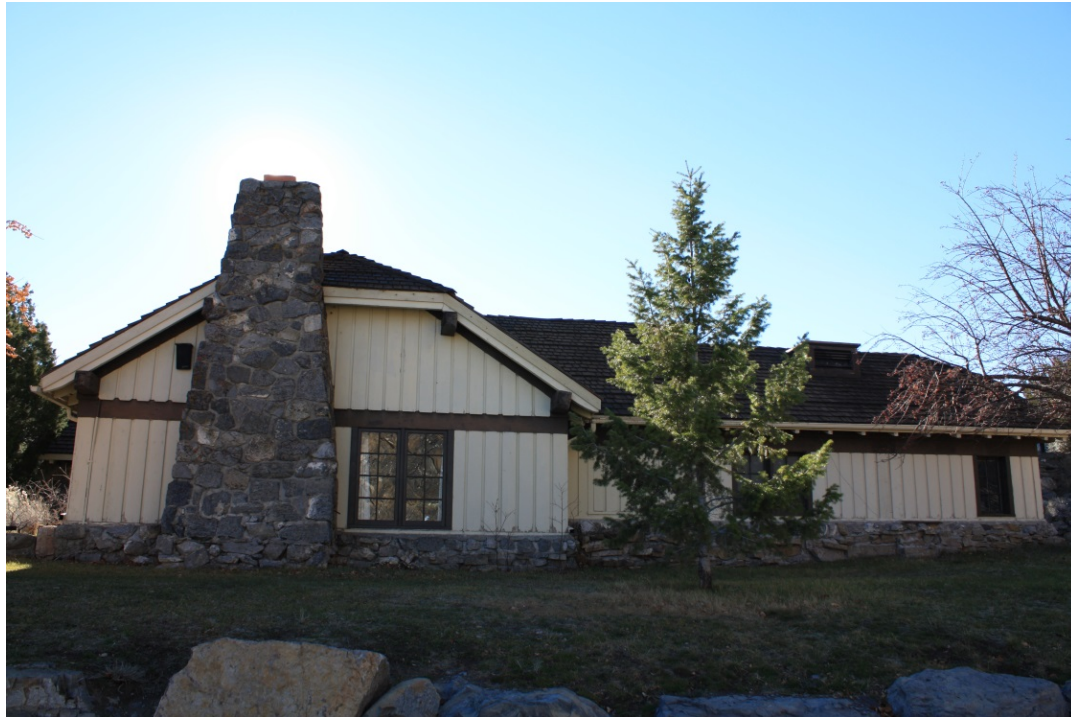
MT_JeffersonCounty_Lewis&ClarkCavernsHD_0011: Feature 6, Lewis and Clark Caverns Headquarters Building, looking southeast.
