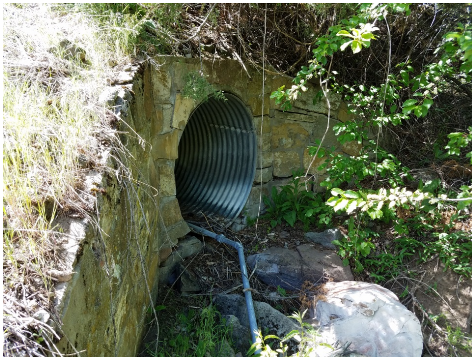
MT_JeffersonCounty_Lewis&ClarkCavernsHD_0023: Feature 11 Culvert, looking southeast.
