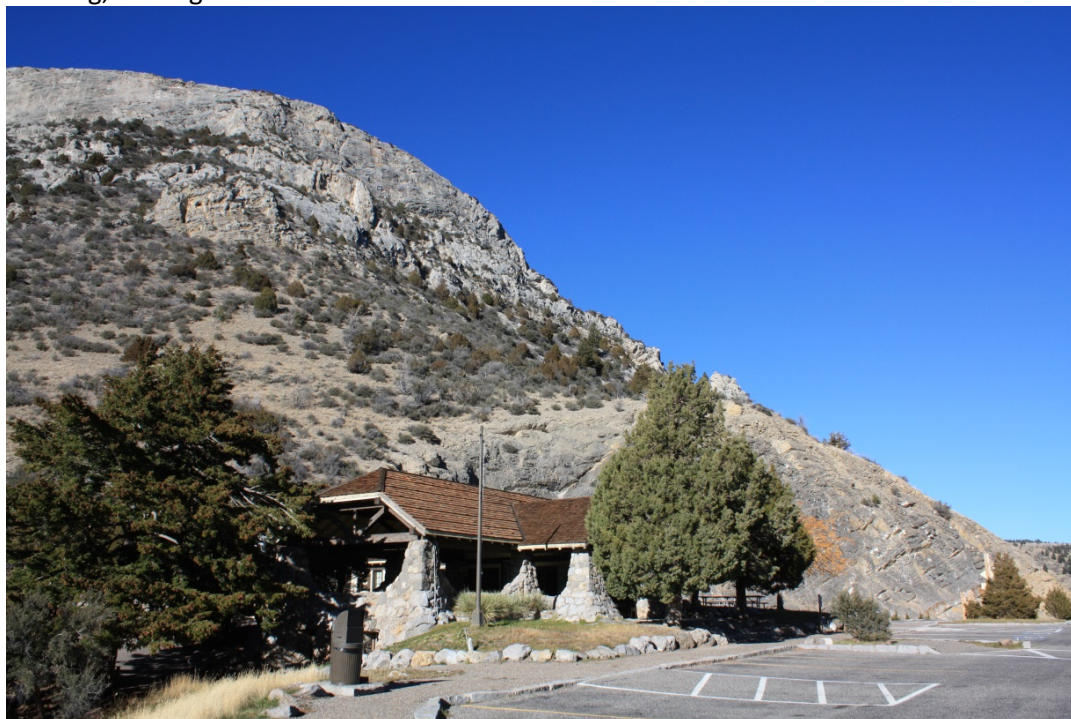
MT_JeffersonCounty_Lewis&ClarkCavernsHD_0012: Feature 6: Lewis and Clark Caverns Headquarters Building, looking east.
