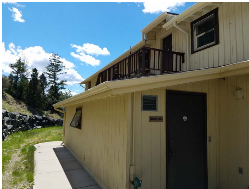
MT_JeffersonCounty_Lewis&ClarkCavernsHD_0019: Feature 7, Concessions Building, rear elevation looking to the southwest.
