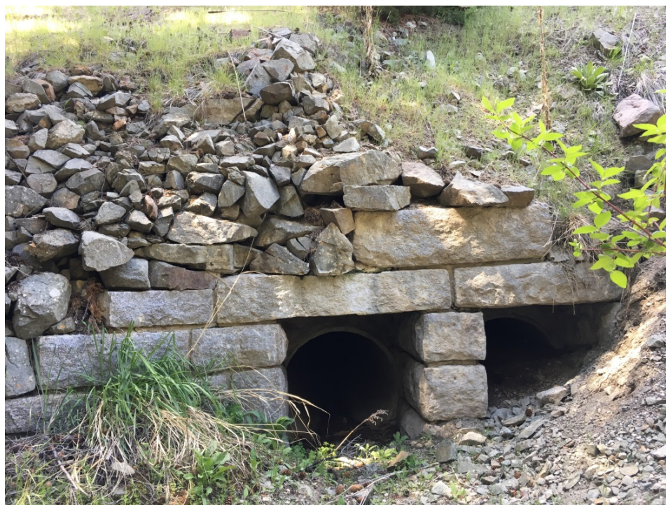
MT_JeffersonCounty_Lewis&ClarkCavernsHD_0020: Feature 10, Culvert, looking east.
