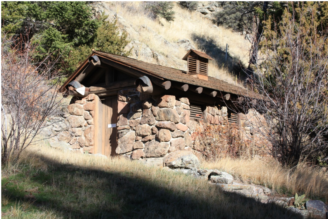
MT_JeffersonCounty_Lewis&ClarkCavernsHD_0036: Below: Feature 8, Latrine in Picnic Area, looking northeast.
