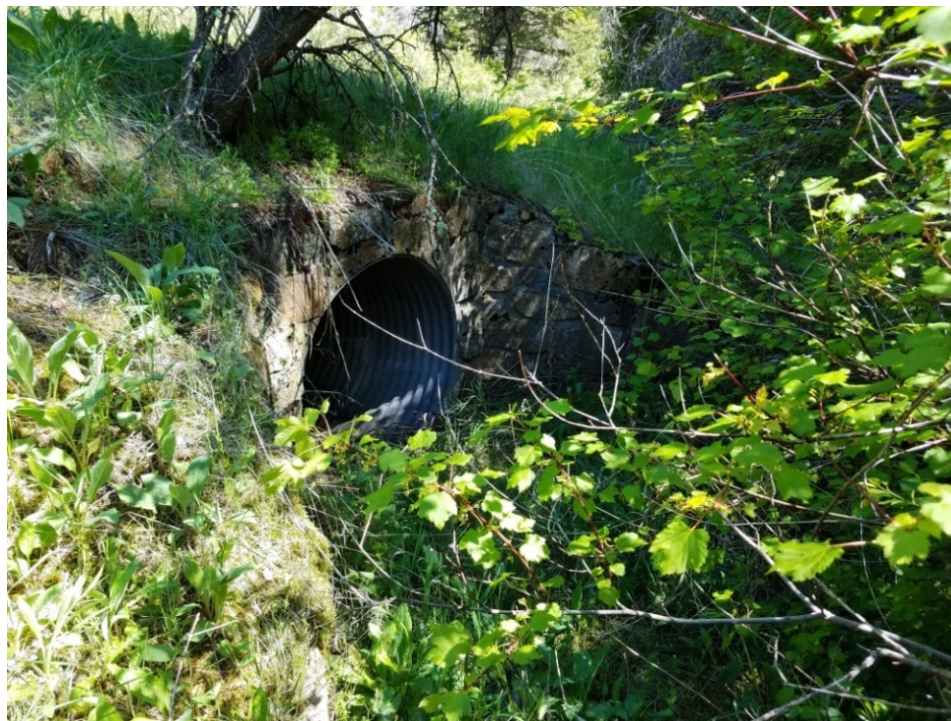
MT_JeffersonCounty_Lewis&ClarkCavernsHD_0022: Feature 11 Culvert, looking northwest.
