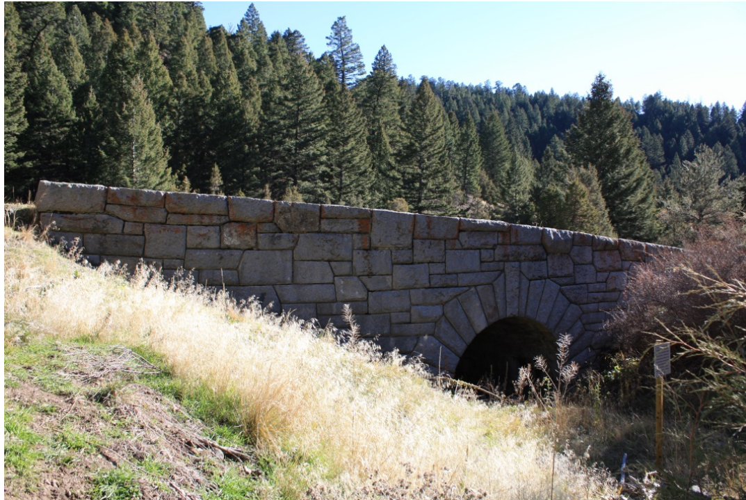
MT_JeffersonCounty_Lewis&ClarkCavernsHD_0029: Above: Feature 9, Granite Arch Bridge, looking to the east.
