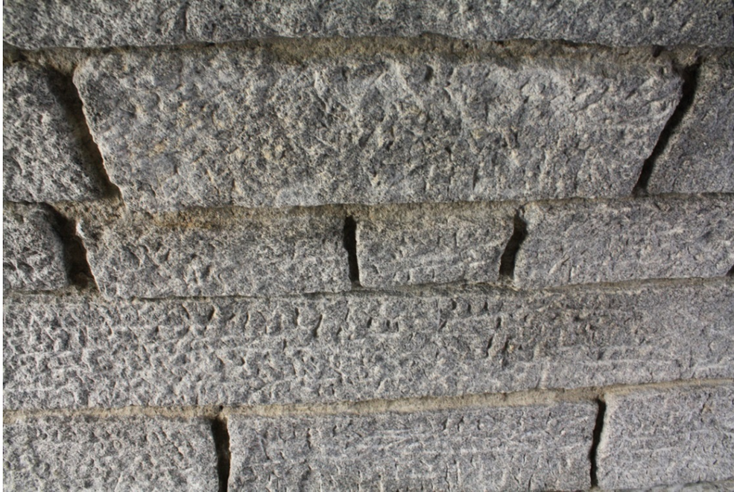
MT_JeffersonCounty_Lewis&ClarkCavernsHD_0031: Above: Feature 9, Stonework inside Granite Bridge barrel vault.
