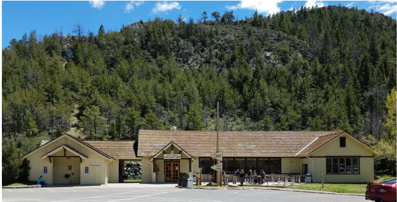
MT_JeffersonCounty_Lewis&ClarkCavernsHD_0015: Feature 7, Concessions Building, looking to the southeast.
