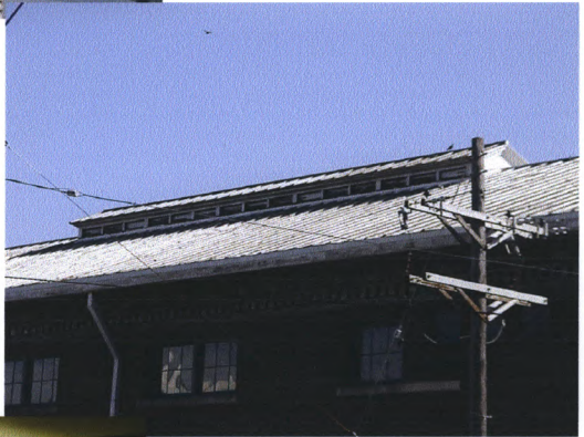
Nisqually Power Substation, Pierce County, WA Detail: Wooden Louvered Roof Vent, Looking East 09/00, M.Sullivan, Photo
