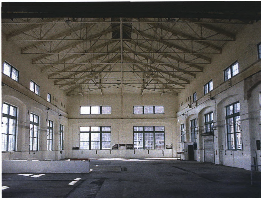
Nisqually Power Substation, ▲ Pierce County, WA Interior View, Main Floor, Looking South 09/00, M. Sullivan, Photo
