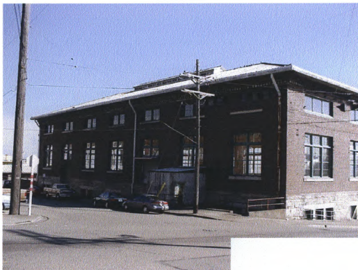
Nisqually Power Substation, Pierce County, WA West Elevation, Looking East 09/00, M.Sullivan, Photo
