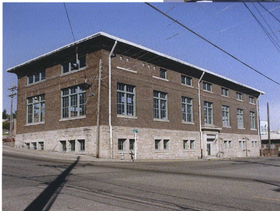
Nisqually Power Substation, Pierce County, WA East and South Elevations, Angle Looking Northwest 09/00, M.Sullivan, Photo
