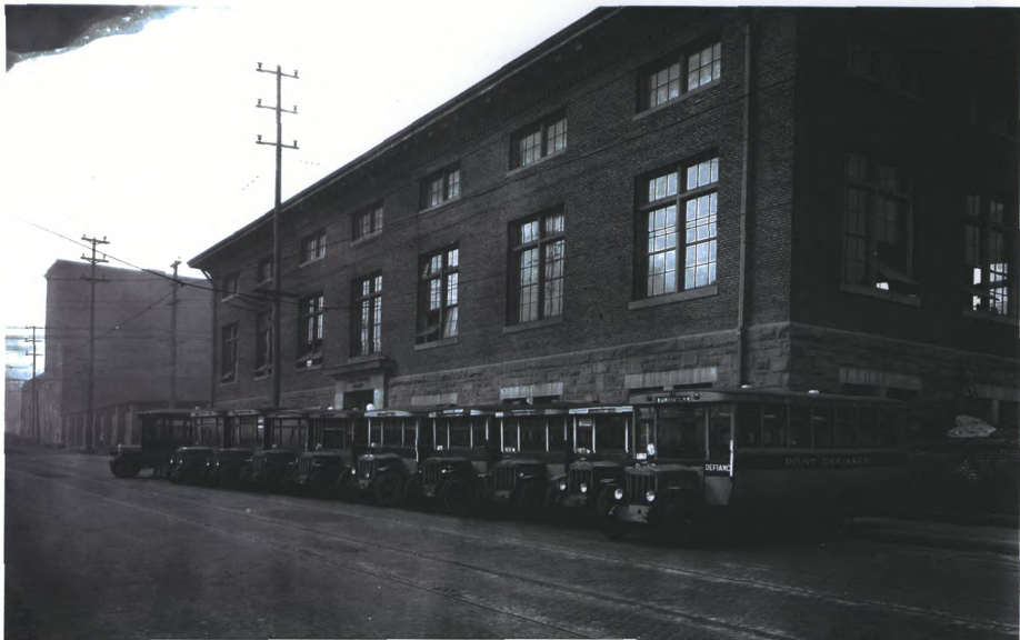
National Register of Historic Preservation Nomination Form – Section 12 NISQUALLY POWER SUBSTATION, 2416 S. C Street, Tacoma, Pierce Co., WA Historic Photograph, c. 1912, Photographer: Boland Original Negative Located at the Washington State Historical Society View: Main Building, View of East and North Exterior Elevations from Corner of 24 th C Streets
