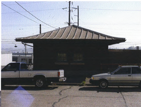
Nisqually Power Substation, Pierce County, WA Detail: Storehouse, West Elevation, Looking East 09/00, J.Lovejoy, Photo
