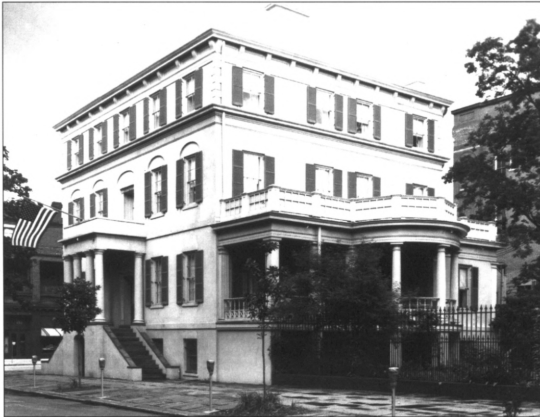
Juliette Gordon Low Birthplace, south elevation, southeast corner. Photo courtesy of Juliette Gordon Low Girl Scout National Center, 1980.
