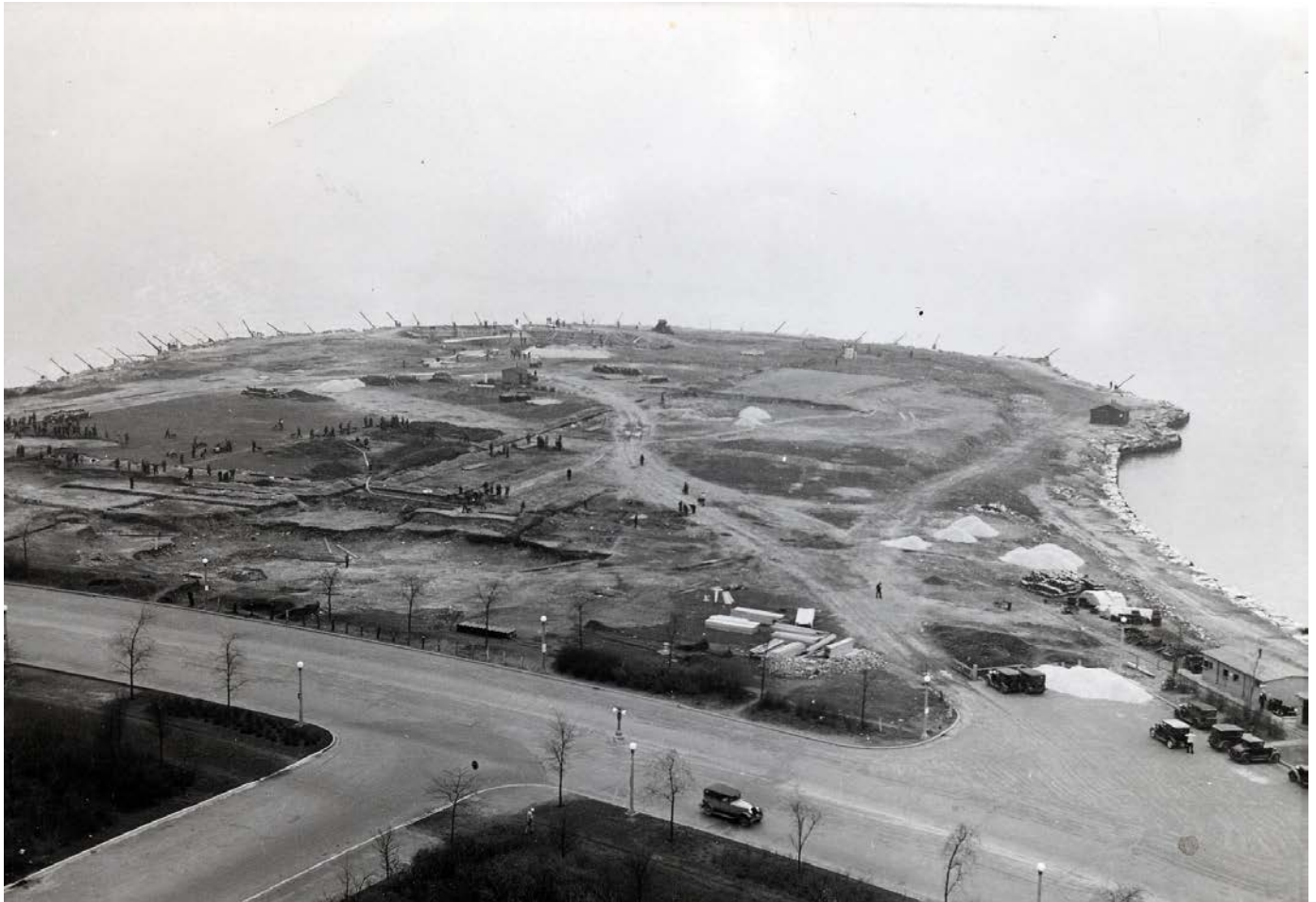
Figure 4. Aerial view of Promontory Point showing underway to complete revetments and grading, 1936, Chicago Park District Records: Photographs, Chicago Public Library Special Collections
