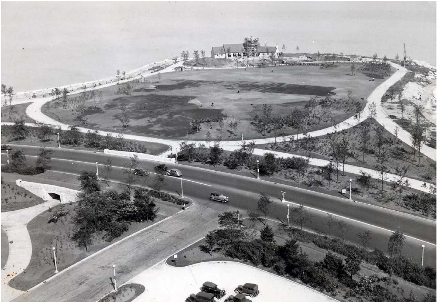
Figure 5. Promontory Point landscape and pavilion construction, 1937, Chicago Park District Records: Photographs, Chicago Public Library Special Collections.
