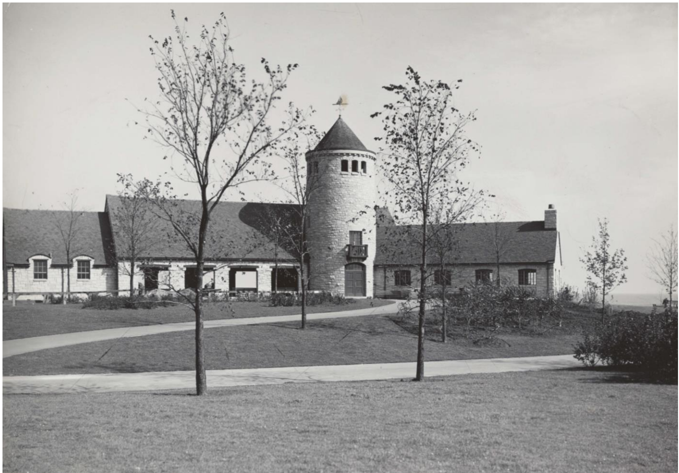
Figure 9. Promontory Point Pavilion, ca. 1940, Chicago Park District Records: Photographs, Chicago Public Library Special Collections.
