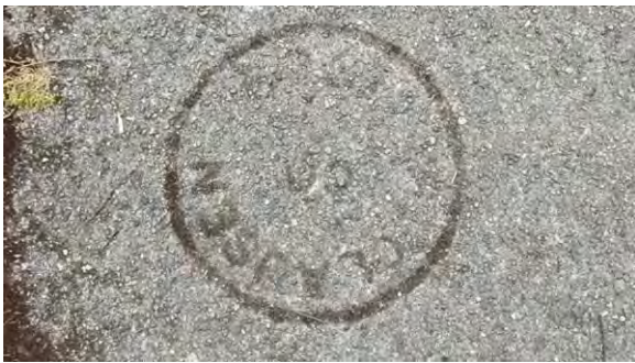
Examples of Contractor stamp cast into sidewalks
