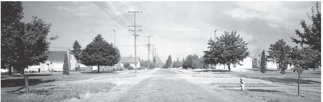
1941 Aug18 - N. 21 st Street & Union Avenue, view east district on right, Tacoma Public Utilities Collection
