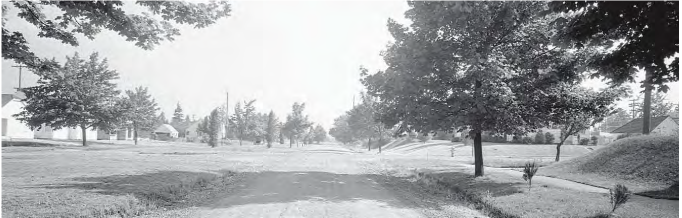
1941 Aug18 - N 21st Street & Union Avenue, view south district on left, Tacoma Public Utilities Collection
