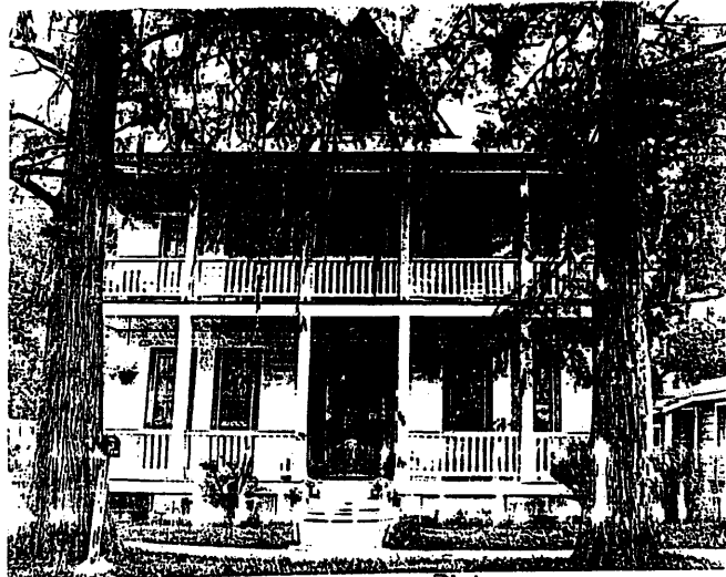
Pre 1915 Restoration Photo
