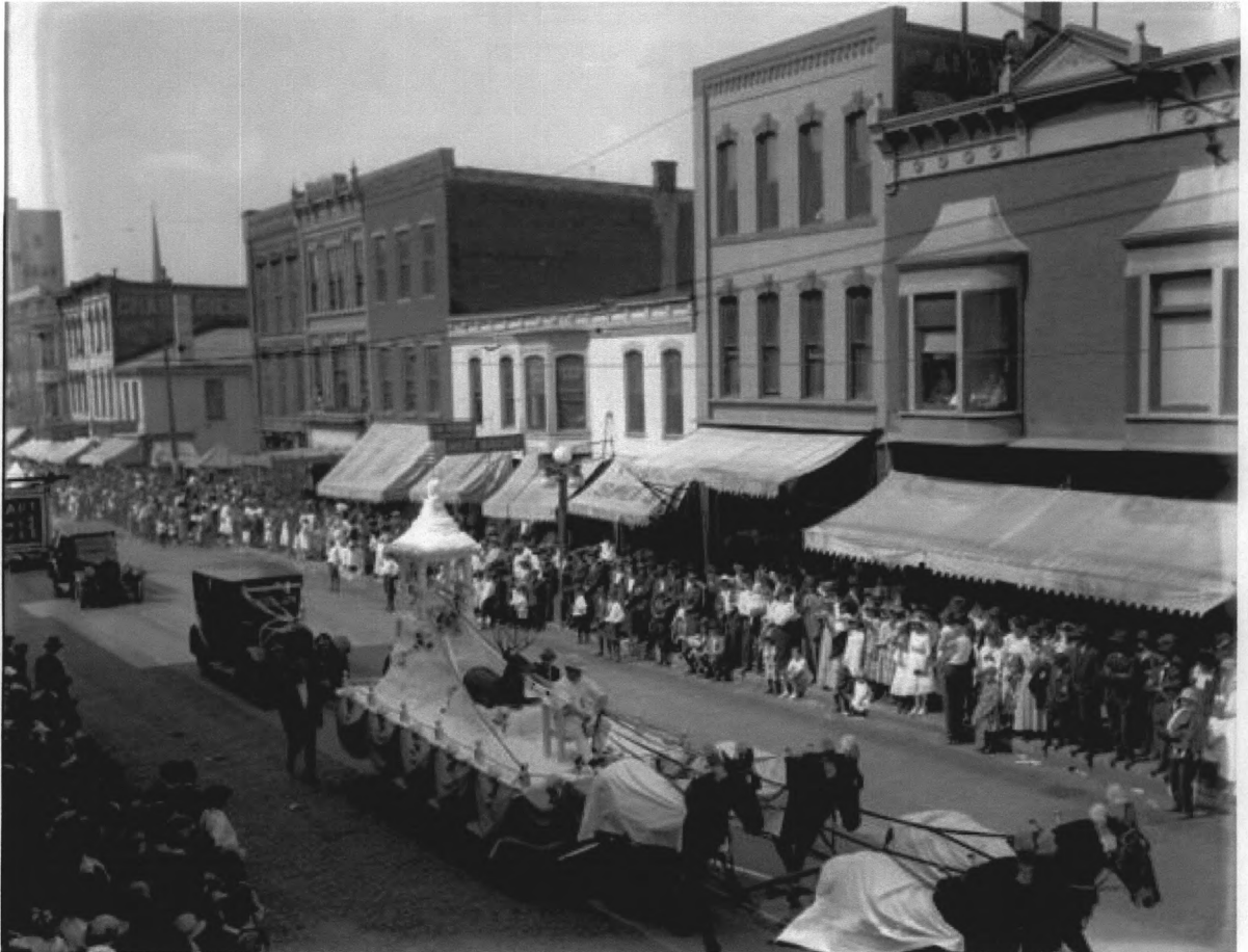
Figure 15. View of the 300 block of E. 2 nd Street in 1920, looking west from the middle of the block at the north side.
