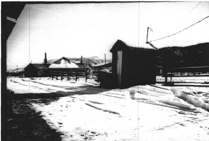
Shed #2, north and west elevations, view to southeast. Clubhouse is on left in background. Photo by Allan Mathews, December 2004.
