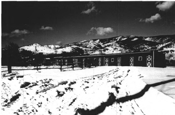
Barn #7, south and east elevations, view to northwest. Photo by Allan Mathews, December 2004.
