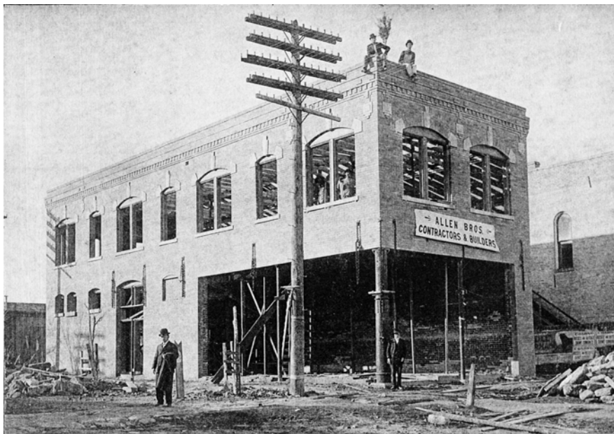
Wheeler Building (101 W. South Main, #33) under construction in 1907. Image courtesy of E.A. Arnim Archives & Museum, Flatonia, TX.
