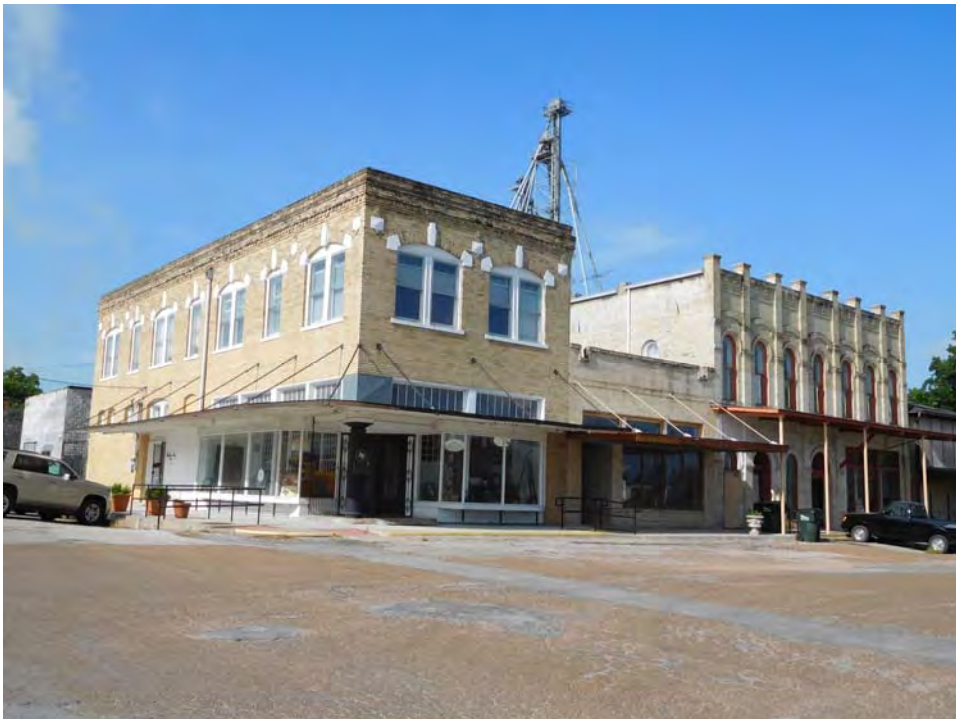
Photo 34 101-109 W. South Main
