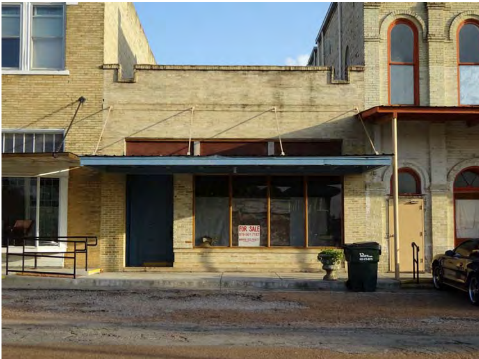
Photo 10 105 W. South Main St
