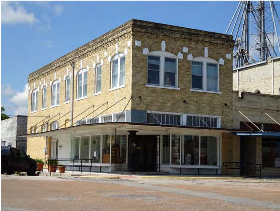
Photo 9 101 W. South Main St
